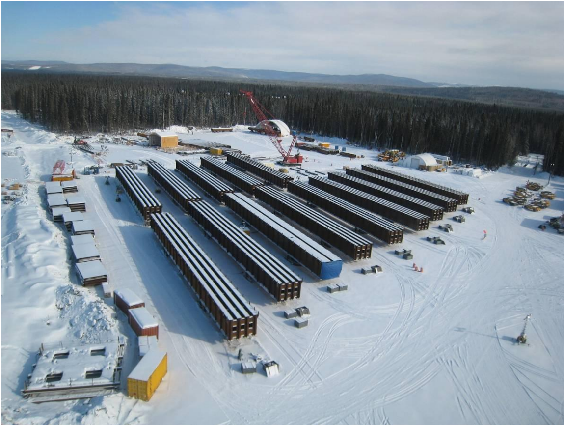
Figure 3. Northern Rail Extension Beams. Photographed March 2013.
