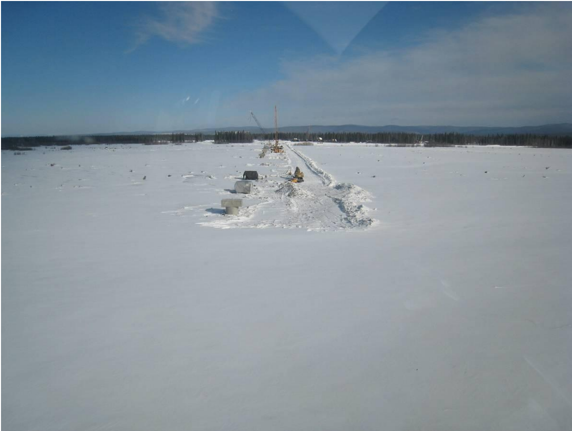
Figure 1. Northern Rail Extension Winter Progress. Photographed March 2013.
