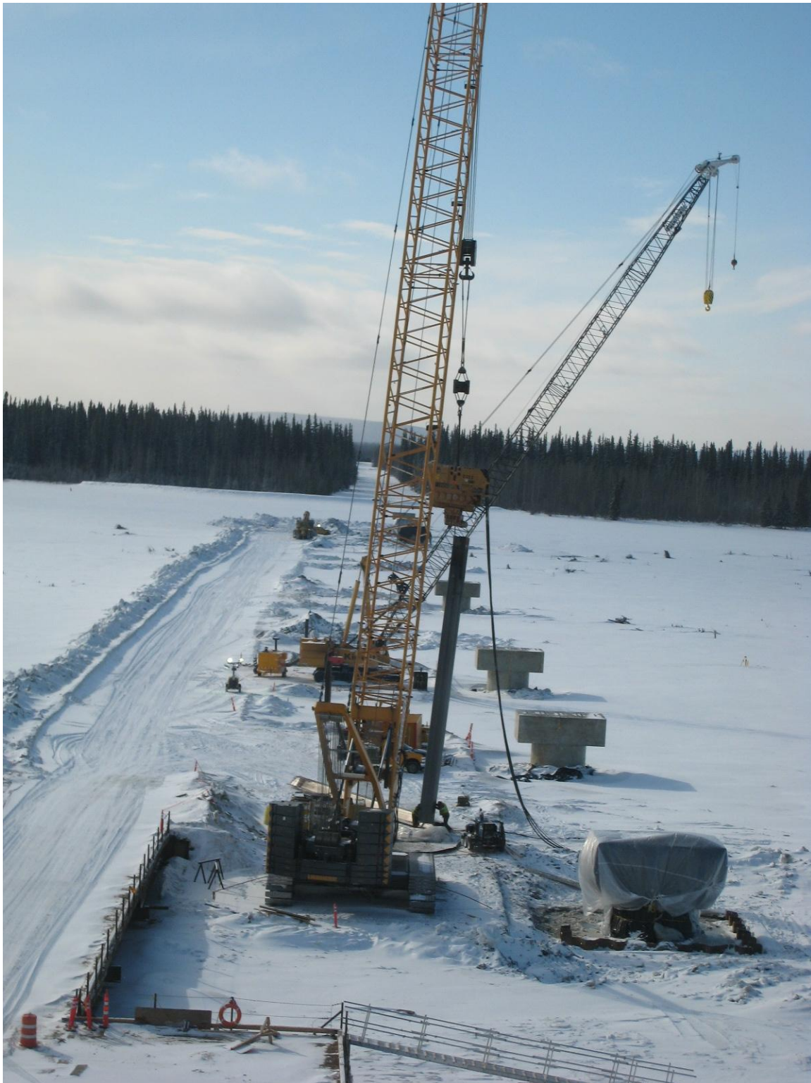
Figure 2. Northern Rail Extension Alignment, looking south. Photographed March 2013.
