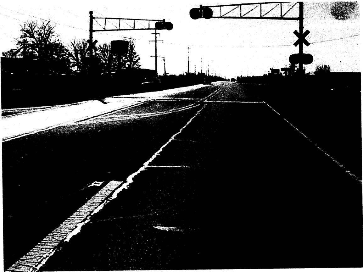
Allen Road and PPHW Crossing – Looking South
