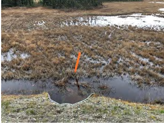
Photo 7. Cross Drainage at Large Wetland Area
