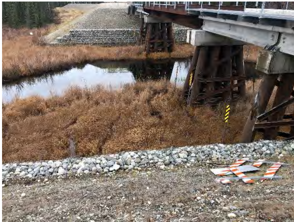
Photo 2. Clear Drainage Way, Gabion Walls are in Good Condition.
