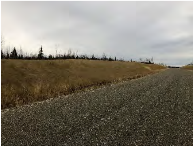
Photo 1. Stable Side Slope Vegetation.
