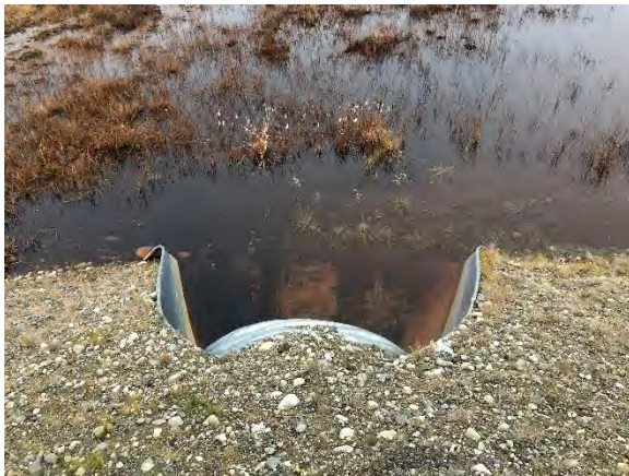
Photo 8. Culvert Apron, No Indication of Settlement or Erosion
