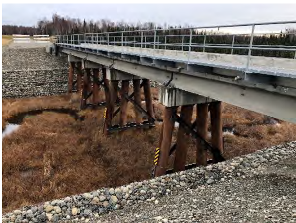
Photo 3. Unobstructed Drainage at Bridge Crossing.
