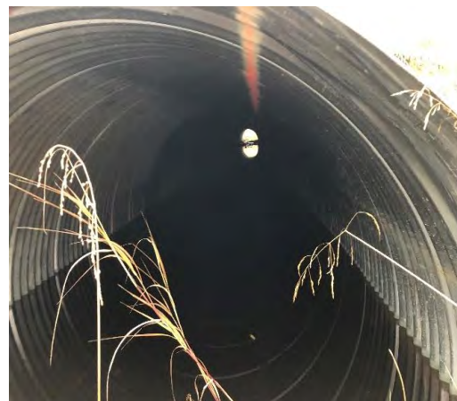
Photo 6. Culvert Showing no Signs of Debris Accumulation or Flow Issues.
