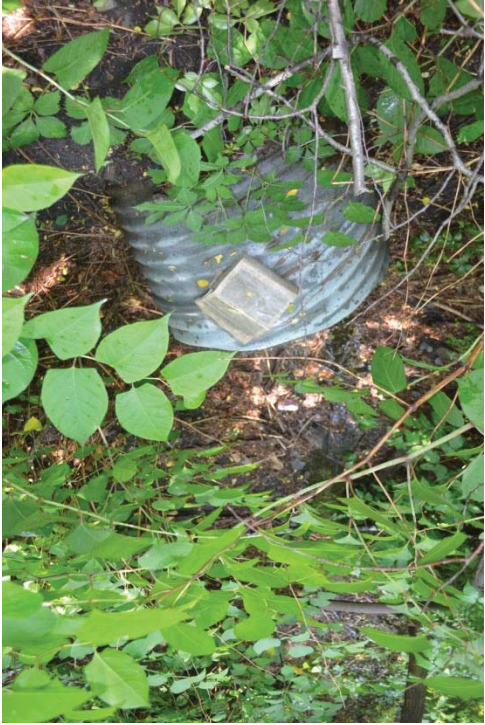
Culvert visible on south side of Harsimus Branch
