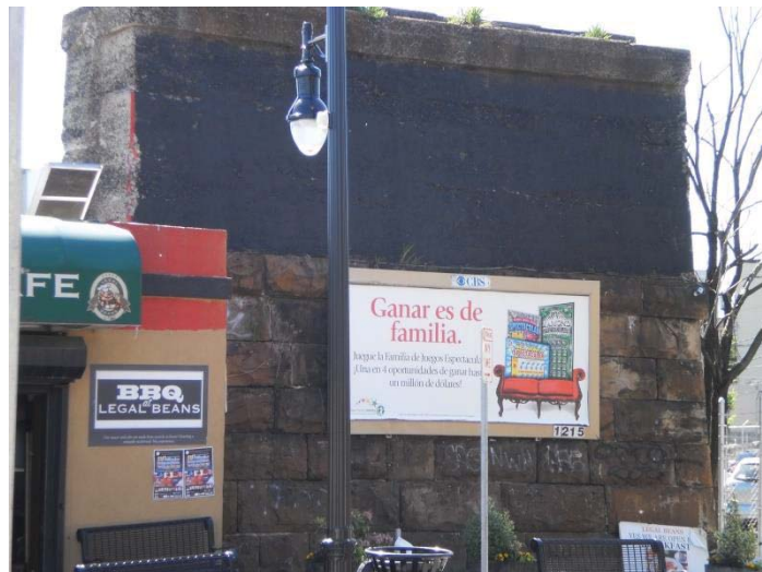
Photo taken 2013. Pier extant as of June 18, 2017.
