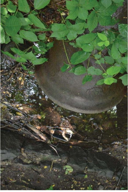
Iron culvert on north side of Harsimus Branch
