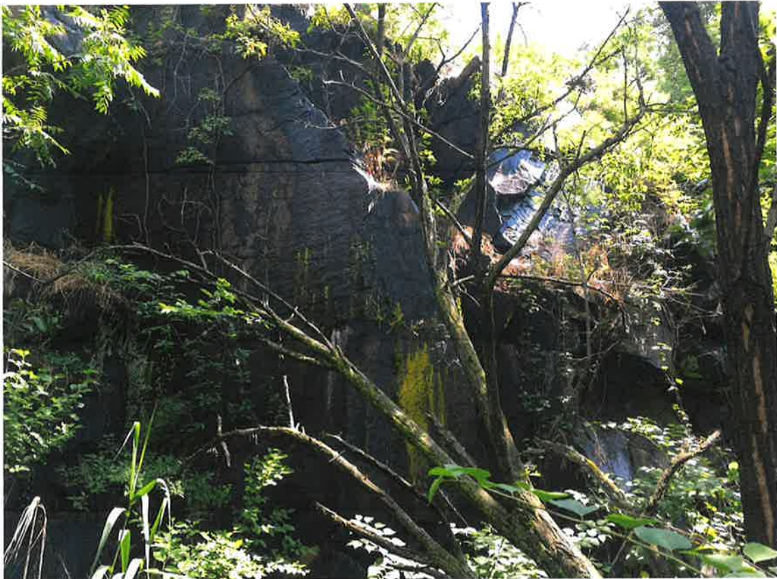
Photo 9. This stone wall was excavated to accommodate the Harsimus Branch and remains a monument to the engineering of this line.
