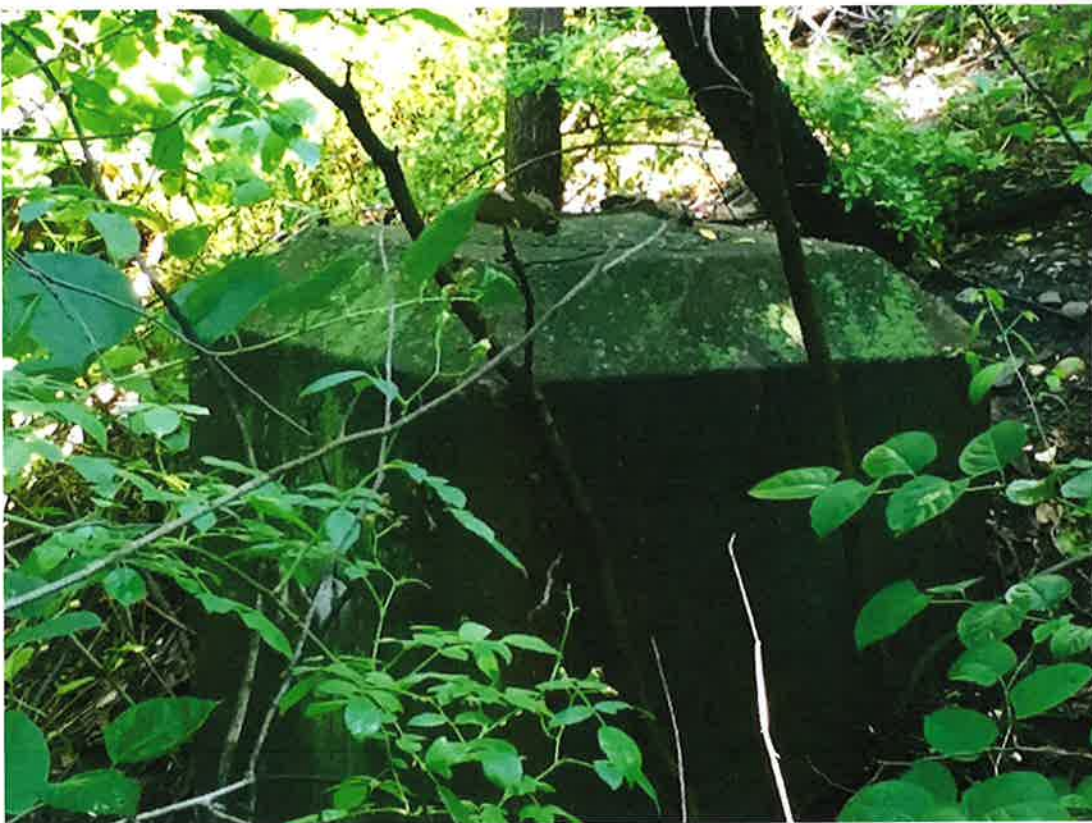
Photo 3. The second set of catenary foundation blocks. This one is on the north side.
