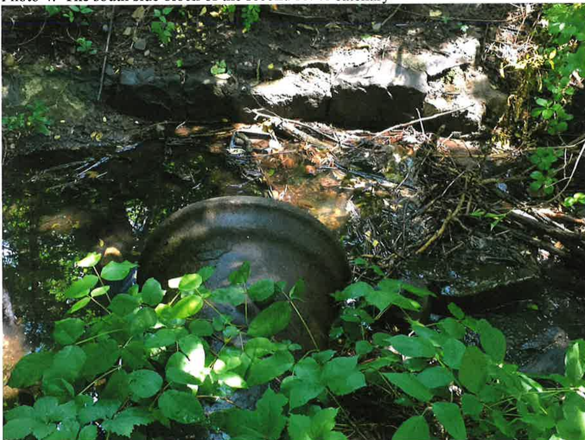
Photo 4. Culvert on the north side of the rail bed with man made stone banks. Looking north.
