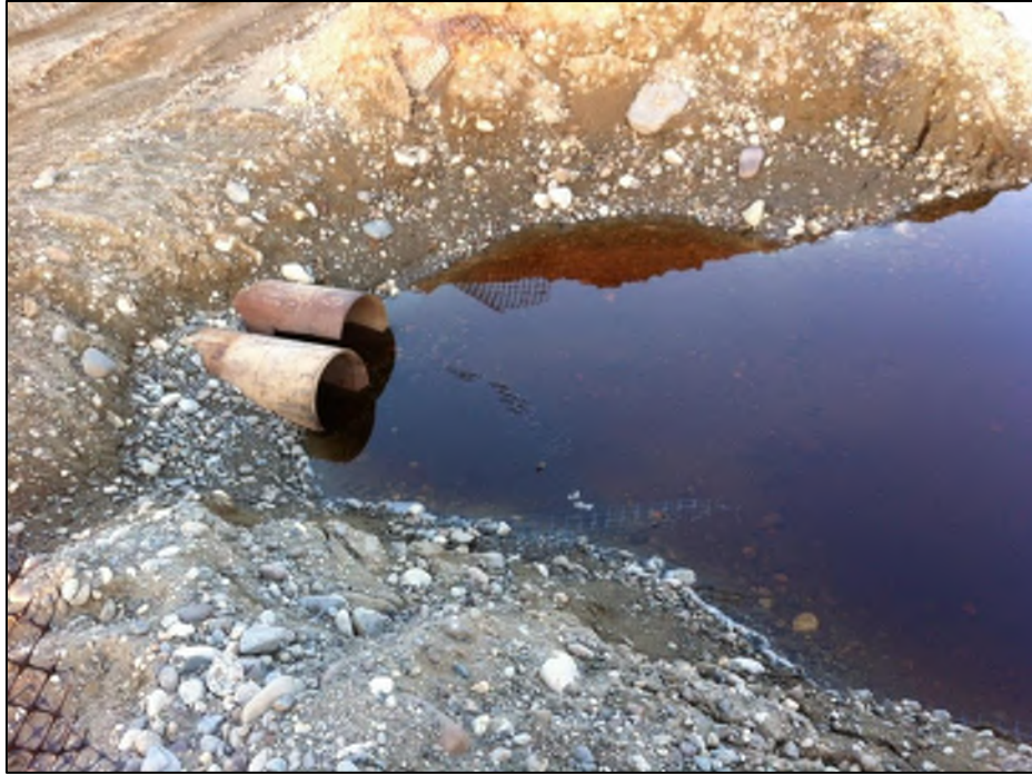
Figure 11: Inlet on project left to move impounded water with two 12" pipes. May 2, 2014. Notice the level of the impounded water has dropped significantly since April 22, 2014.
