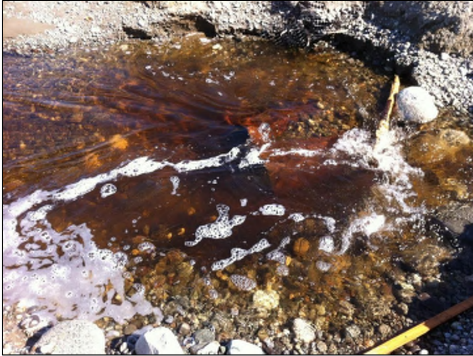
Figure 3: Impounded water from project left at STA4602+25 over the inlet: two 16" pipes. April 22, 2014.
