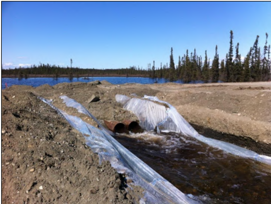
Figure 4: Outlet from the two 16" pipes into a Visqueen-lined channel into the wetlands on project right. April 22, 2014.
