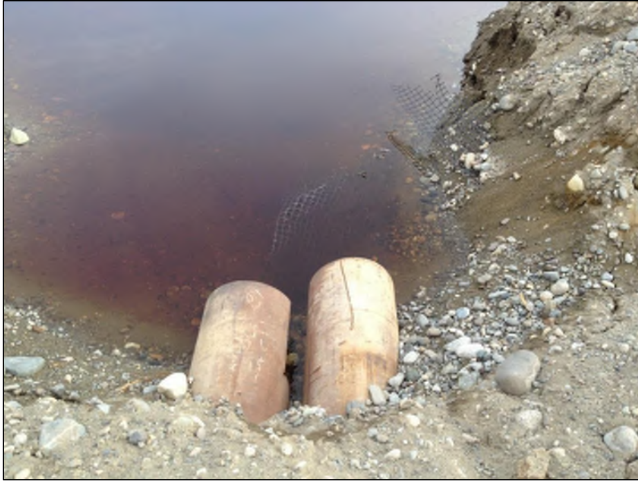
Figure 13: Inlet on project left to move impounded water with two 12" pipes. May 5, 2014. Notice the level of the impounded water has dropped significantly since April 22, 2014.
