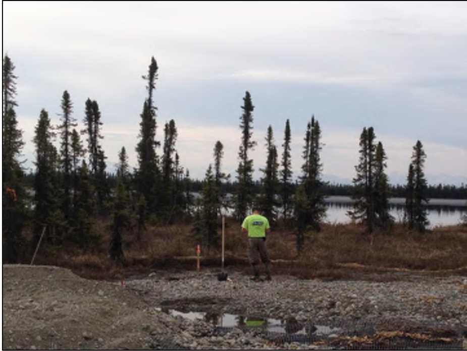
Figure 15: Laborer with metal rake and shovel removing fill from wetlands on project right. May 5, 2014.
