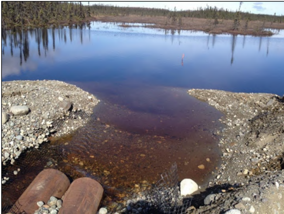
Figure 10: Inlet on project left to move impounded water with two 16" pipes. April 29, 2014. Notice the level of the impounded water has dropped significantly since April 22, 2014.
