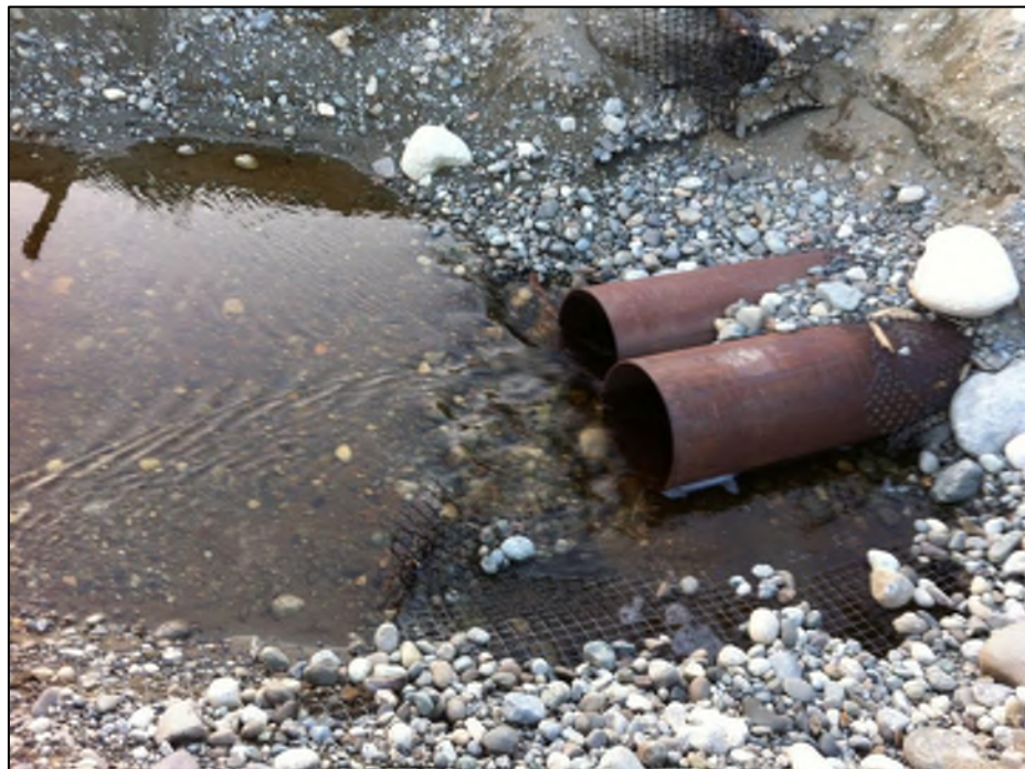
Figure 12: Inlet on project left to move impounded water with two 16" pipes. May 2, 2014. Notice the level of the impounded water has dropped significantly since April 22, 2014.
