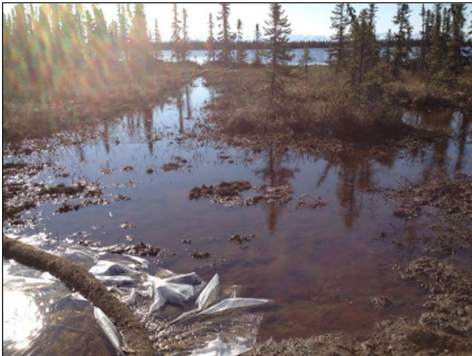
Figure 20: Cleaned-up wetlands after fill removal. May 9, 2014.
