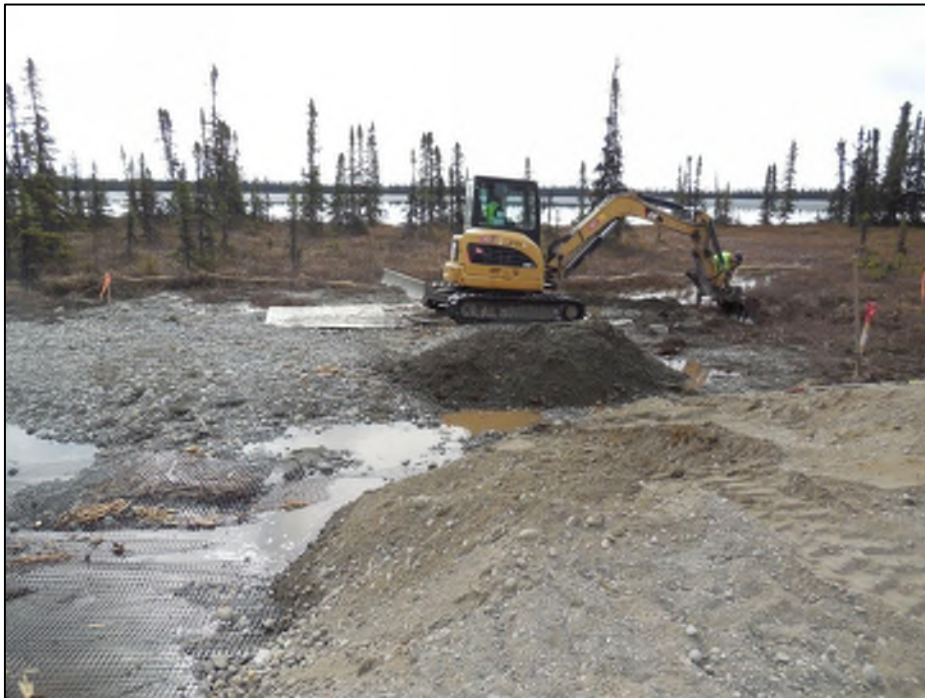
Figure 16: CAT 305 excavator on small crane pad removing fill from wetlands on project right. May 5, 2014.
