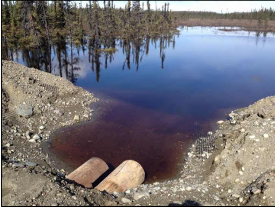
Figure 9: Inlet on project left to move impounded water with two 12" pipes. April 29, 2014. Notice the level of the impounded water has dropped significantly since April 22, 2014.
