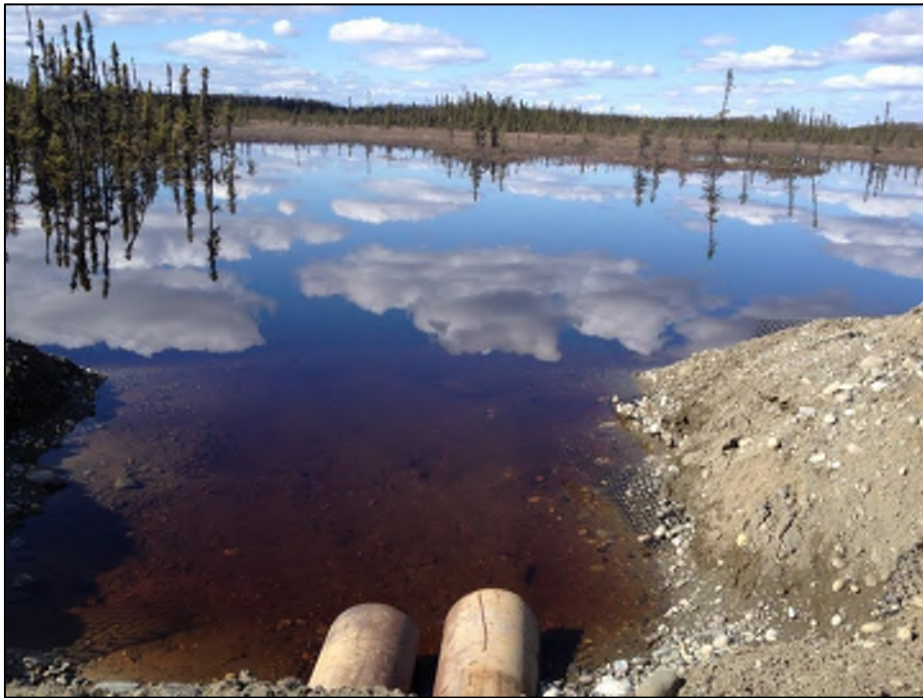
Figure 6: Inlet on project left to move impounded water with two 12" pipes. April 24, 2014. Notice the level of the impounded water has dropped significantly since April 22, 2014.
