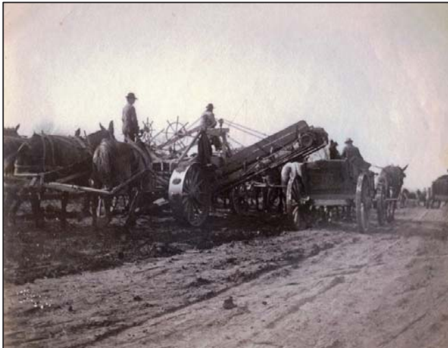
Excavation for the line near Raytown, Missouri.
