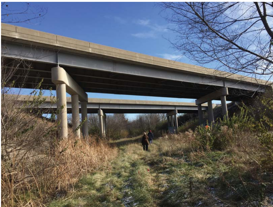
Overhead bridge at 63 rd Street near Raytown.
