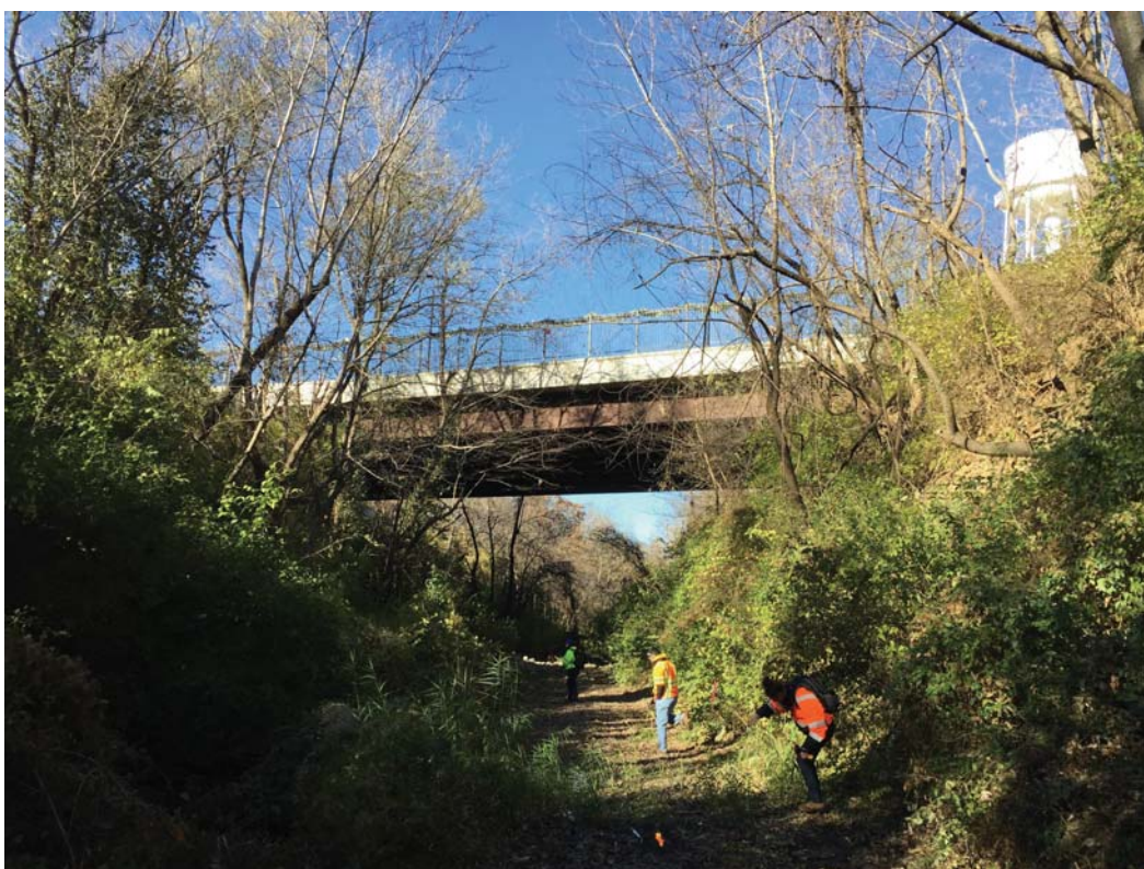
The I-470 overhead bridge near Vale.
