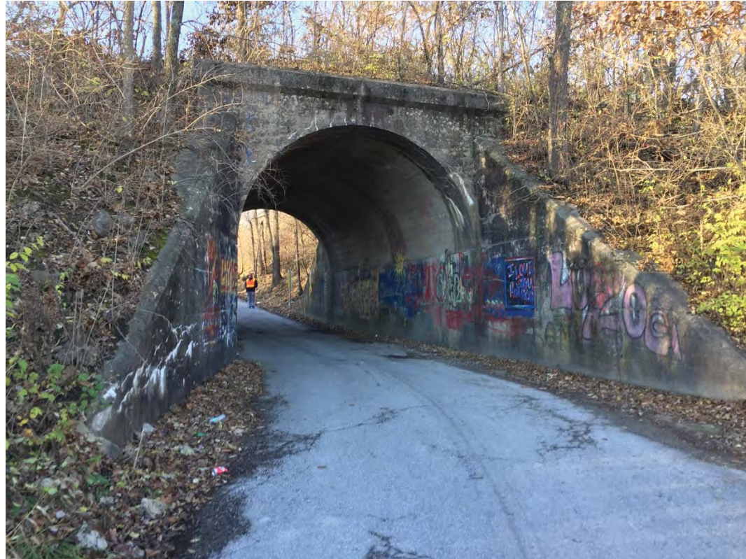
Skewed concrete arch bridge at Frost Rd. and east 79 th St.; view looking northeast.
