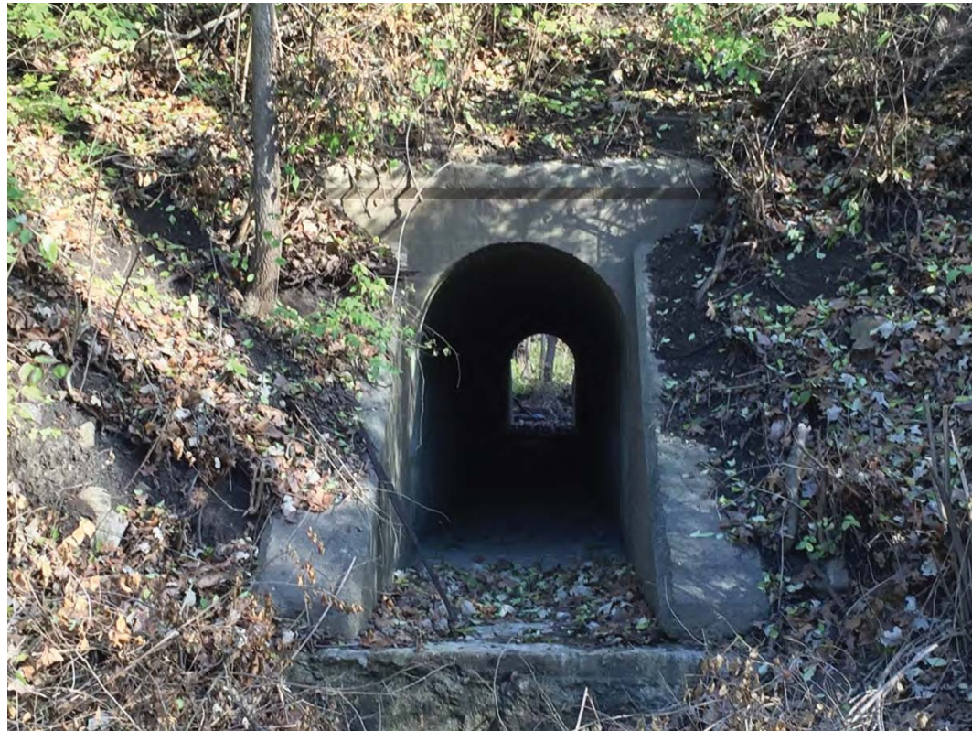
Concrete arch culvert north of NW Chipman Rd.; view looking east from the right-of-way.
