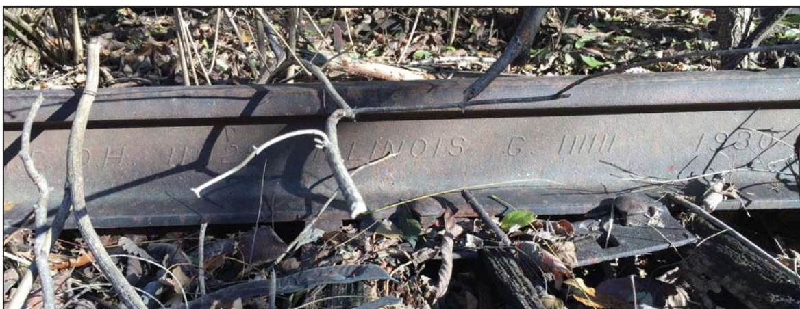
Two examples of rail typical in the study area, manufactured by the Illinois Steel Co.
