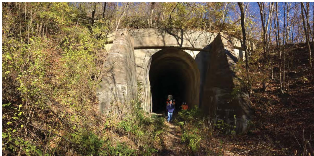
Panoramic view of Vale Tunnel, looking north.
