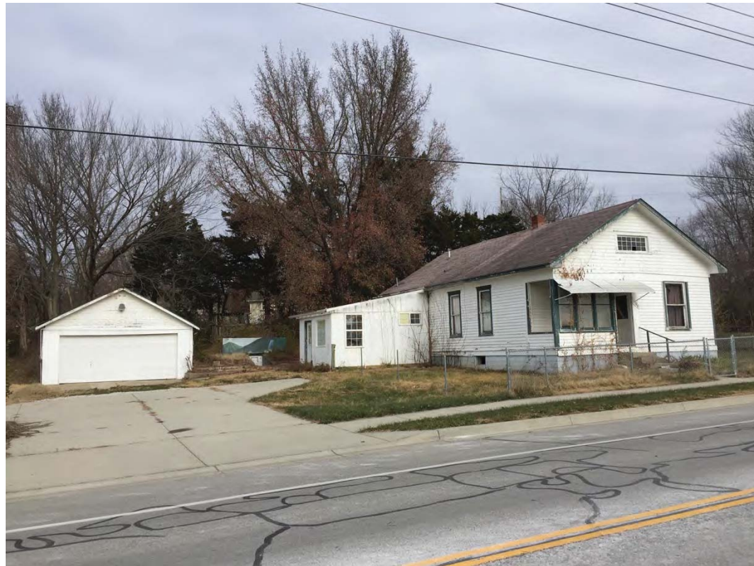
1700 Southwest Longview Rd.; view looking east, southeast.
