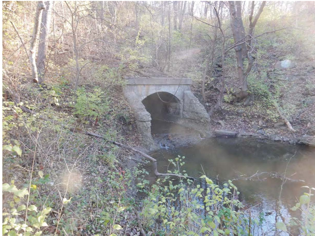
Concrete arch culvert near Blue Ridge Cutoff and East 47 th St. (KML 111)
