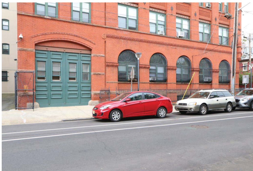
Plate 75: Detail view of the ground level of the Thomas J. Stewart Company Building illustrating the complementary metal window guards installed when the building was converted for residential use.
