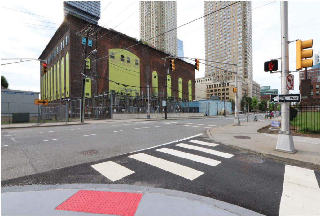
Plate 92: General view of the north and west elevations of the Hudson & Manhattan Railroad Powerhouse.
