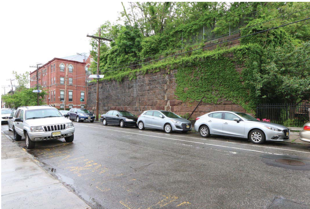
Plate 10: View of the westernmost segment of the Pennsylvania Railroad Harsimus Branch Embankment at Sixth and Brunswick streets.
