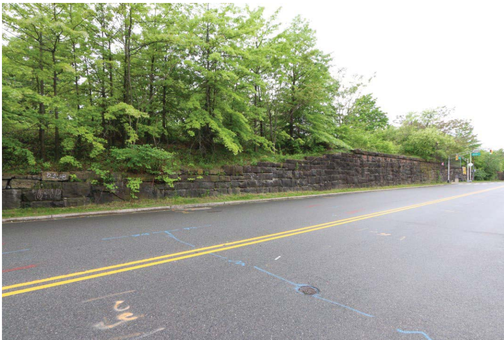
Plate 20: View of the Pennsylvania Railroad Harsimus Branch Embankment along Sixth Street, between Manila Avenue and Luis Munoz Marin Boulevard. Note how the north elevation steps down as the segment stretches east, towards the Hudson River.
