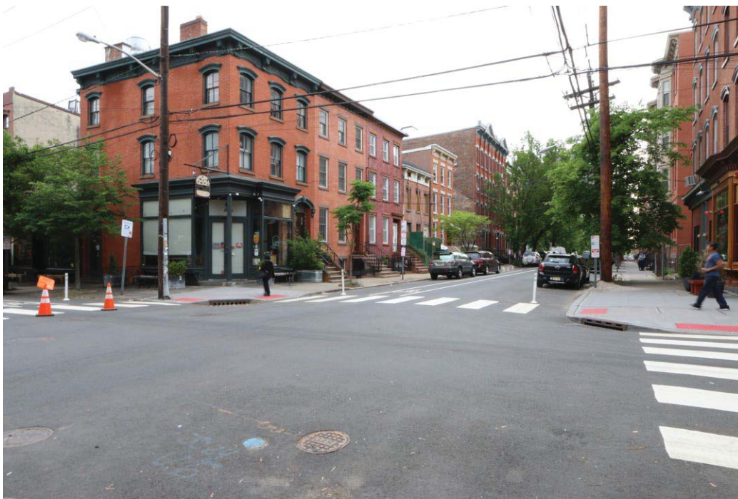
Plate 49: General view of the Harsimus Cove Historic District at the intersection of First and Erie streets.
