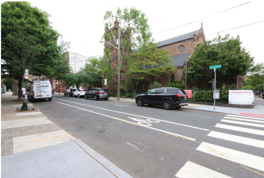
Plate 51: General view of the Grace Van Vorst Church at 35 Erie Street, which is a contributing resource to the Harsimus Cove Historic District.
