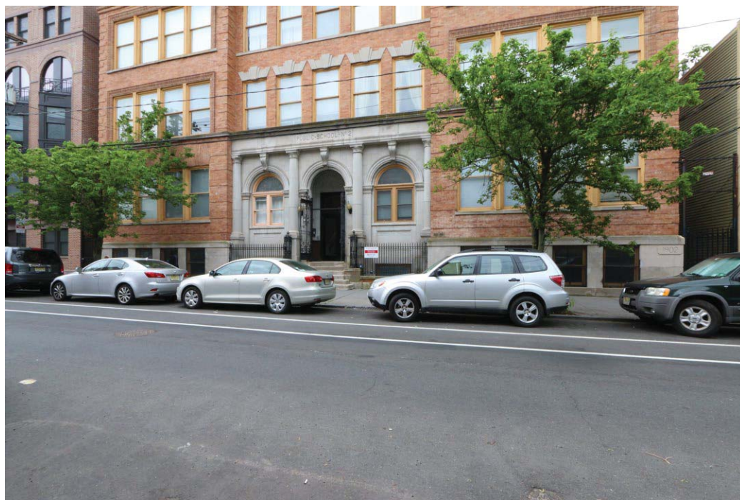
Plate 54: View of Public School No. 2 at 60-66 Erie Street, a contributing resource to the Harsimus Cove Historic District.
