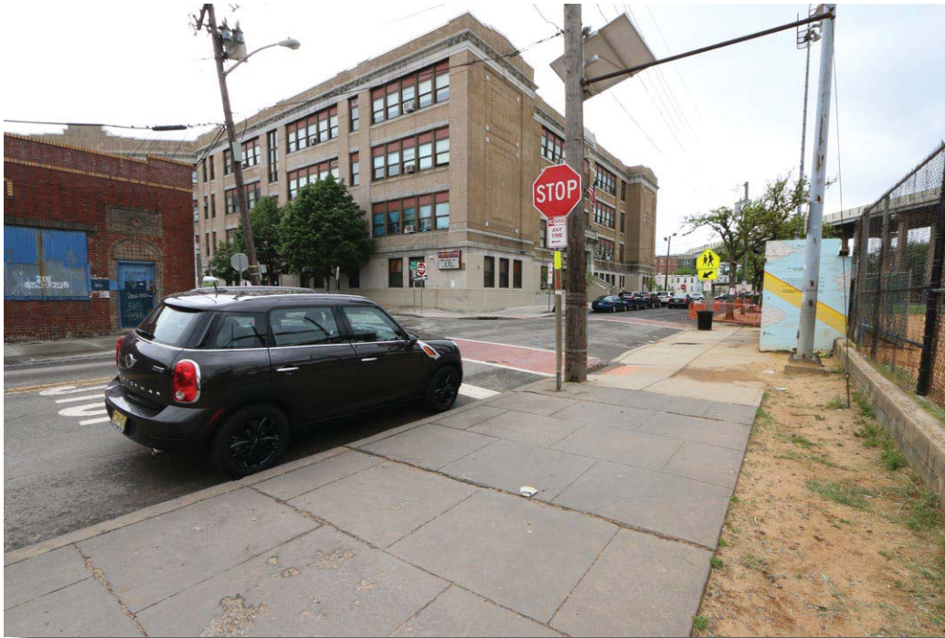
Plate 7: View of Public School No. 5 from Merseles Street. Mary Benson Park is partly visible to the right (west).
