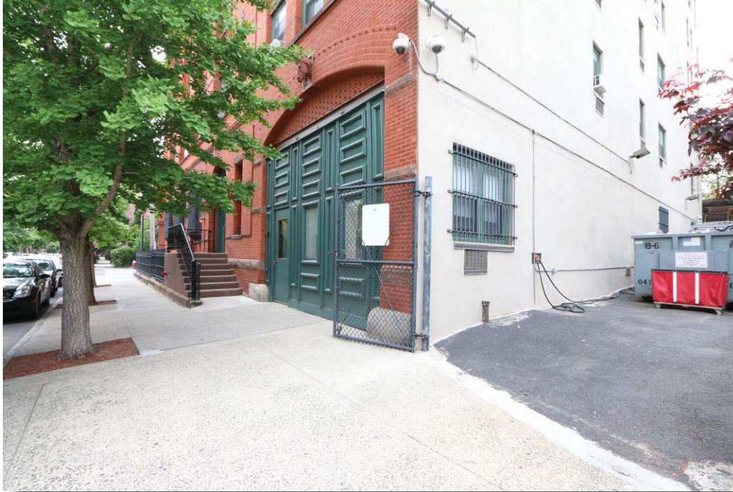
Plate 77: Detail view of the south elevation of the Thomas J. Stewart Company Building.
