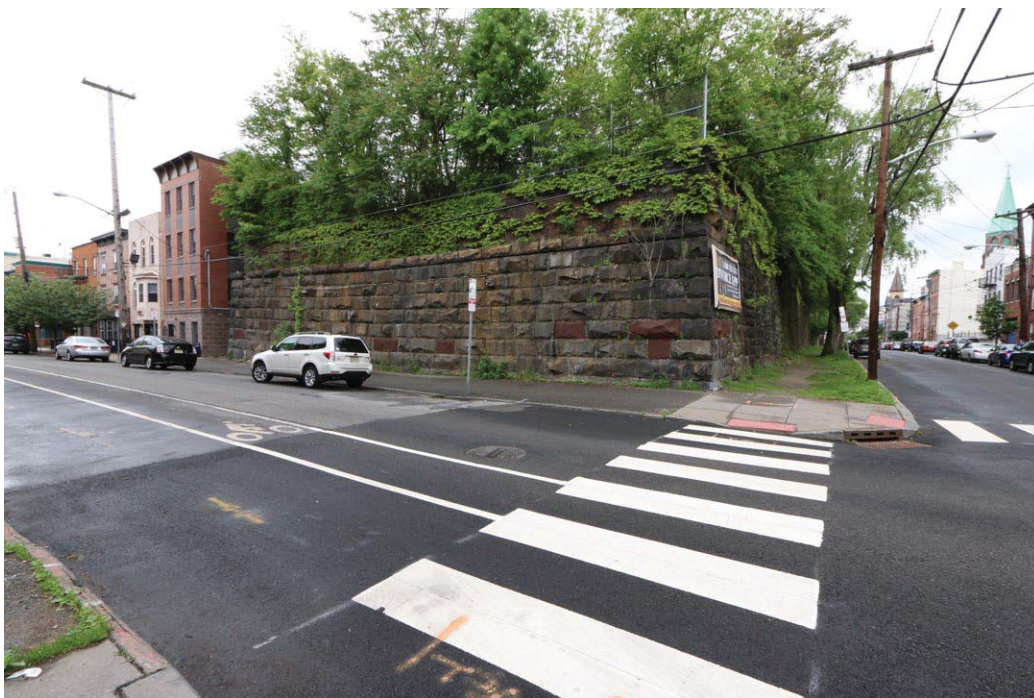
Plate 12: View of one of the bridge seats facing Coles Street, at Sixth Street, of the Pennsylvania Railroad Harsimus Branch Embankment.
