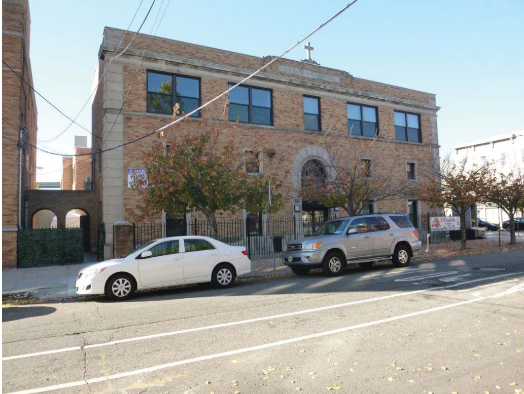
Plate 104: View of the Holy Rosary School, built in 1953 and designed by Anthony De Pace.
