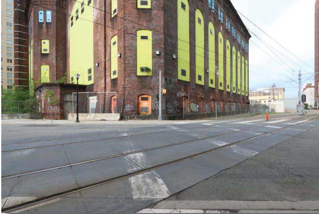
Plate 94: View of the canted northeast corner of the Hudson & Manhattan Railroad Powerhouse.
