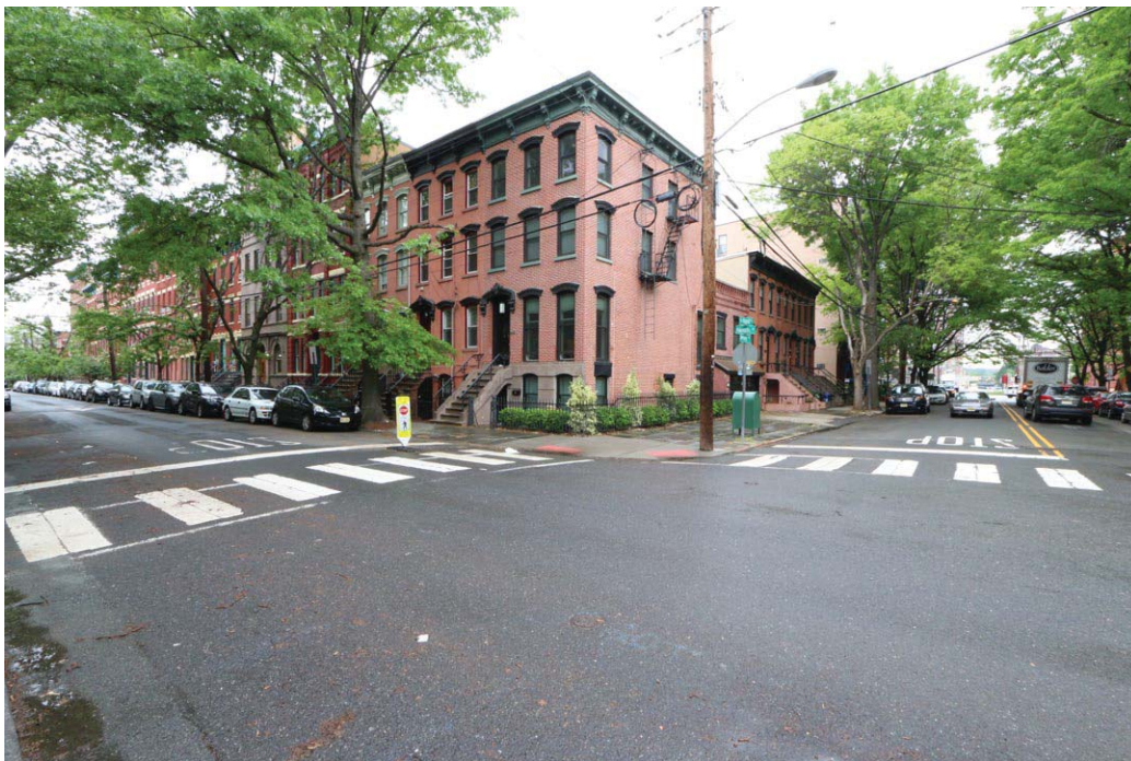
Plate 33: View looking towards the intersection of Ninth Street and Jersey Avenue. This view encompasses most of the buildings part of the Hamilton Park Historic District Extension.
