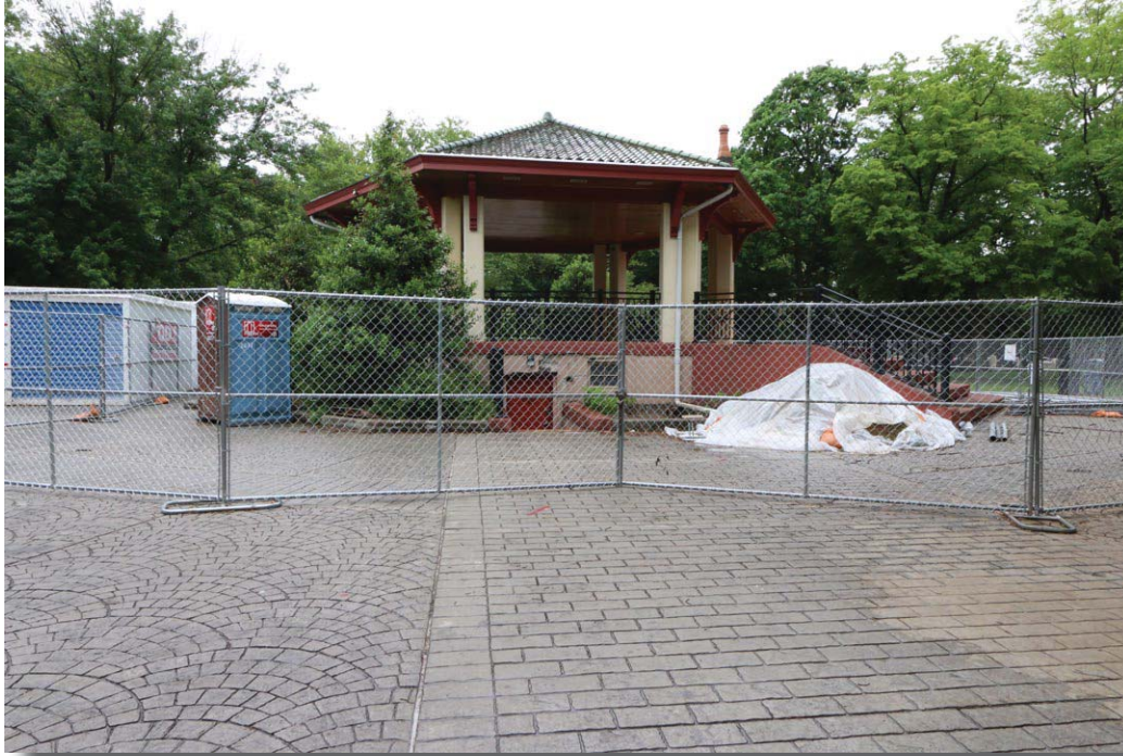
Plate 34: View of the gazebo sited in the center of Hamilton Park, a mid-nineteenth-century park square that contributes to the Hamilton Park Historic District.
