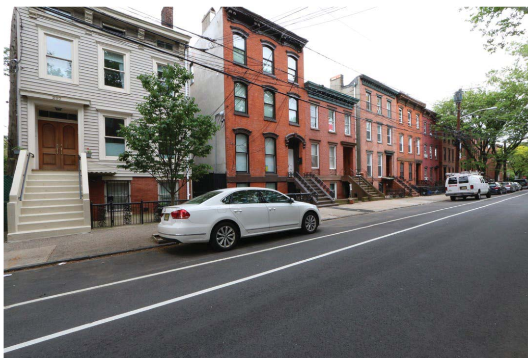
Plate 57: View along the south side of Fourth Street, between Jersey Avenue and Erie Street, within the Harsimus Cove Historic District.
