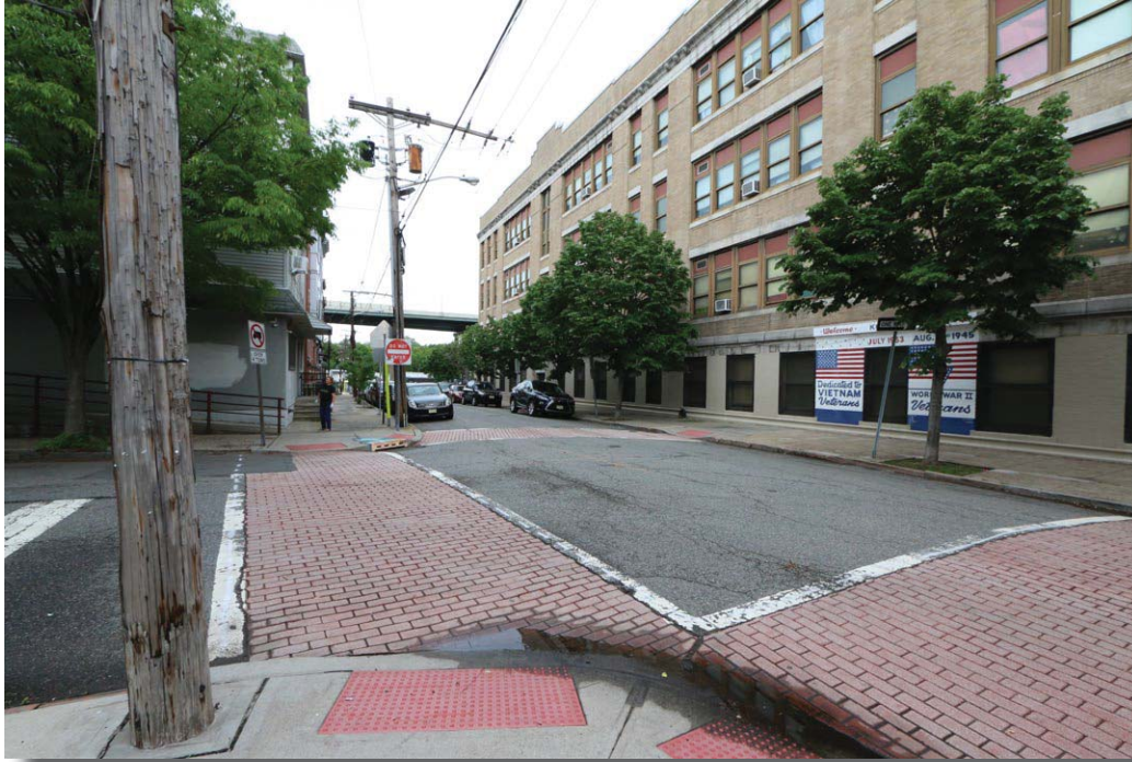
Plate 9: View along the south elevation of Public School No. 5 on Third Street.
