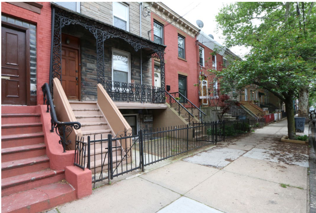
Plate 61: Detail view of some of the characteristic decorative ironwork found throughout the Harsimus Cove Historic District.
