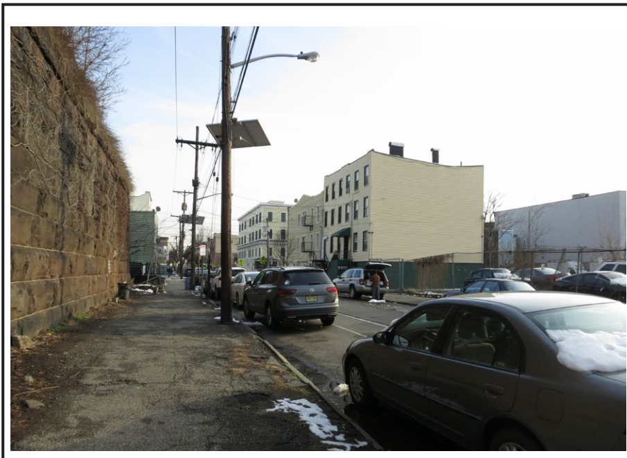
View along Brunswick Street from the Pennsylvania Railroad Harsimus Branch Embankment at Sixth Street.
