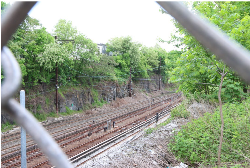
Plate 2: General view along the New Jersey Railroad Bergen Cut Historic District, which is a key contributing resource to the Pennsylvania Railroad (New York to Philadelphia) Historic District.
