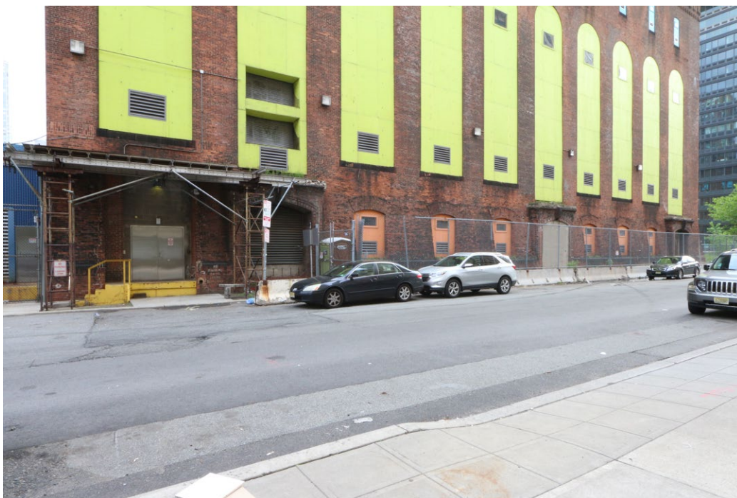
Plate 93: Detail view of the ground level of the Hudson & Manhattan Railroad Powerhouse.
