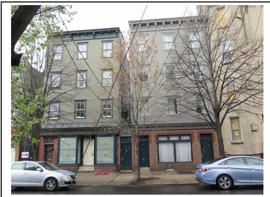
View of 365 Second Street at right, the former location of Holy Grace Hall, between Monmouth and Brunswick streets.
