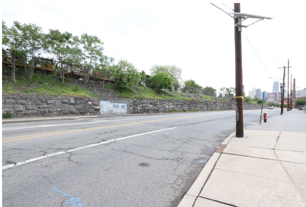
Plate 3: View along Christopher Columbus Drive looking towards the stone embankment of the Pennsylvania Railroad (New York to Philadelphia) Historic District as the district extends to its terminus at Brunswick Street.
