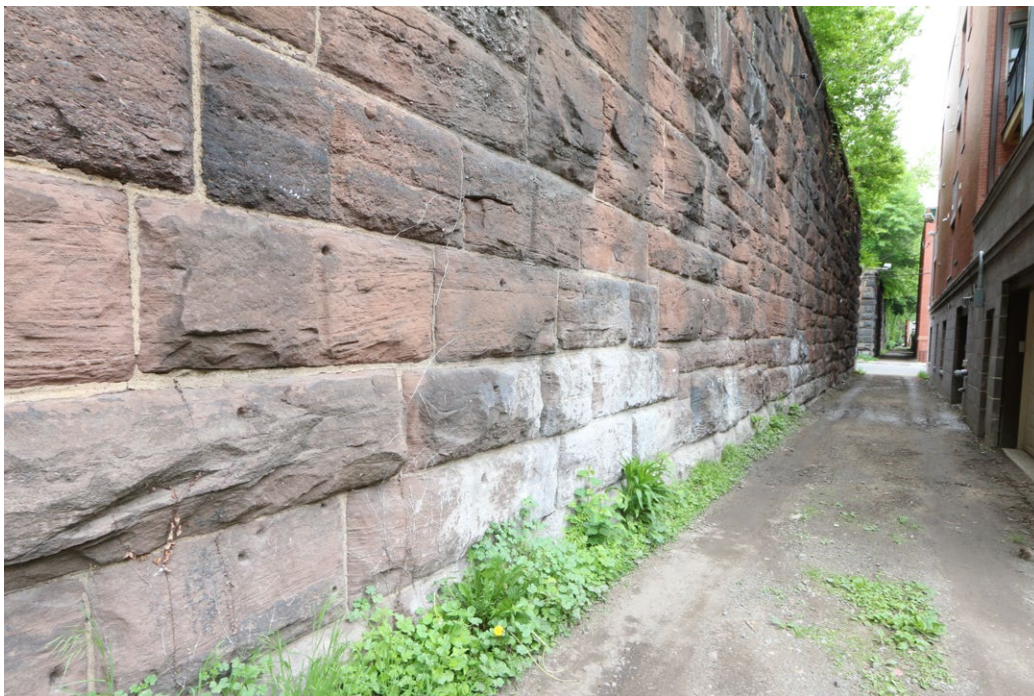
Plate 14: Detail view of the soft brown sandstone used for the construction of the south retaining walls of the Pennsylvania Railroad Harsimus Branch Embankment.
