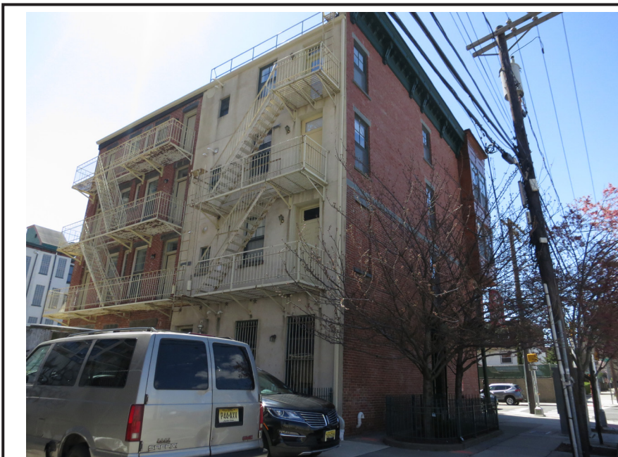
View of the rear (east) and north elevations of the building at 382 Luis Munoz Marin Boulevard.
