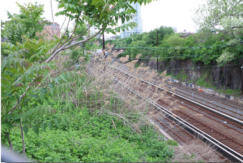
Plate 1: General view along the New Jersey Railroad Bergen Cut Historic District, which is a key contributing resource to the Pennsylvania Railroad (New York to Philadelphia) Historic District.
