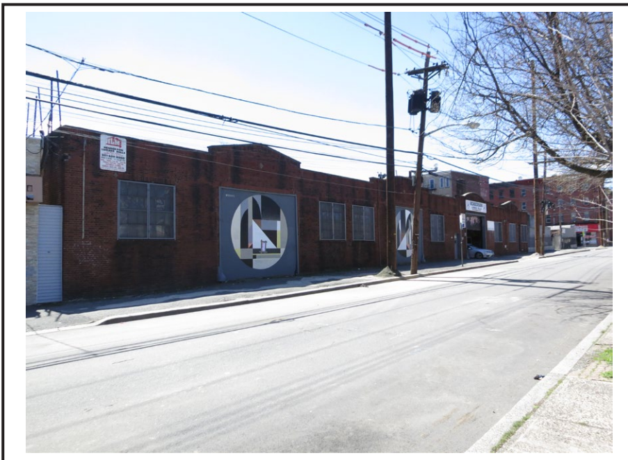
Overview of Henderson Lumber Mills at 195 First Street.
