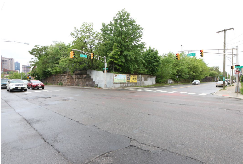
Plate 21: Perspective view of the easternmost segment of the Pennsylvania Railroad Harsimus Branch Embankment, at the intersection of Sixth Street and Luis Munoz Marin Boulevard.
