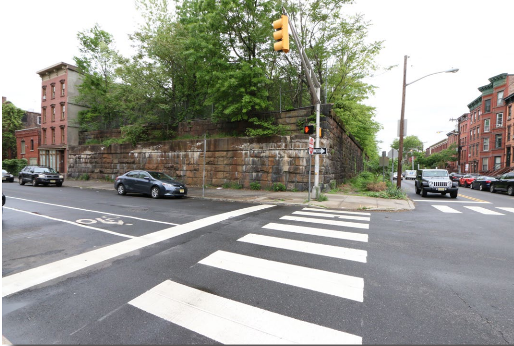
Plate 17: View of the bridge seat and abutment of the Pennsylvania Railroad Harsimus Branch Embankment at the intersection of Sixth and Erie streets. Note how the height of the embankment is lower as the linear segments approach the Hudson River.
