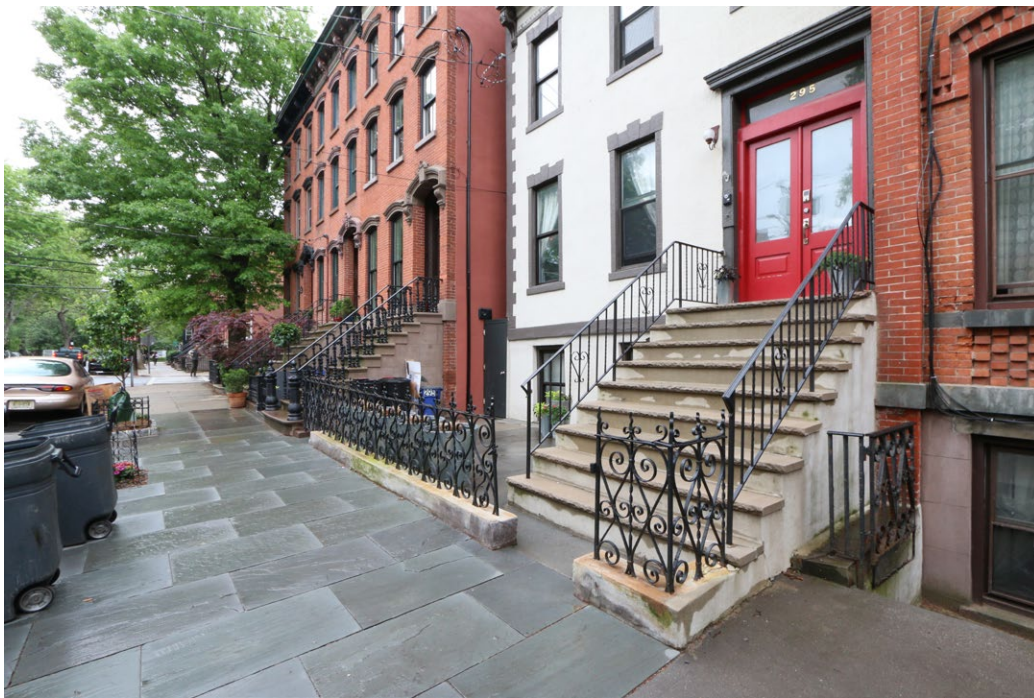
Plate 28: Representative view of the decorative features common on many of the extant row houses composing the Hamilton Park Historic District, such as the ornamental ironwork, lintels, stone water tables, and distinct entrance stoops.
