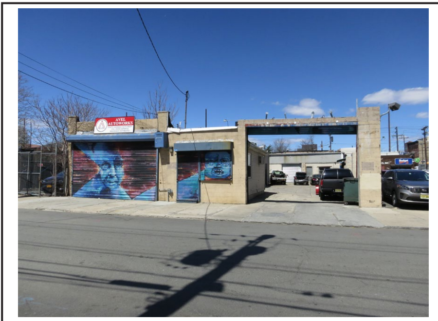
View of the rear (southern) elevation of 181 First Street at right, and the southern garage building associated with Avel Autoworks on Bay Street at left.
