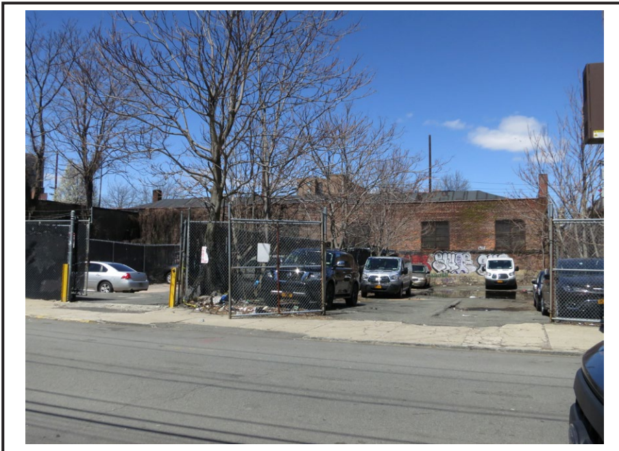
View of the rear (south) elevation of 195 First Street.
