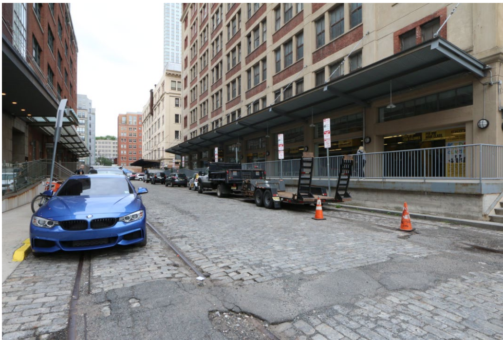
Plate 81: General view along Provost Street within the Warehouse Historic District, adjacent to the Great Atlantic & Pacific Tea Company Warehouse illustrating the original cobblestone paving and rail siding.
