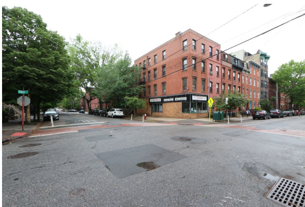
Plate 37: General view within the Hamilton Park Historic District at the intersection of Eight Street and Jersey Avenue.
