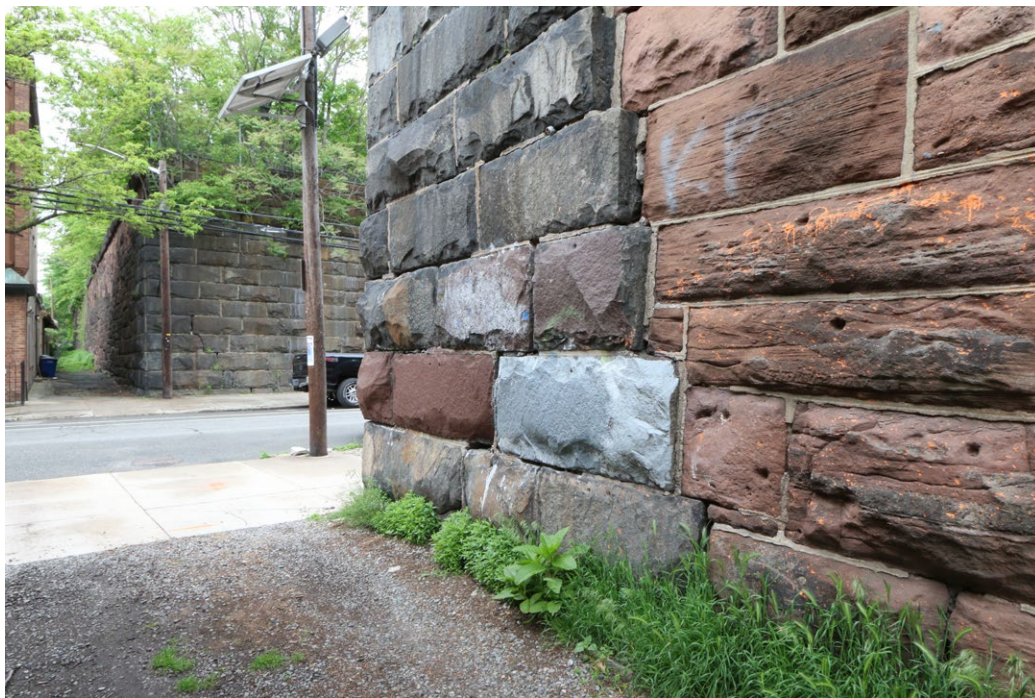
Plate 15: Detail view of the Pennsylvania Railroad Harsimus Branch Embankment which depicts the different types of stone used in the embankment's construction. For bridge abutments, as shown here, granite was used whereas as soft brown sandstone was used for the south retaining walls.
