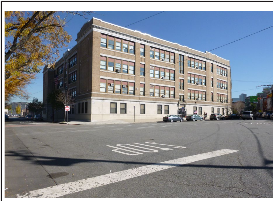
View along Merseles Street from the intersection of Third Street showing the National Register-eligible Public School No. 5.
