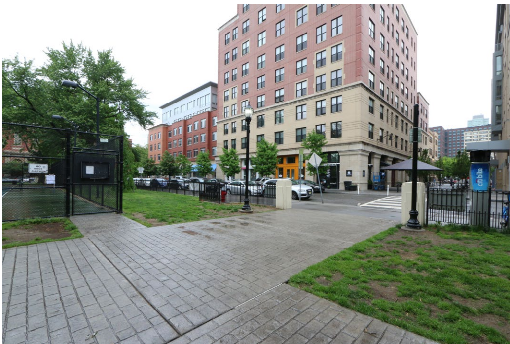
Plate 35: General view of some of the modern infill extant in the Hamilton Park Historic District. Note the use of materials that are compatible in type and color to the existing buildings of the district.
