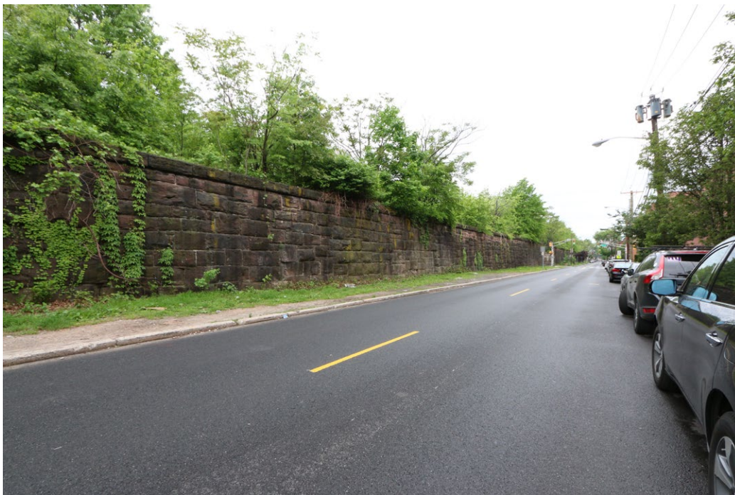
Plate 18: General view of the Pennsylvania Railroad Harsimus Branch Embankment, along Sixth Street between Erie Street and Manila Avenue.
