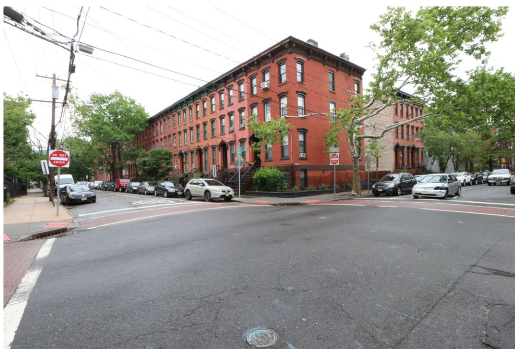
Plate 39: General view within the Hamilton Park Historic District at the intersection of Eight and Erie streets.
