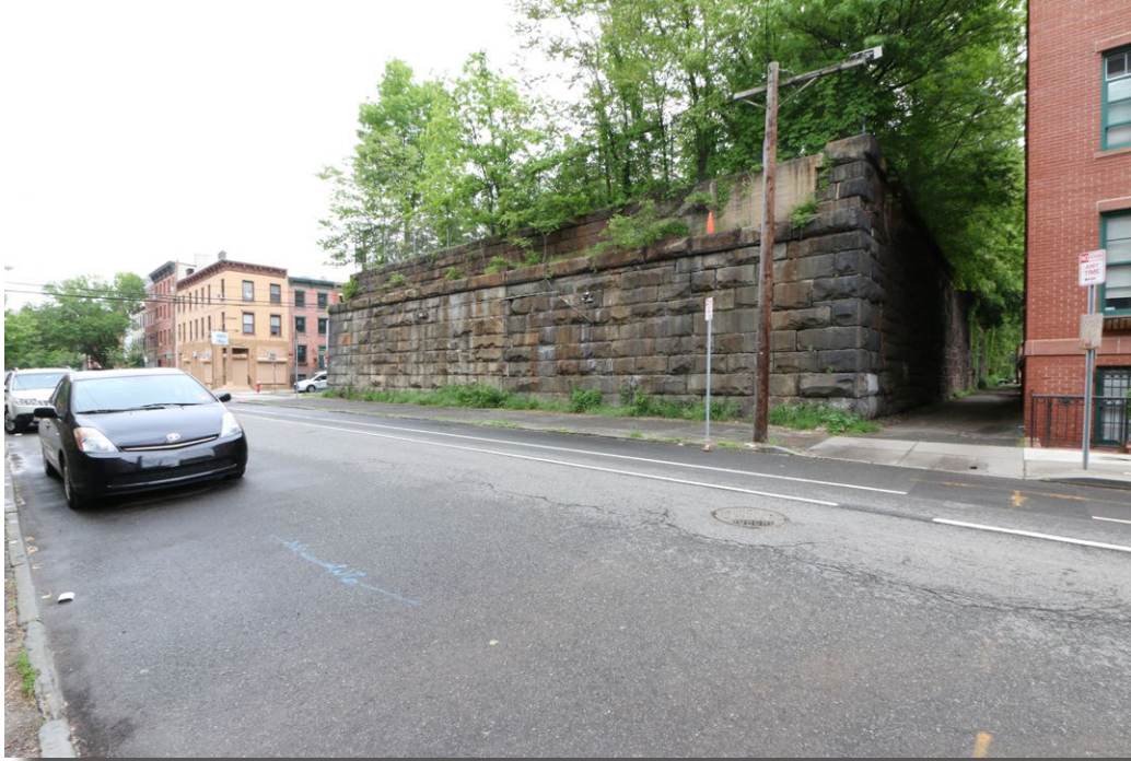
Plate 13: General view of one of the bridge seats facing Coles Street, at Sixth Street, of the Pennsylvania Railroad Harsimus Branch Embankment.
