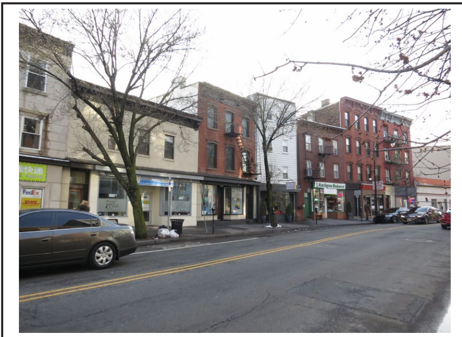
View of mixed-used tenements along Newark Avenue, between Second and Third streets, with the extant Antique Bakery, a longstanding Italian business, at right.
