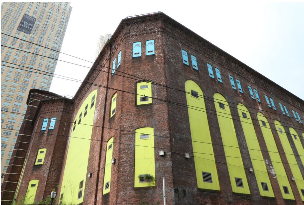
Plate 95: Detail view of the patterned and corbelled brickwork of the cornice of the Hudson & Manhattan Railroad Powerhouse. Note the distinct five-story, arched windows soldiered across the visible elevations.
