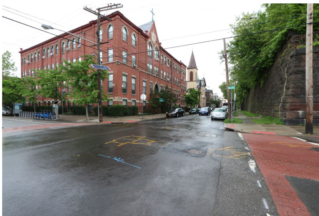
Plate 25: View of the school of the St. Anthony's Polish Roman Catholic Church and School Complex. Visible are the architecturally notable pointed-arched windows, ornate window aprons, and pilasters.
