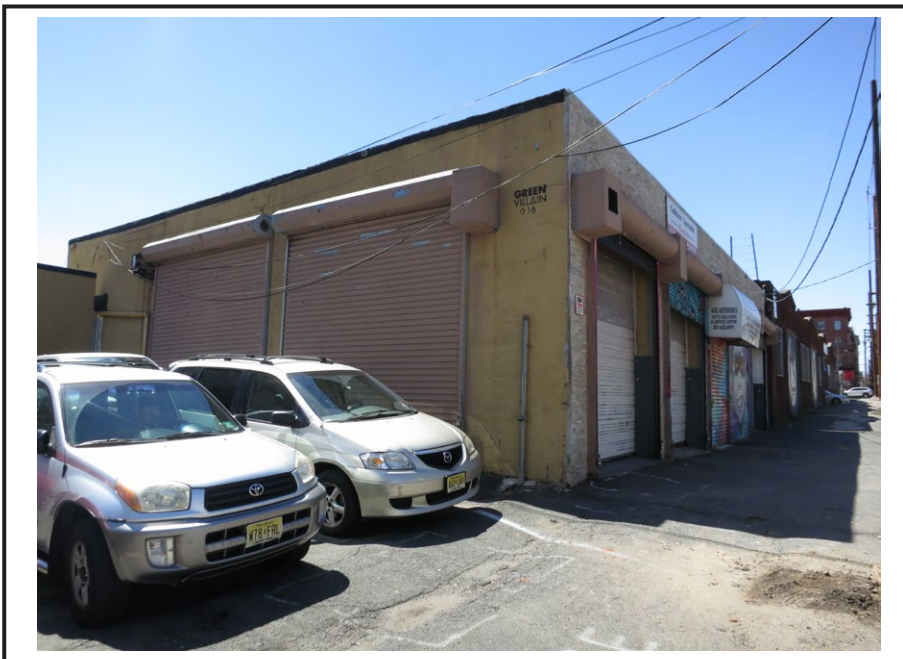
View of the primary and east elevations of 181 First Street.
