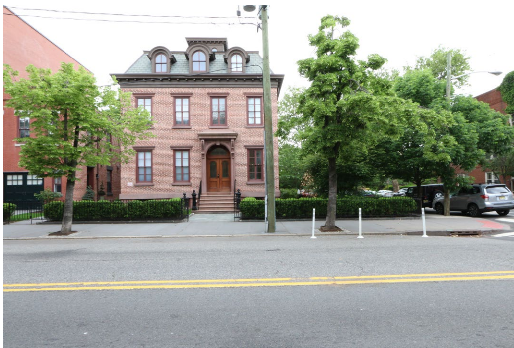
Plate 58: View of one of the few freestanding buildings within the Harsimus Cove Historic District, at the southwest corner of the intersection of Fourth Street and Jersey Avenue.
