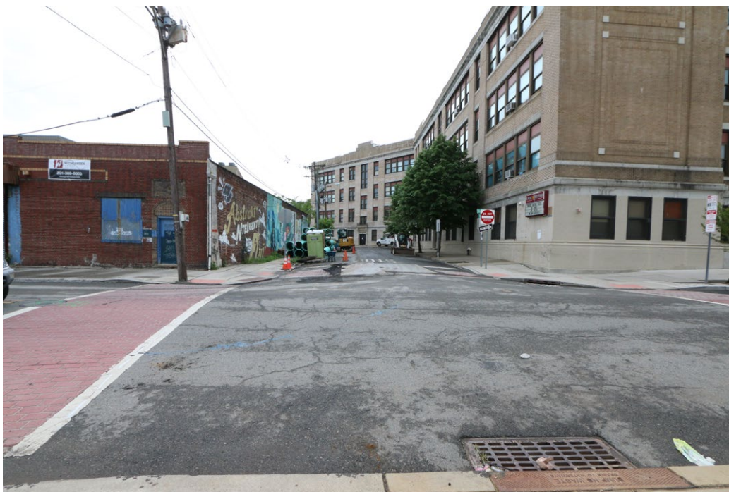
Plate 8: View down Fourth Street depicting the bending footprint of Public School No. 5.
