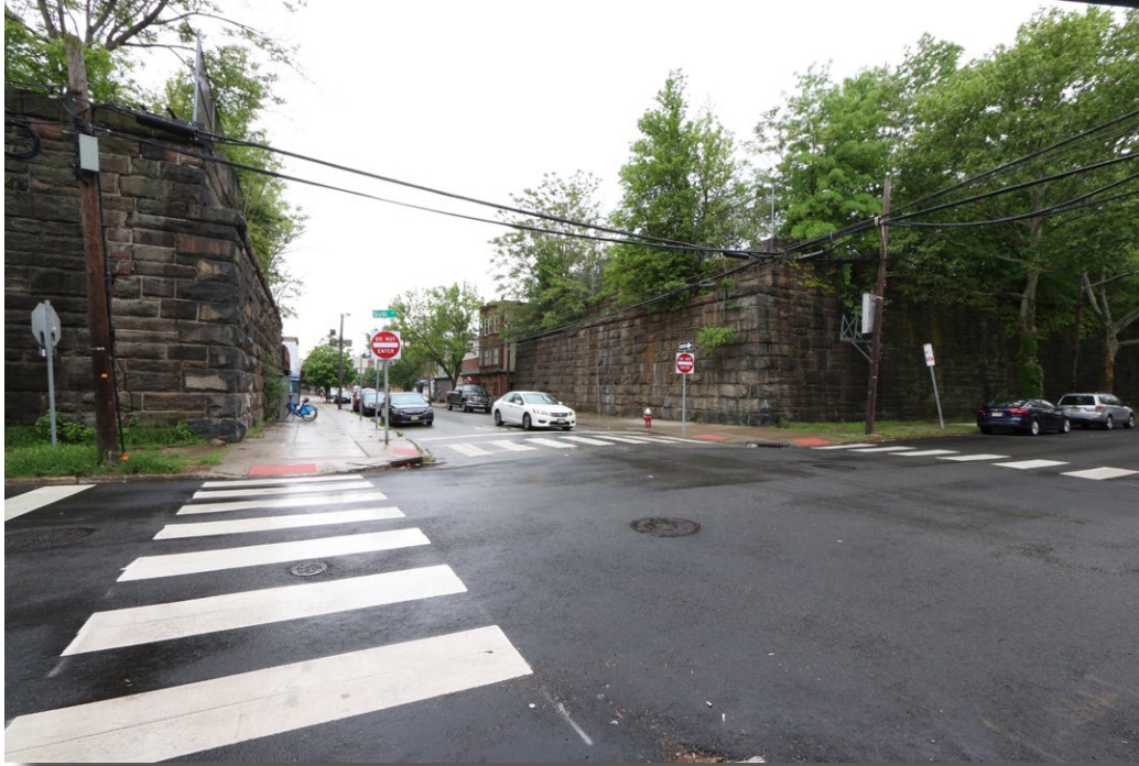
Plate 11: General view of the Pennsylvania Railroad Harsimus Branch Embankment at the intersection of Sixth and Monmouth streets.
