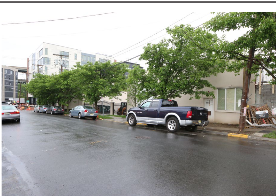
Detail of infill construction and surface parking lot on Sixth Street at right and contemporary mid-rise residential construction on the west side of Division Street at left.
