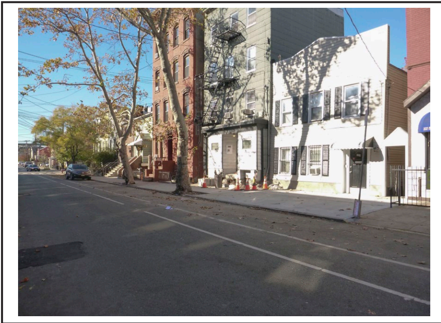
View of late nineteenth- and early twentieth-century residences on the north side of Fifth Street, looking toward Monmouth Street.
