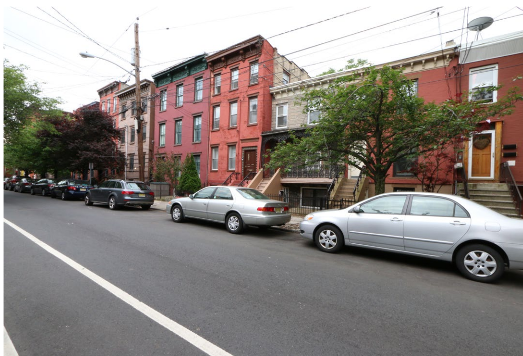
Plate 63: View along the south side of Fifth Street, between Coles Street and Jersey Avenue, within the Harsimus Cove Historic District.
