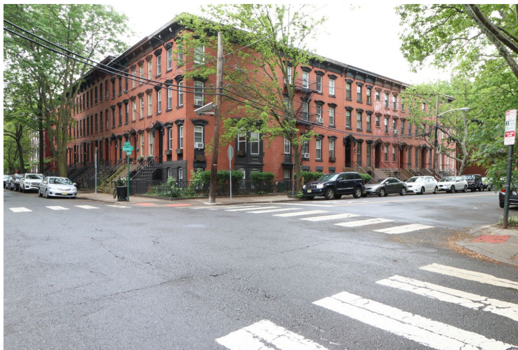
Plate 30: General view of the intact continuity of row houses of the Hamilton Park Historic District, at the intersection of Pavonia Avenue and Coles Street, adjacent to Hamilton Park.
