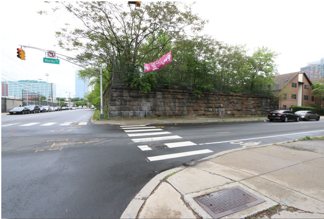
Plate 19: View of the west elevation of the easternmost segment of the Pennsylvania Railroad Harsimus Branch Embankment.
