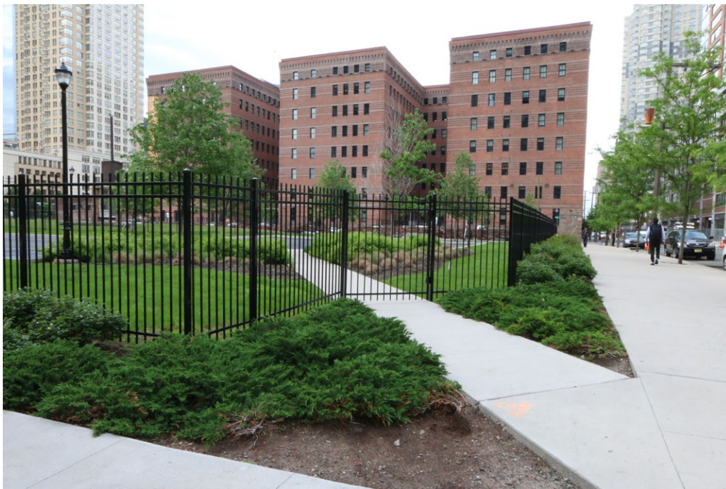
Plate 84: General view of the Butler Brothers' Warehouse, built 1905. This large, monumental industrial building is individually listed on the National Register of Historic Places and is a key contributing resource to the Warehouse Historic District.
