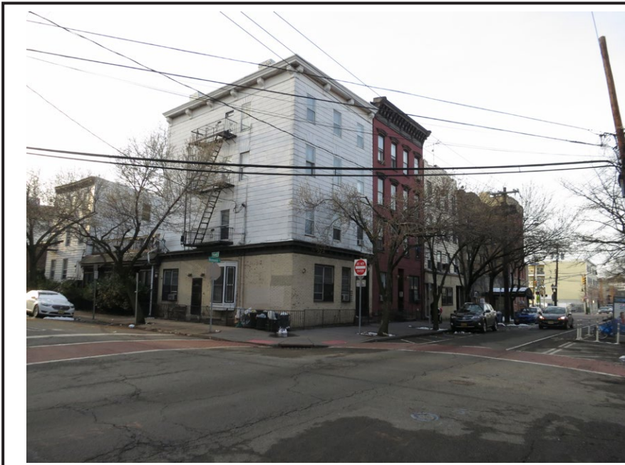
View of extant four-story tenements along Brunswick Street from Third Street. The intersection with Newark Avenue and Fourth Street is visible at right.
