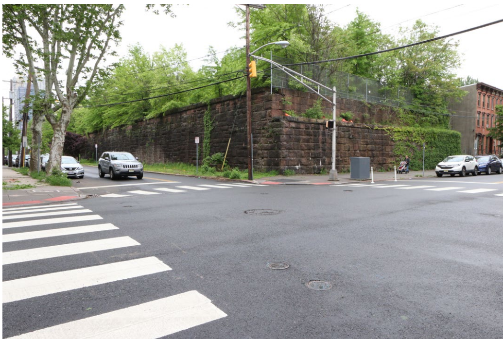
Plate 16: General view of the bridge seat and abutment of the Pennsylvania Railroad Harsimus Branch Embankment at the intersection of Sixth Street and Jersey Avenue. For the north retaining walls of the embankment, a conglomerate-type of stone was used.
