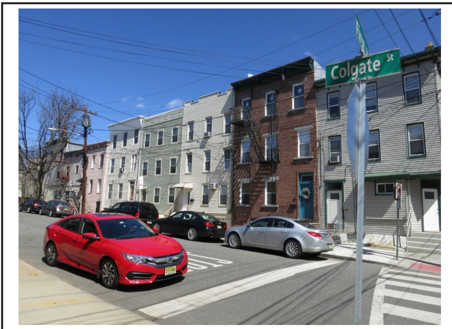
View of late nineteenth-century tenements along Colgate Street, north of First Street.
