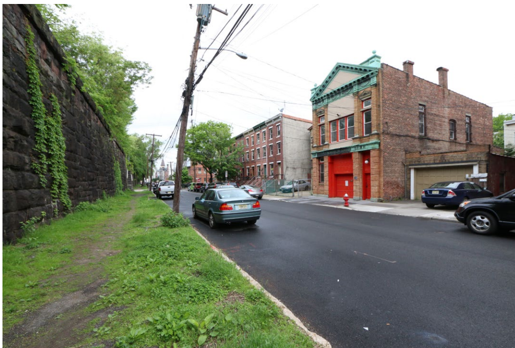
Plate 48: View of 278 Sixth Street, a late nineteenth-century firehouse that features buff-colored brick, limestone, and copper ornamentation, and which contributes to the Hamilton Park Historic District.
