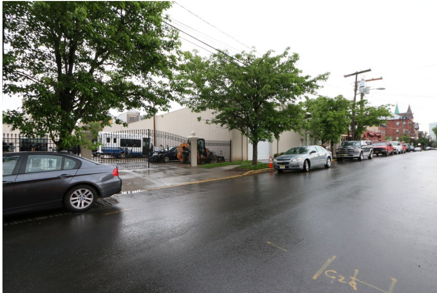
Detail of infill construction and surface parking lot on Sixth Street, east of Division Street.
