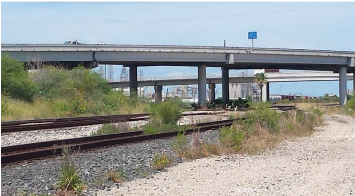
Figure 2-5: Photo of the area proposed for construction of the new rail line and crossing of the existing UP rail line (SH 275/Harborview Drive bridge [foreground] and 51 st Street/Pelican Island Causeway bridge [background] over the project area. Proposed track alignment would be to the left of the tracks shown.)
