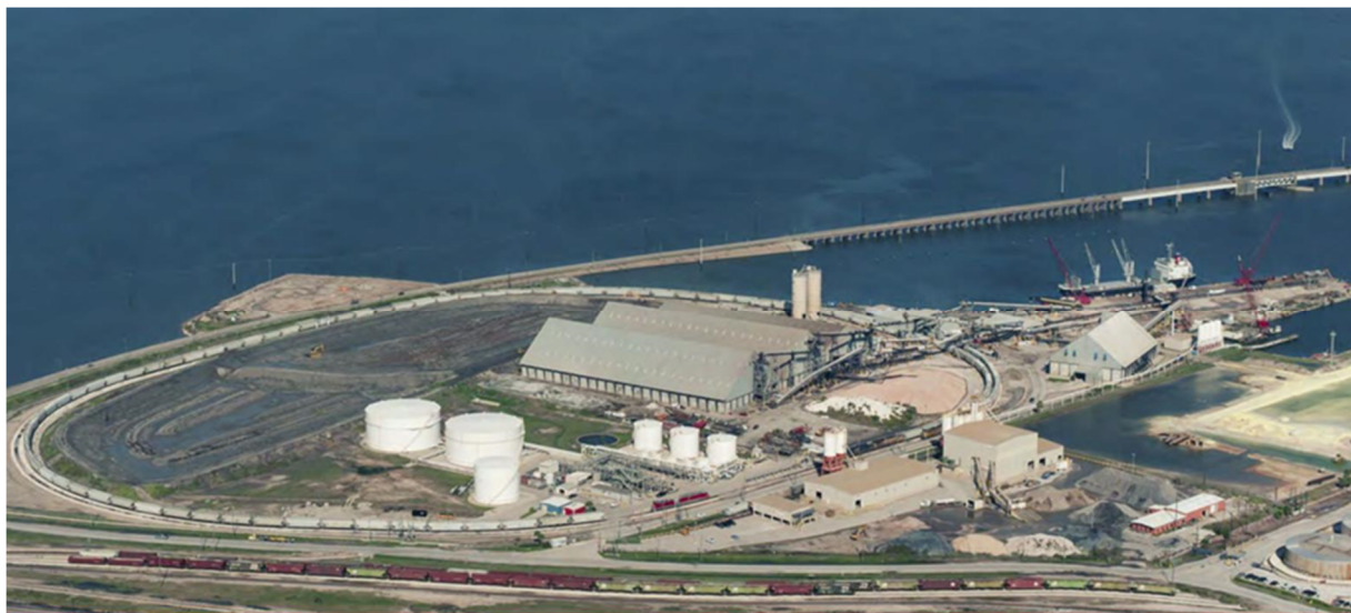
Figure 1-1 - Texas International Terminals, Galveston, Texas
