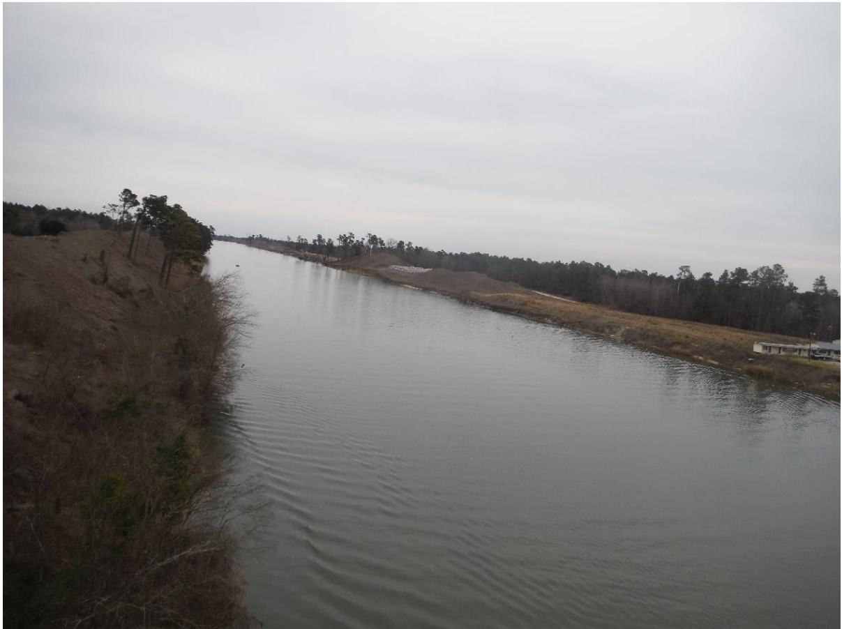
Photograph 2 Diversion Canal, view southeast
