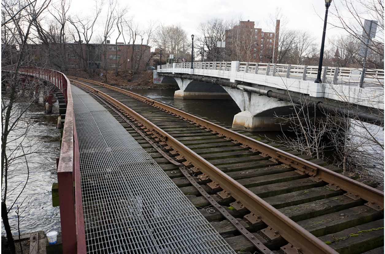
Rail bridge next to the Monroe Street Bridge
