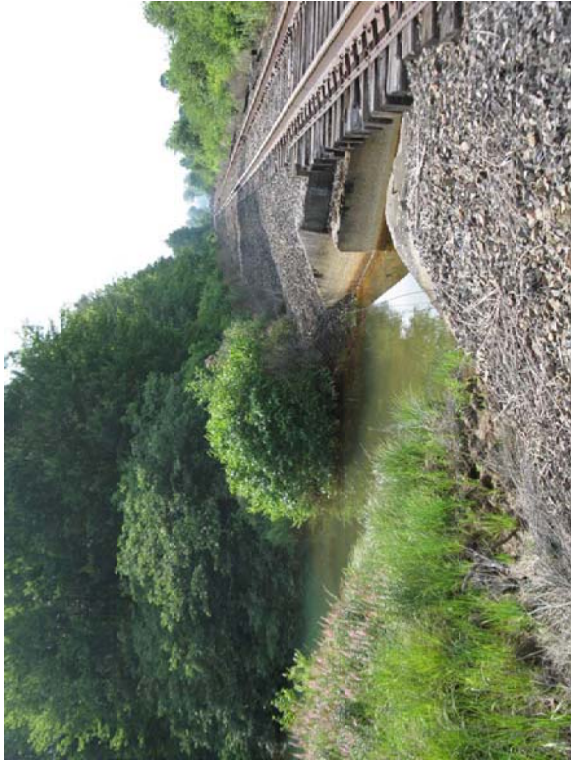
Photograph No. 5: Existing railroad where new Laurel Run creek crossing segment ties down.
