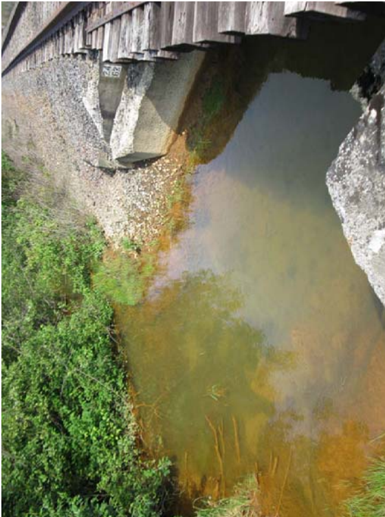
Photograph No. 7: Opposite side of existing bridge with no Sparganium in direct area but is just out of the work area so indirect impacts could occur if bridge replacement occurs.
