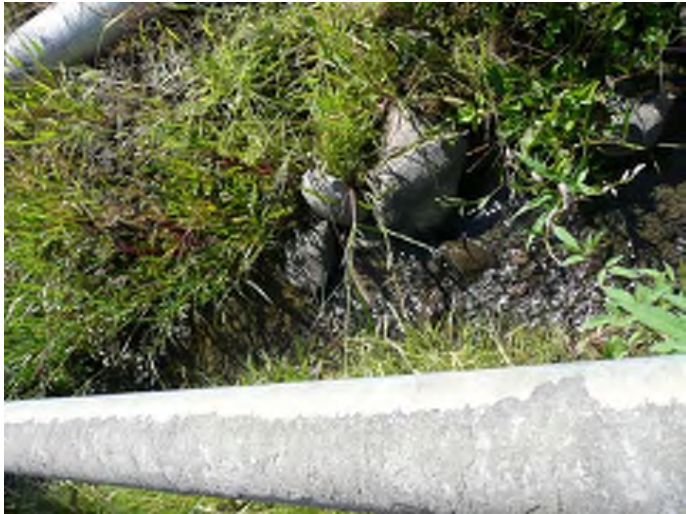
View of Detail of Canal EL20 Extension and pipe taken 8/21/2007 Photography Neg. No (Roll No./Frame No.): P1000497.jpg Comments:
