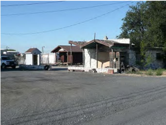
View of north and east facades, facing southwest. taken 8/21/2007 Photography Neg. No (Roll No./Frame No.): Comments: Photo No. P1000457.jpg
