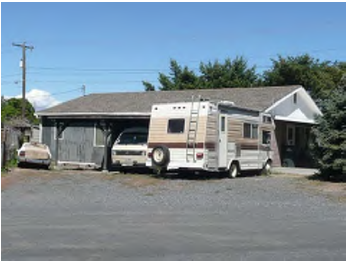
View of west façade, facing north northeast. taken 8/21/2007 Photography Neg. No (Roll No./Frame No.): Comments: Photo No. P1000505.jpg
