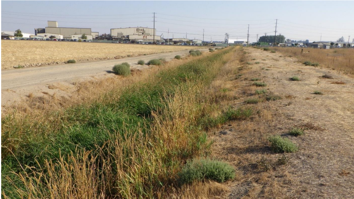
Figure 4. Overview of canal RCD 180+182, facing north.
