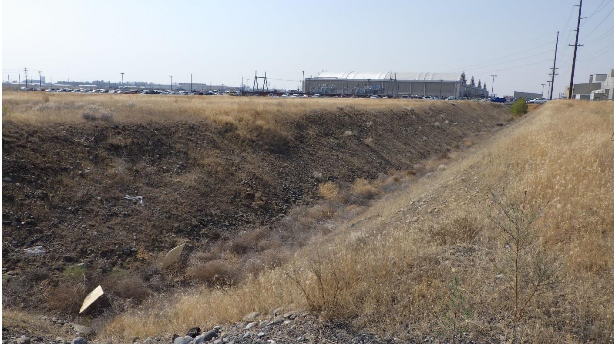
Historic canal (8 Place Hangar Drainage Ditch) on parcel 171006000, facing west.
