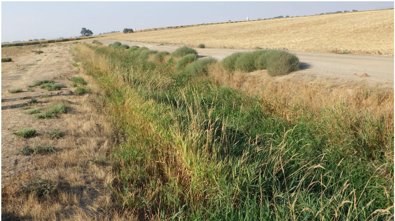
Historic canal RCD 180+182 bordering the west side of parcel 110069492, facing south.
