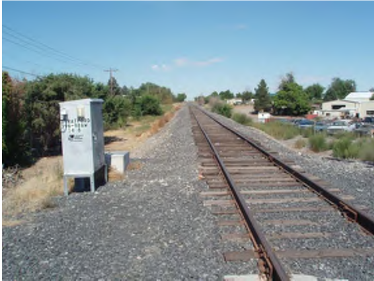
Photo 9: View of existing Columbia Basin Railroad (Segment 3) at Stratford Road crossing looking northwest.
