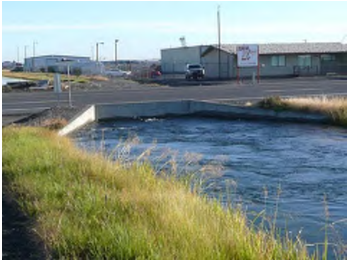
View of Ditch No. EL20 Culvert at Wheeler Road, View North taken 8/21/2007
