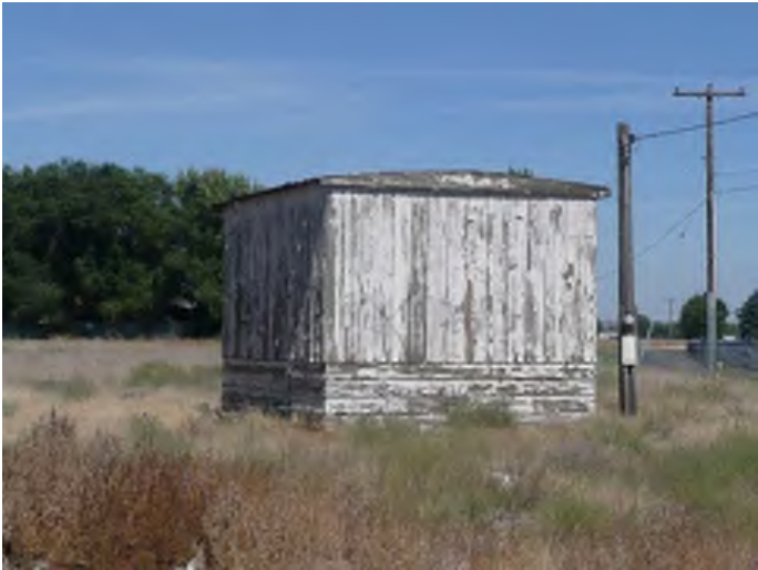
View of west and north facades, facing southeast. taken 8/21/2007 Photography Neg. No (Roll No./Frame No.): Comments: Photo No. P1000546.jpg
