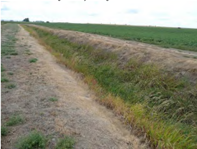
Photo 3: View of RCD 180+2 (Map Id. No. 18) and proposed Segment 1 crossing location looking south with active agricultural field to right of photo.
