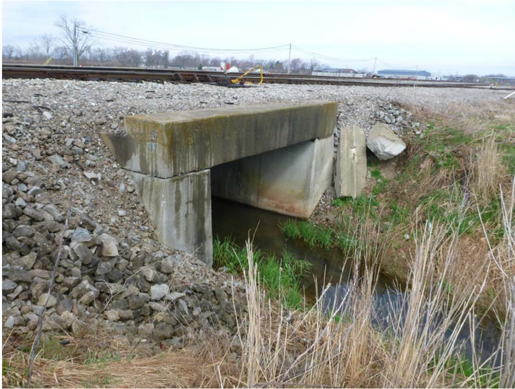
Photo 9. WOUS-4. Channel conveyed under L&I Line. Orientation northwest.
