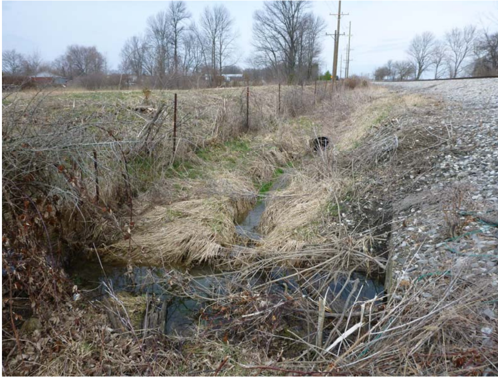
Photo 7. WOUS-3. Ephemeral channel conveyed under L&I Line, drains to the west into a human-made impoundment. Orientation northwest.
