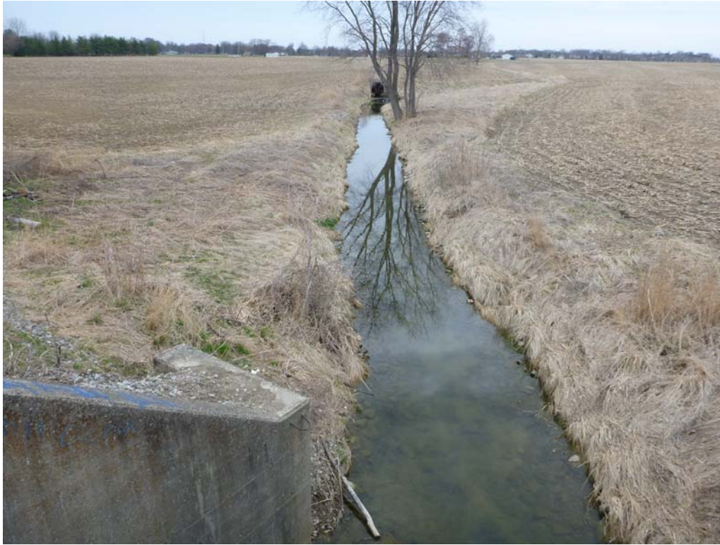
Photo 1. WOUS-1. Unnamed tributary of Young's Creek that is conveyed under L&I Line through a large concrete structure. Orientation northeast (upstream).
