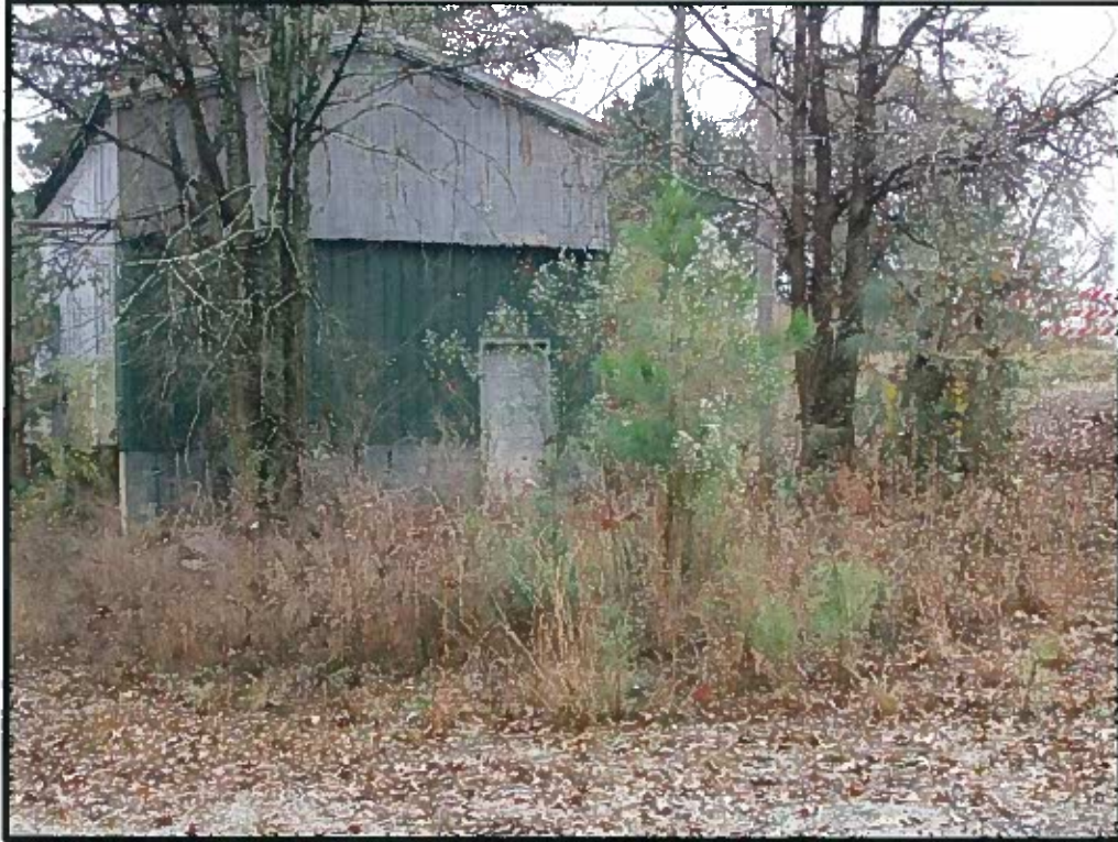
Photograph No. 3: Western façade of the smaller Century Granite Company Building.
