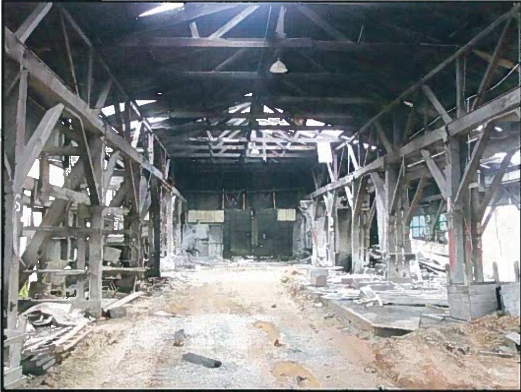
Photograph No. 1: Interior view of the main Century Granite Company Building, facing east.
