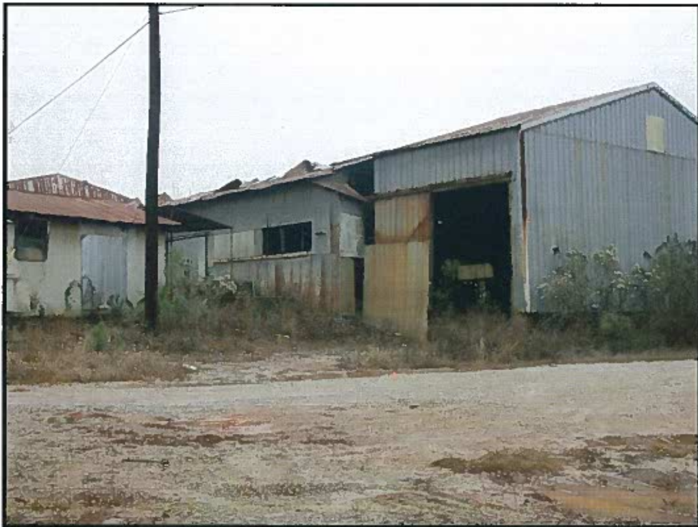
Photograph No. 4: Exterior view of the main Century Granite Company Building and Shed.
