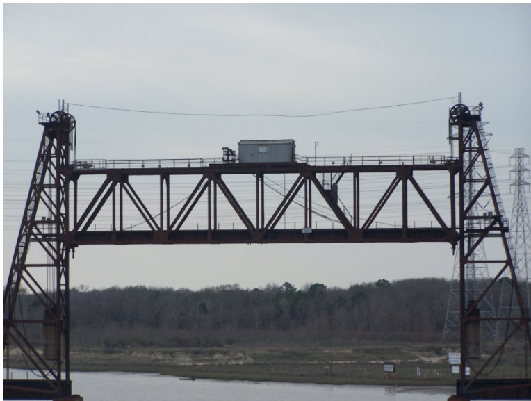
Figure 4. Cedar Bayou Bridge, Looking South
