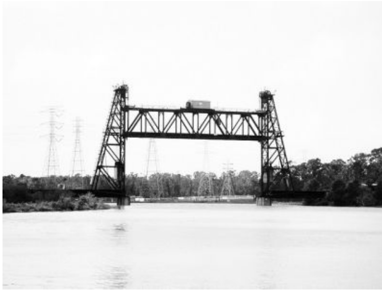
Figure 3. Cedar Bayou Bridge, Looking South
