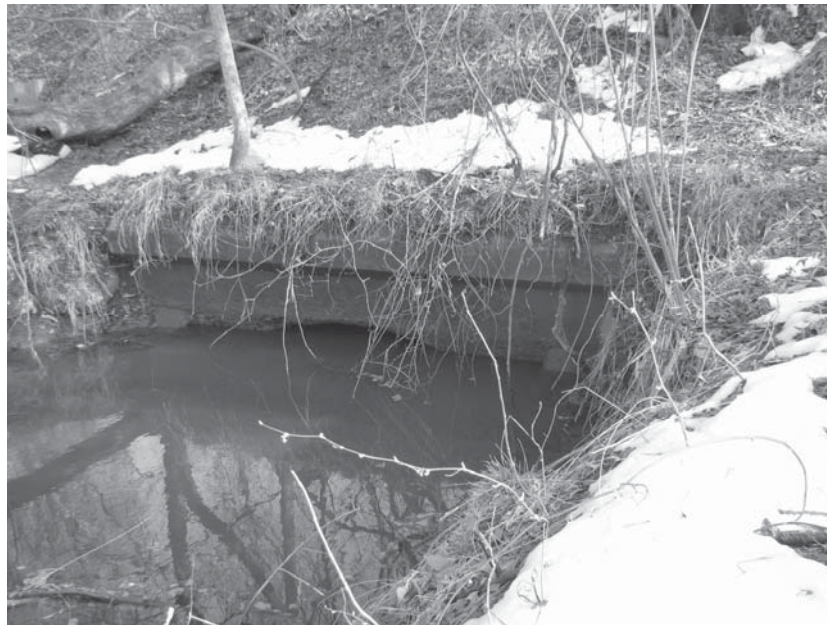
Looking upstream (north) at south end of culvert #980.
