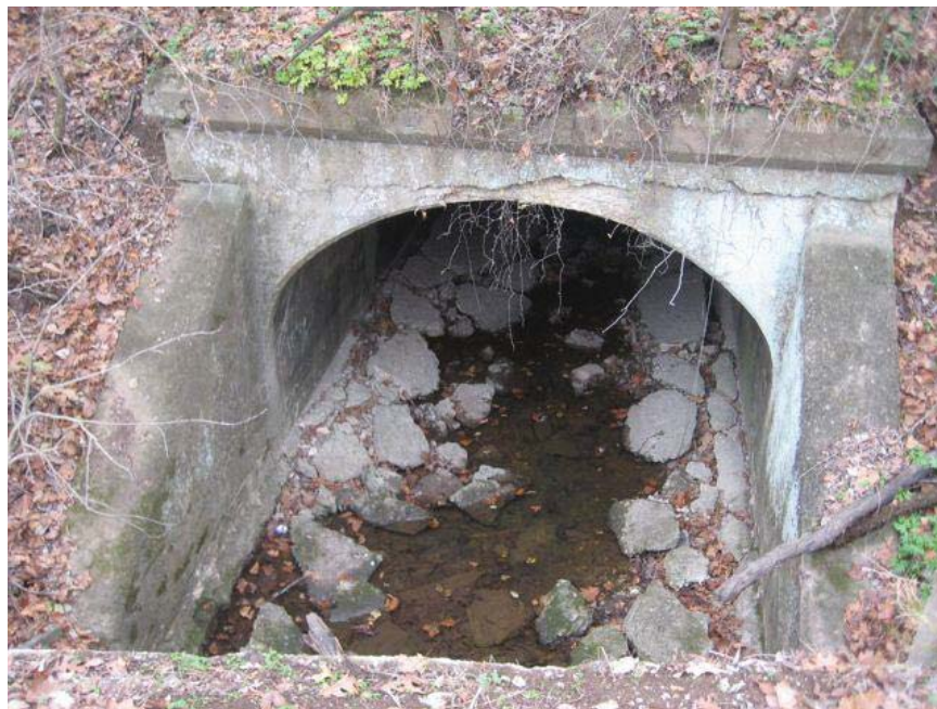
Looking downstream (south) from County Road at north end of culvert #1053.
