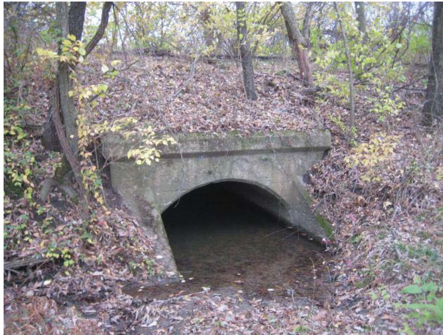
Looking downstream (south) at north end of culvert #1049.
