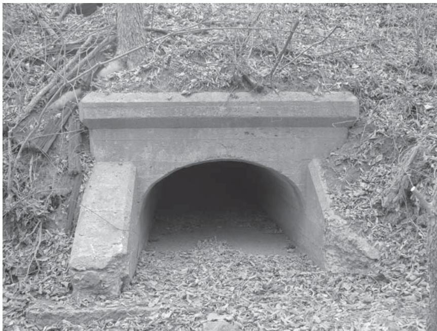
Photo 0033.jpg. North face of culvert #2047.
