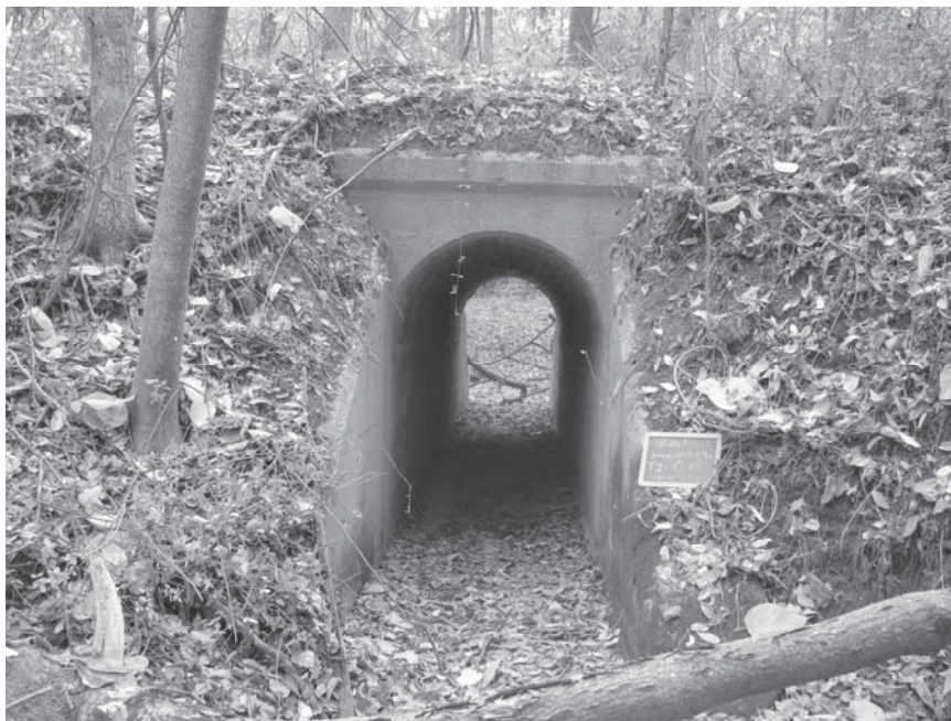
Photo 0019.jpg. North face of culvert #2128
