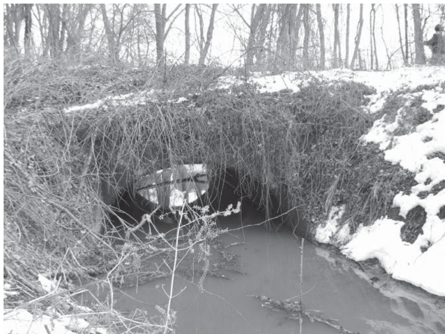
Looking upstream (east) at west end of culvert #990.
