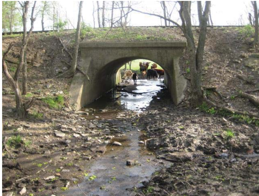
Looking upstream (north) at south end of culvert #2008.
