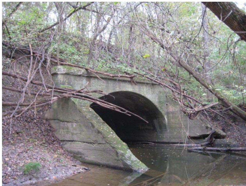
Looking southwest at northeast wing of culvert #2055.
