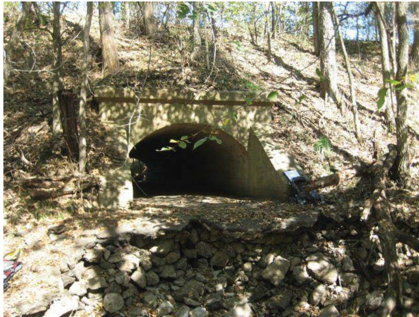
Looking upstream (north) at south end of culvert #2029.
