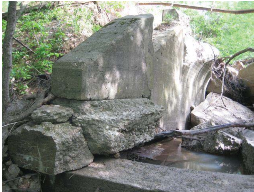
Looking north at culvert #2018.
