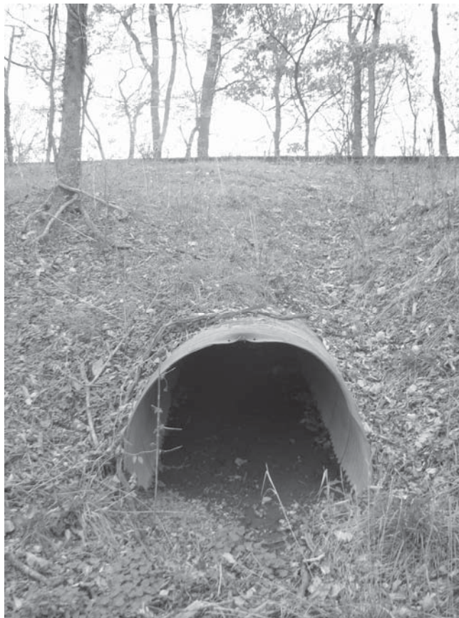
C 1060.jpg. North face of culvert #1060.
