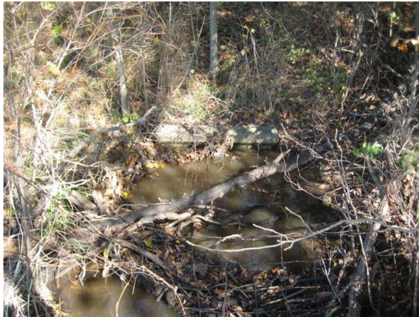
IMG_4747.jpg. South face of culvert #1128.
