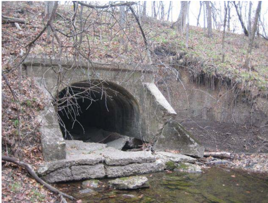
Looking upstream (north) of culvert #1053.
