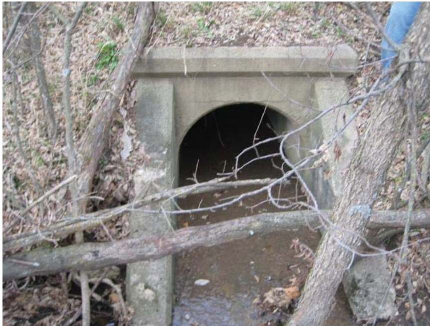
IMG_4800.jpg. South face of culvert #1144.
