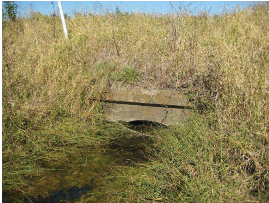
Looking upstream (north) at culvert #2039.
