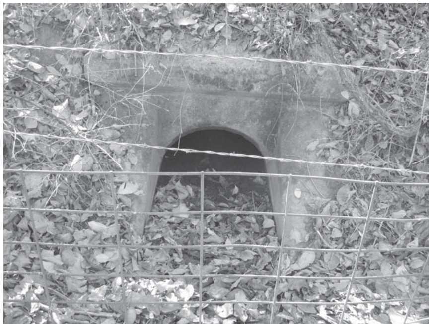
Photo 0053.jpg. North face of culvert #1128.
