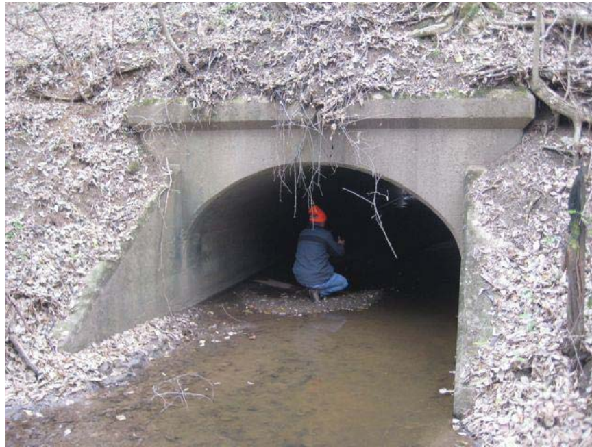
Looking upstream (south) at north end of culvert #1099.
