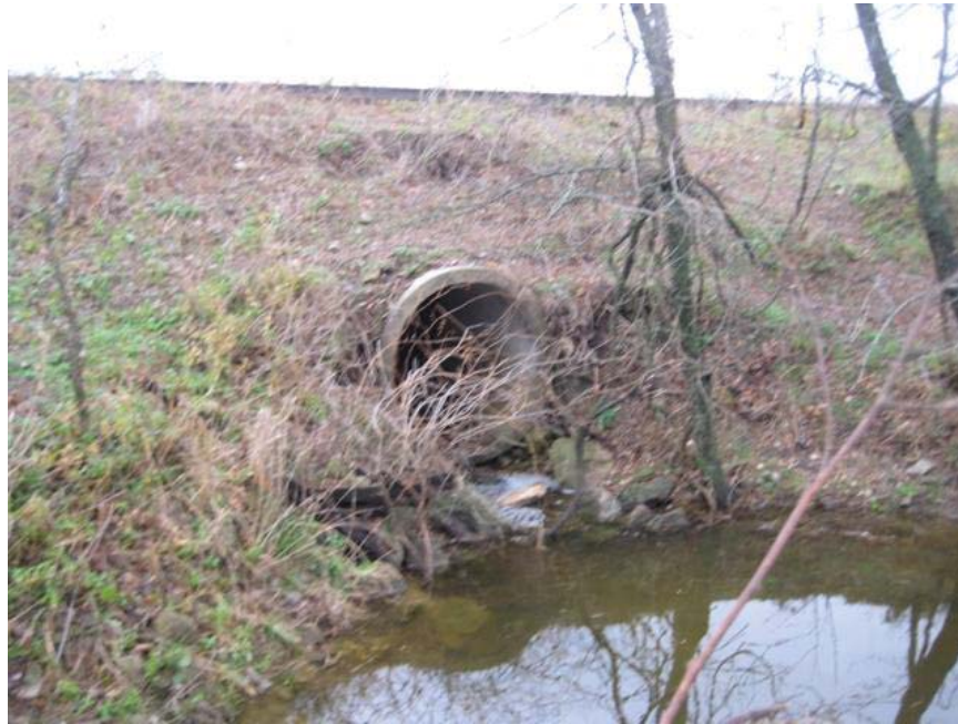
Picture 644.jpg. Culvert #2021.
