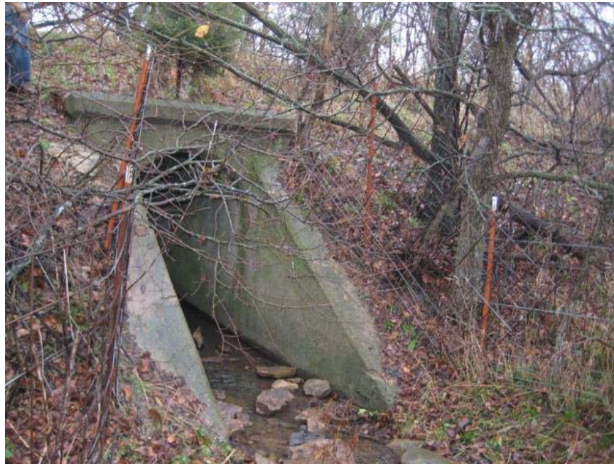
Picture 558.jpg. South face of culvert #2003.
