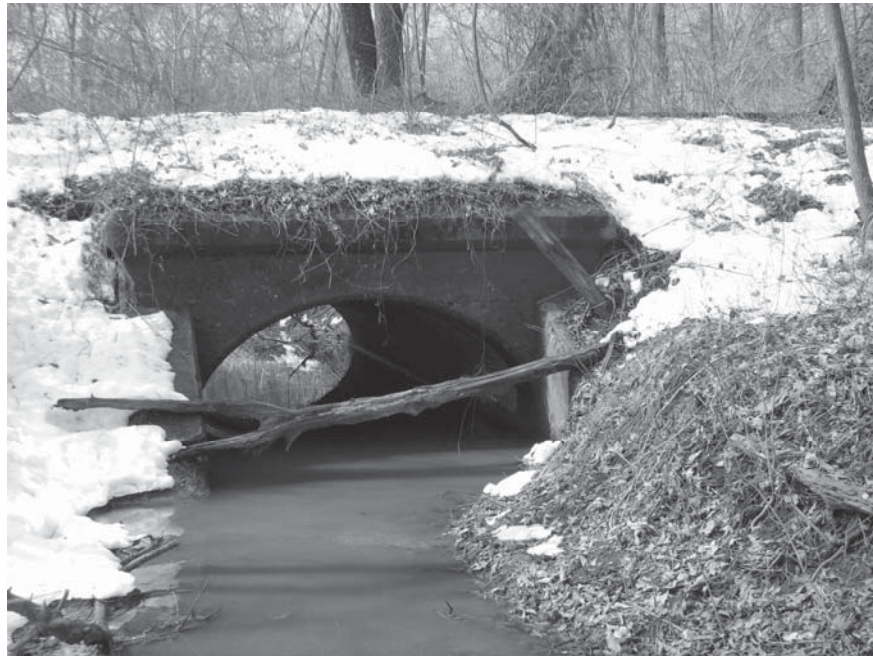
Looking downstream (west) at east end of culvert #990.
