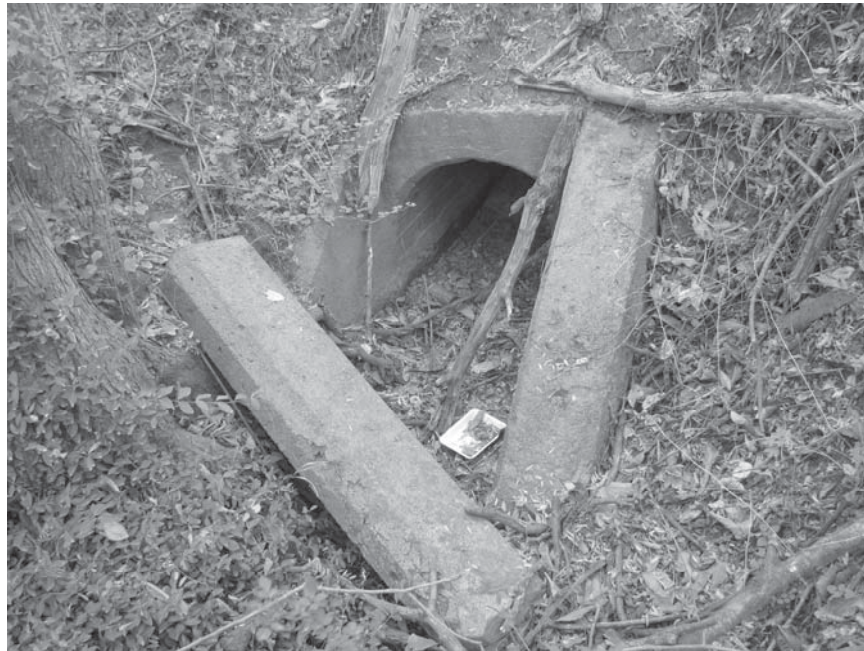
C 2095.jpg. Culvert #2095.
