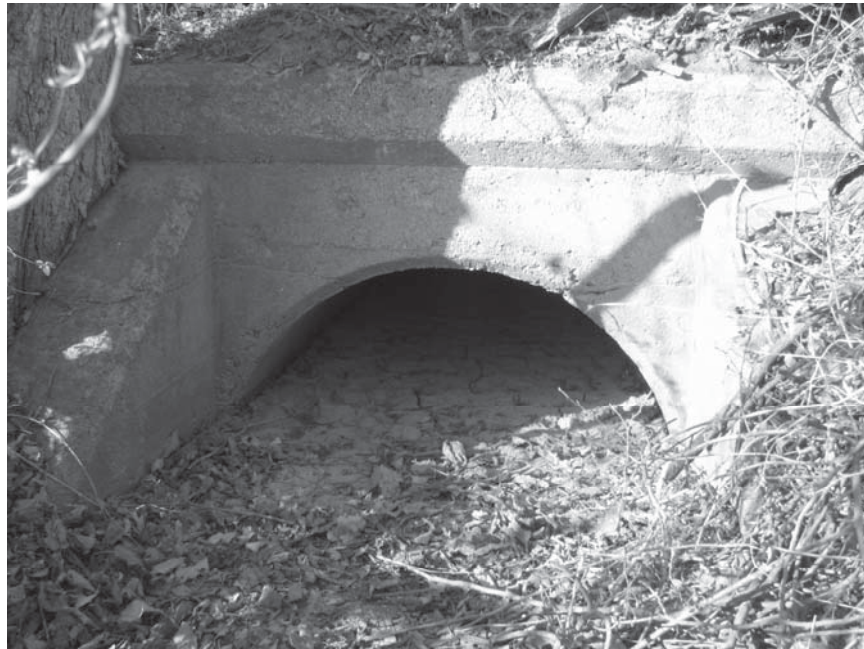
Photo 0056 C52 T2 1148.jpg. Culvert #1111.
