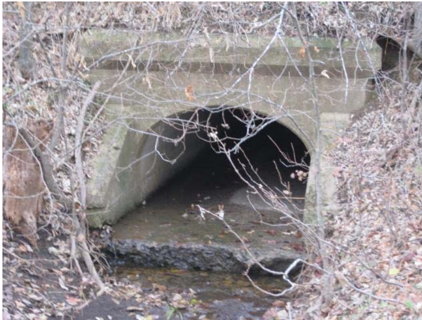
IMG_5139.jpg. South face of culvert #2047.
