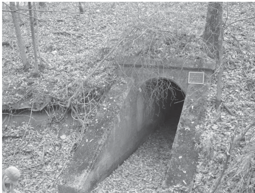
Photo 0023.jpg. North face of culvert #2111.
