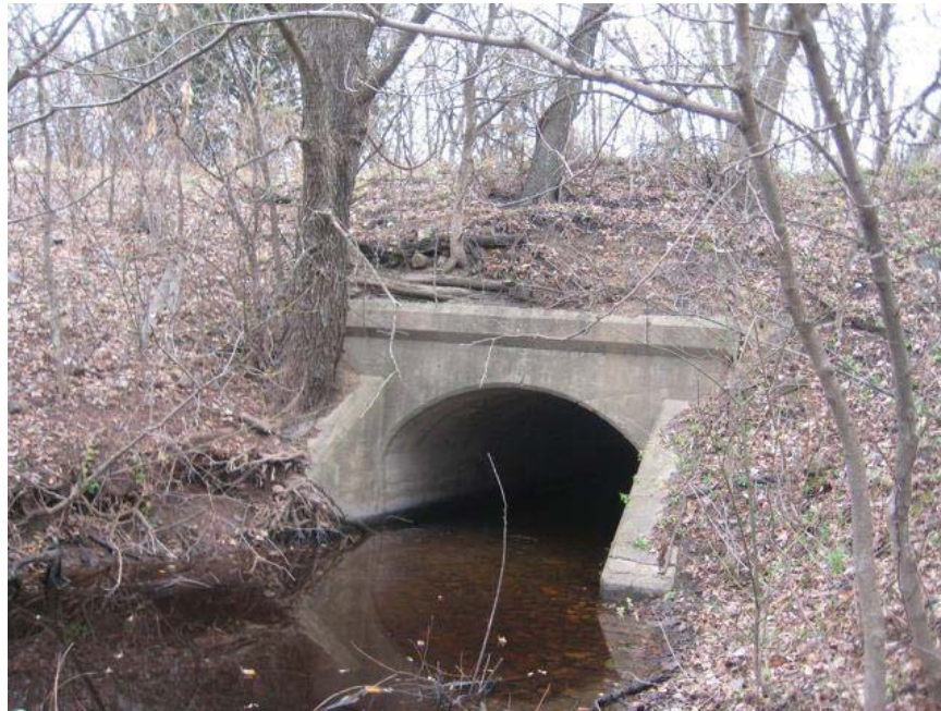
Looking upstream (north) at south end of culvert #1159.
