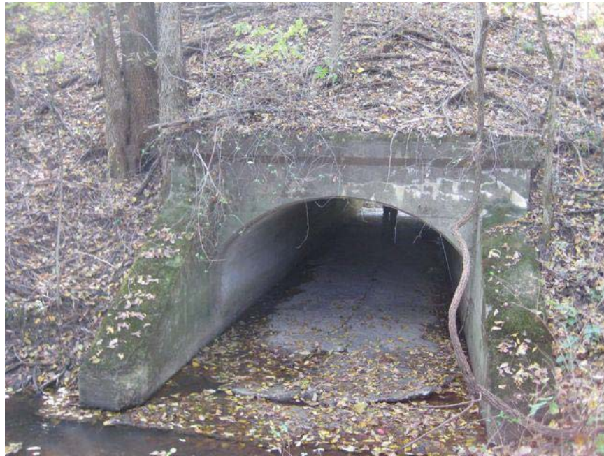
Looking downstream (south) at north end of culvert #2115.
