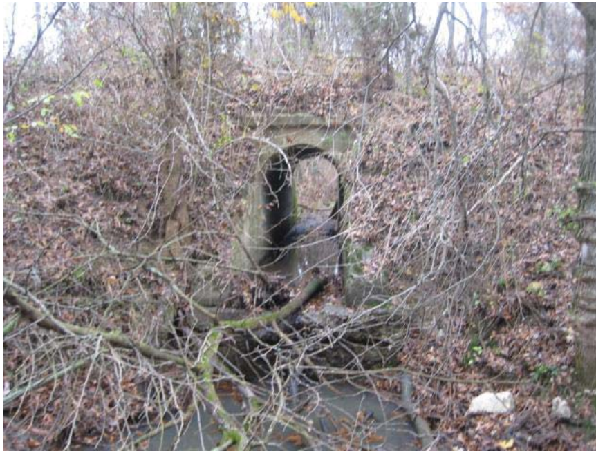
IMG_5591.jpg. South face of culvert #2128.
