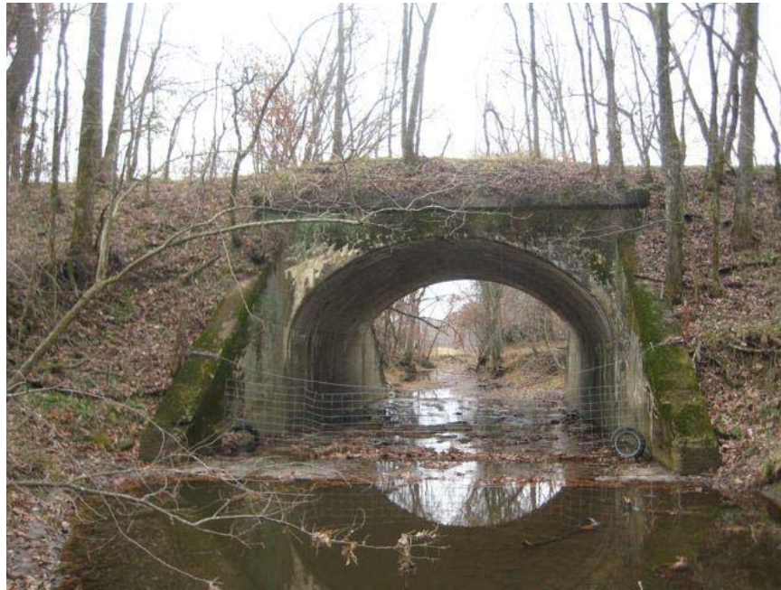
Looking downstream (south) at north end of very large culvert #1025.
