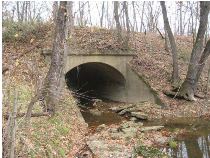
Looking upstream (northeast) at south end of culvert #1022.
