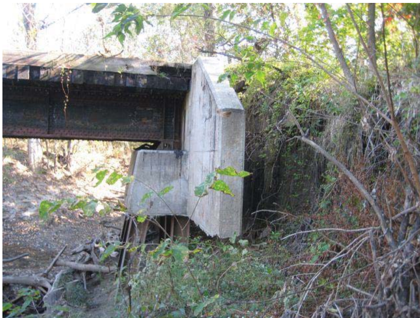
Looking north at east abutment of bridge #3031.
