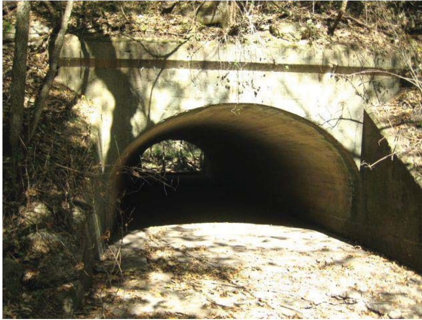
Looking upstream (north) through culvert #2032.
