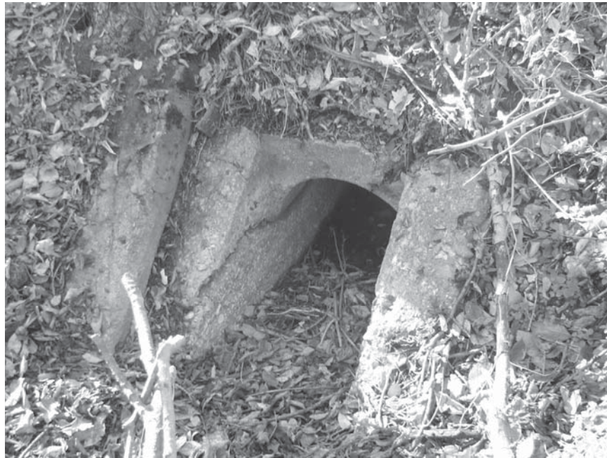
C 1047.jpg. Culvert #1047.
