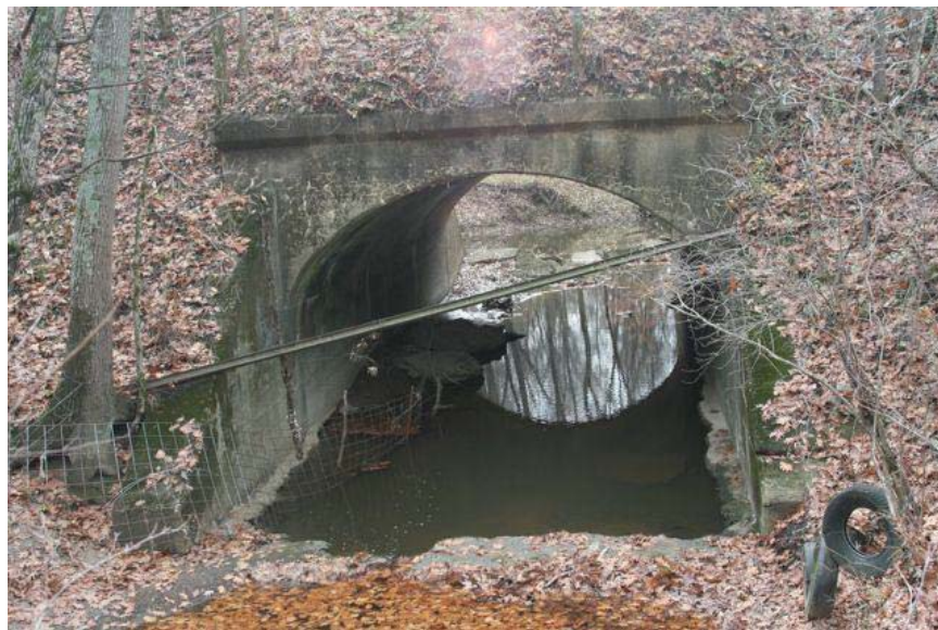
Looking downstream (south) at north end of culvert #1022.
