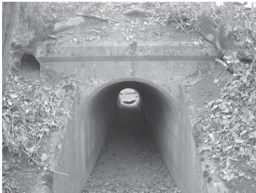
C 1162.jpg. North face of culvert #1162.
