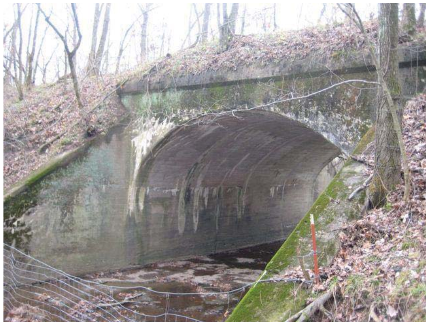
Looking southeast across north end of culvert #1025.
