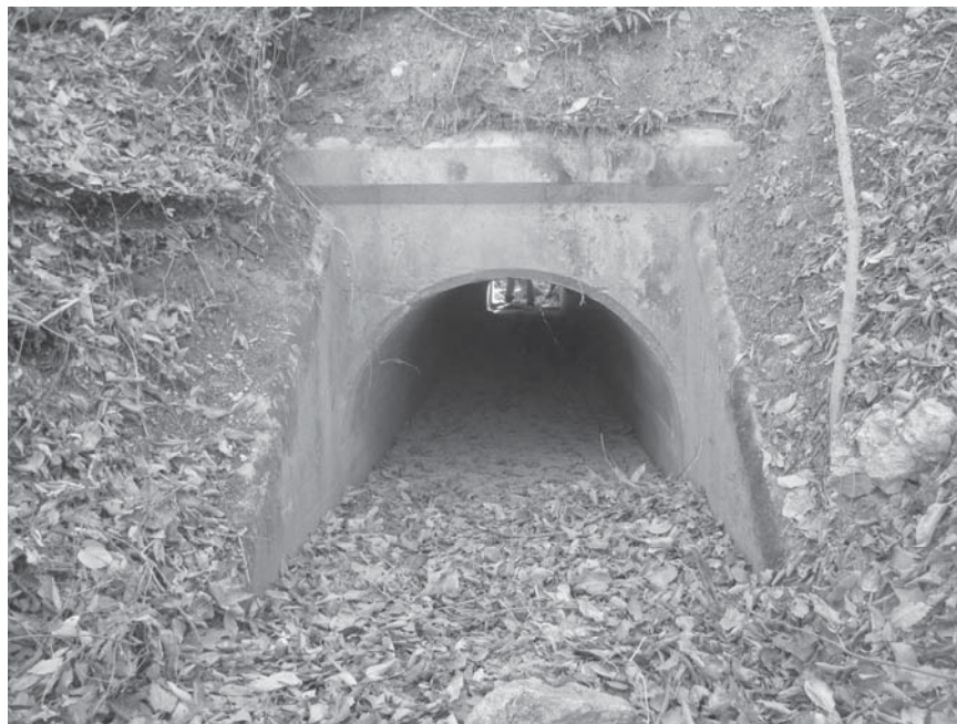
Photo 0044.jpg. North face of culvert #1150.
