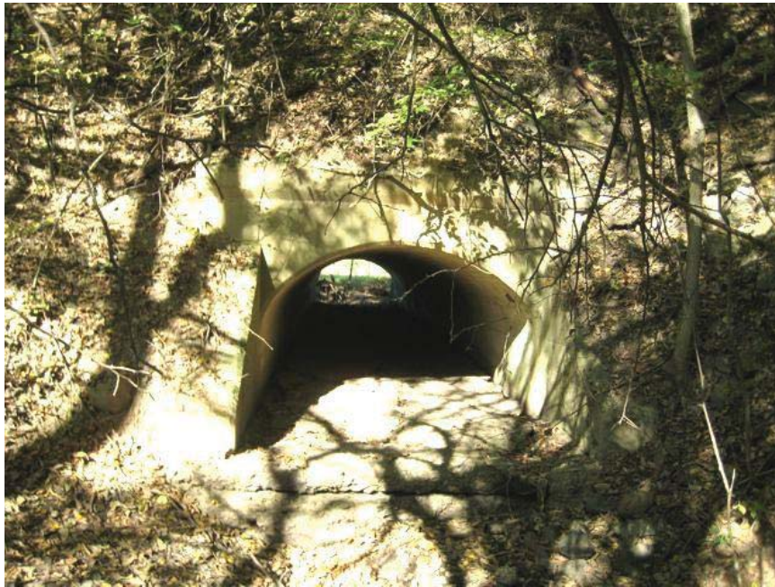
Looking north at south end of culvert #2023.
