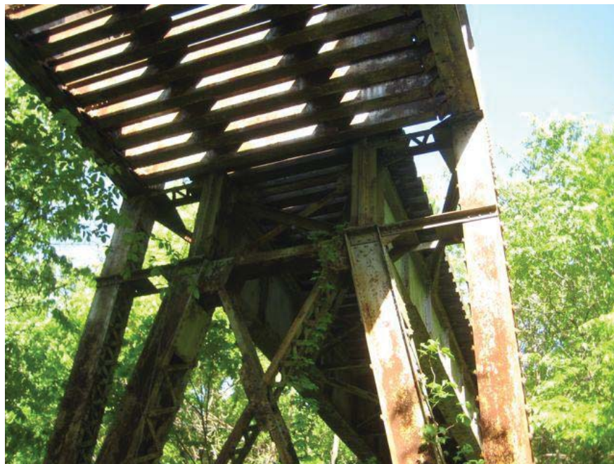
Looking northeast at west intermediate pier at west end of center span of bridge #2141.
