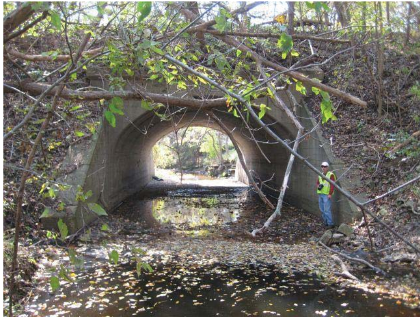
Looking upstream (north) at taller culvert #2122.
