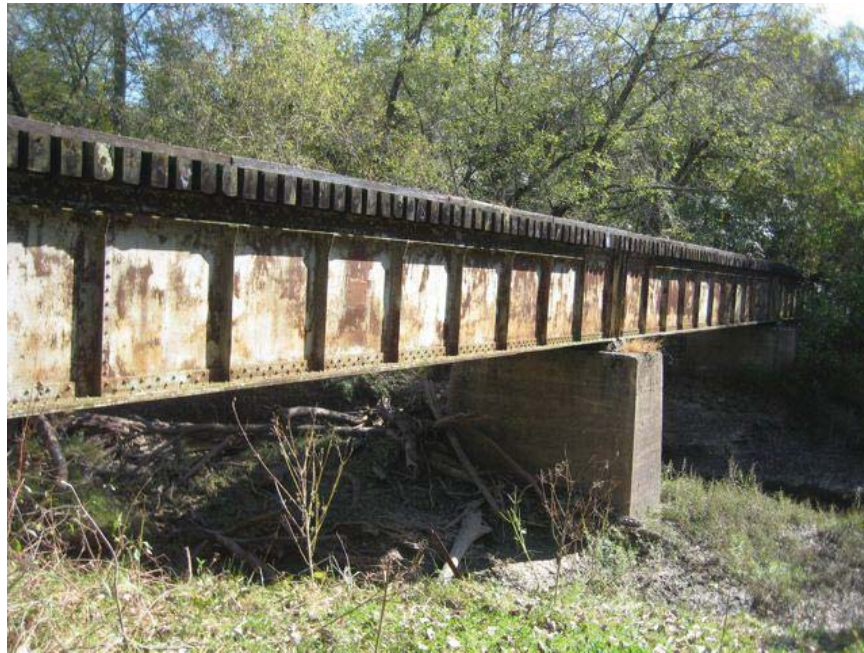
Looking northeast at three-span bridge #3042.
