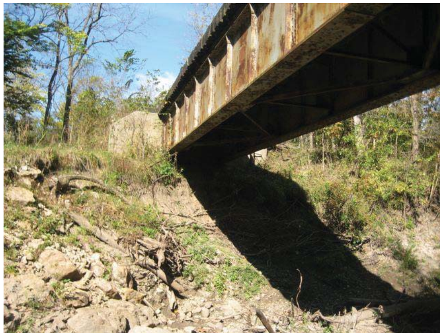
Looking west along bridge at west abutment of bridge #3042.
