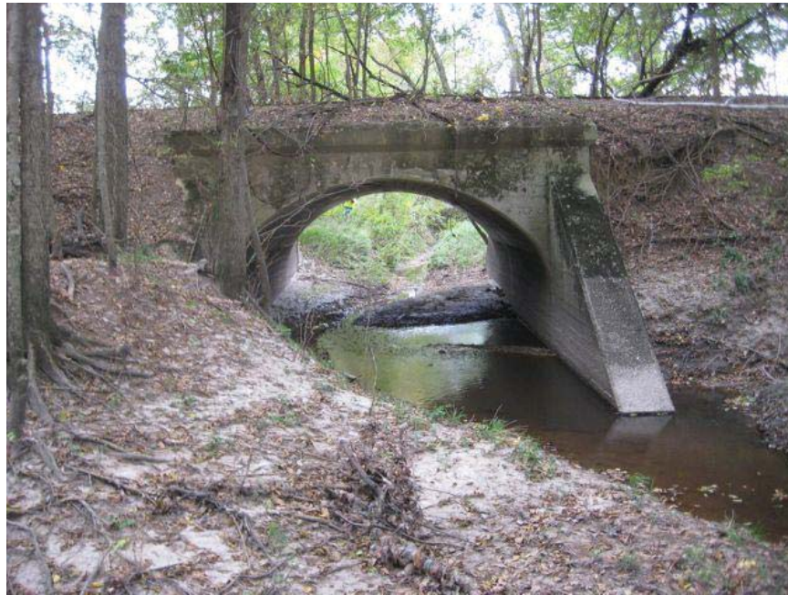
Looking downstream (south) at north culvert face of culvert #3000.
