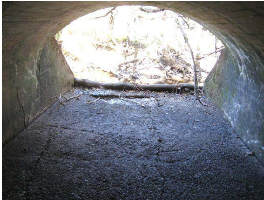
Looking upstream (north) from culvert #2032.
