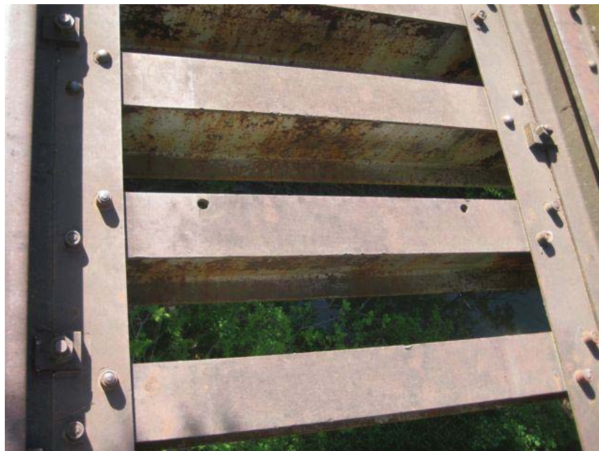
Looking down at steel stringers in center span between through-girders of bridge #2141.
