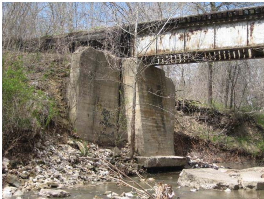
Looking northwest at west intermediate pier between center girder span and west end timber span of bridge #2152.
