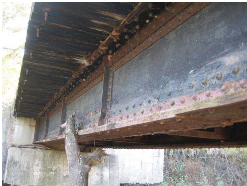
Looking southeast along north side of east end span of bridge #3031. Note typical built-up plate girder riveted construction.
