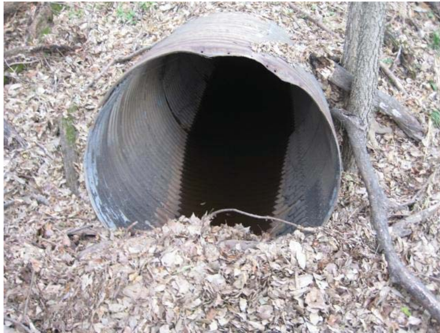
IMG_4855.jpg. South face of culvert #1162.
