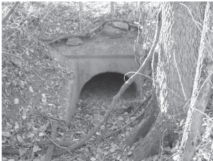
Photo 0046.jpg. North face of culvert #1145.
