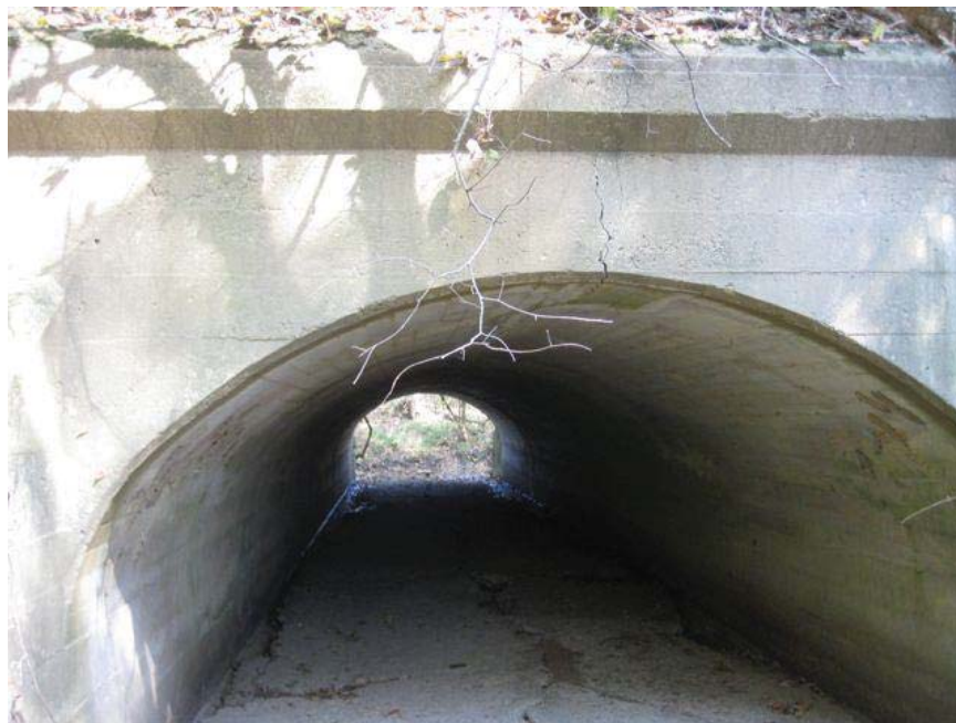
South headwall of culvert #2115.
