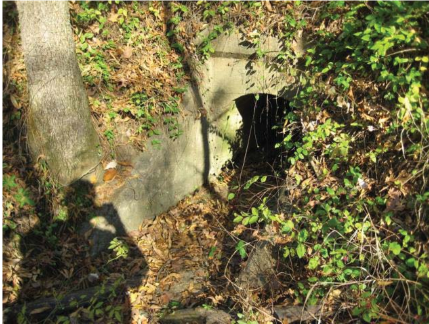
IMG_4385.jpg. South face of culvert #1019.
