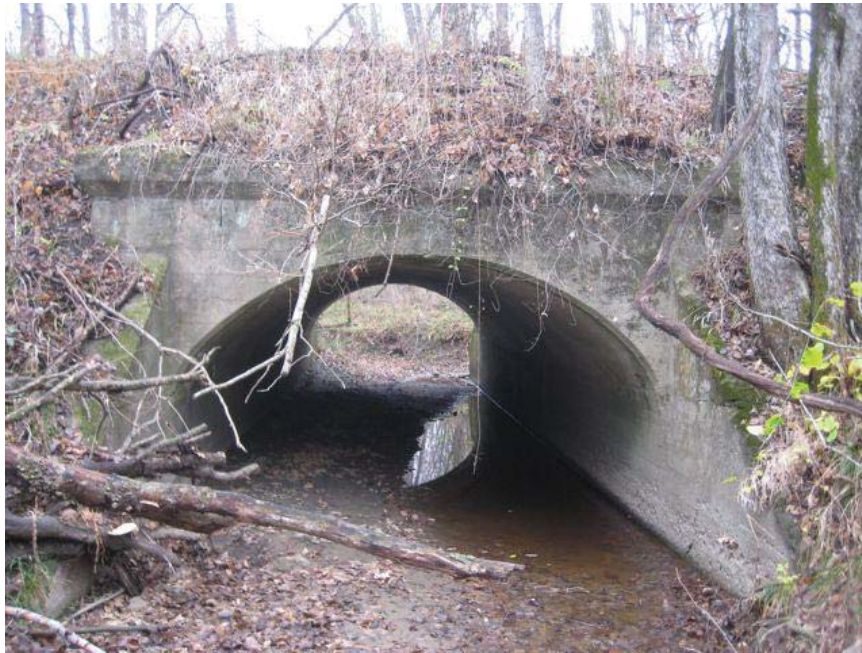
Looking upstream (north) at south end of culvert #1033.
