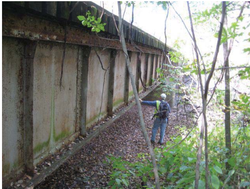
Looking west along north side of east end span from east abutment of bridge #3042. Note lower ground clearance.
