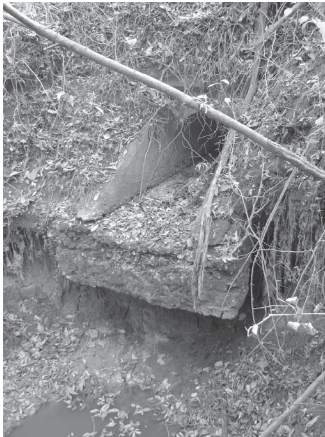
Photo 0074.jpg. North face of culvert #1019.
