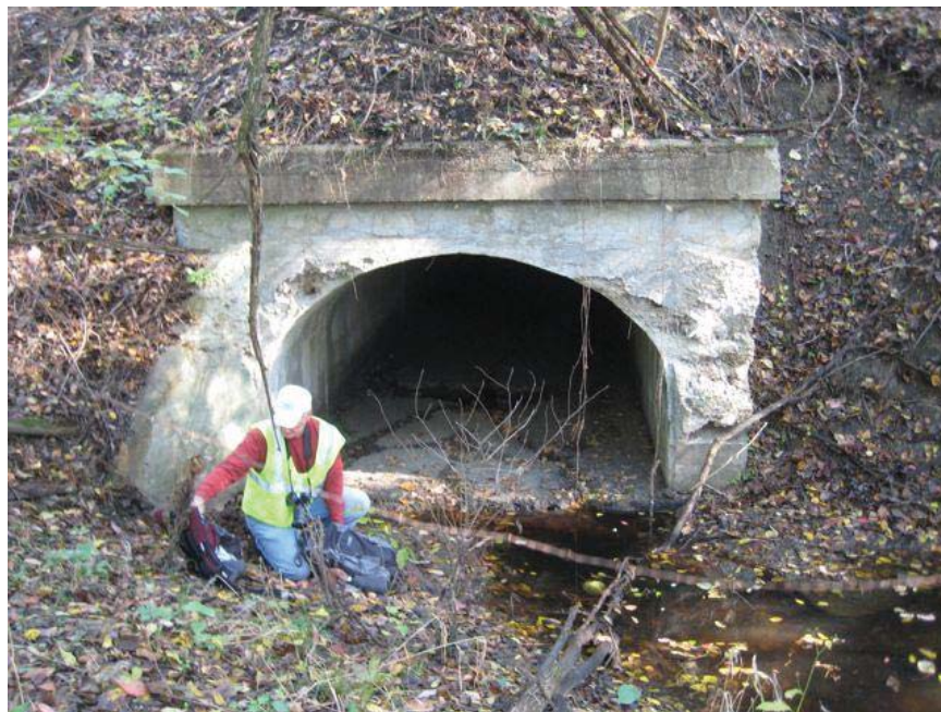
Looking downstream (north) at culvert #2087.
