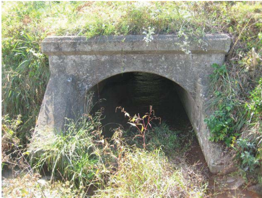
Looking downstream (south) at culvert #2042.
