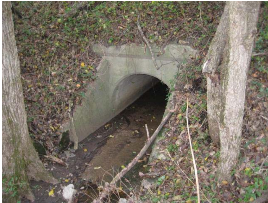
IMG_4821.jpg. South face of culvert #1150.
