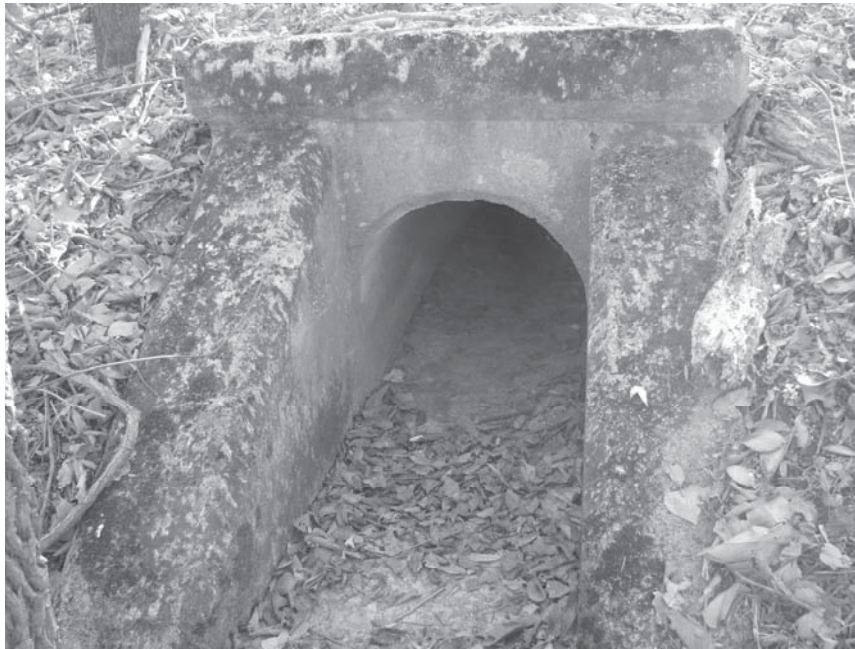
Photo 0055 C51 T2 1133.jpg. Culvert #1117.
