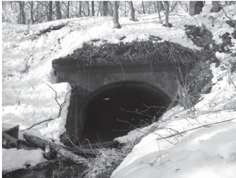
Looking downstream (south) at north end of culvert #980.
