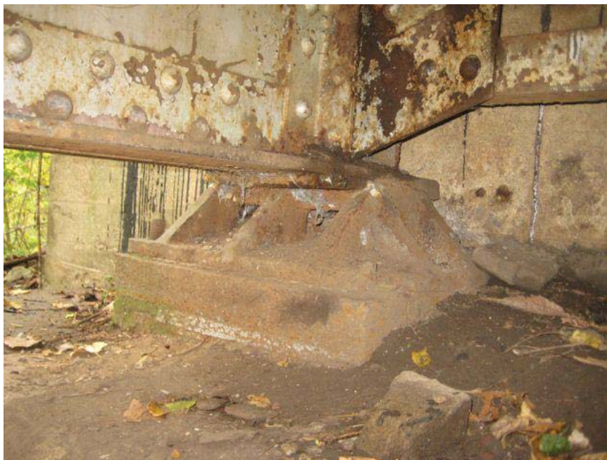
Typical girder end bearing at west abutment under south girder of bridge #2063.
