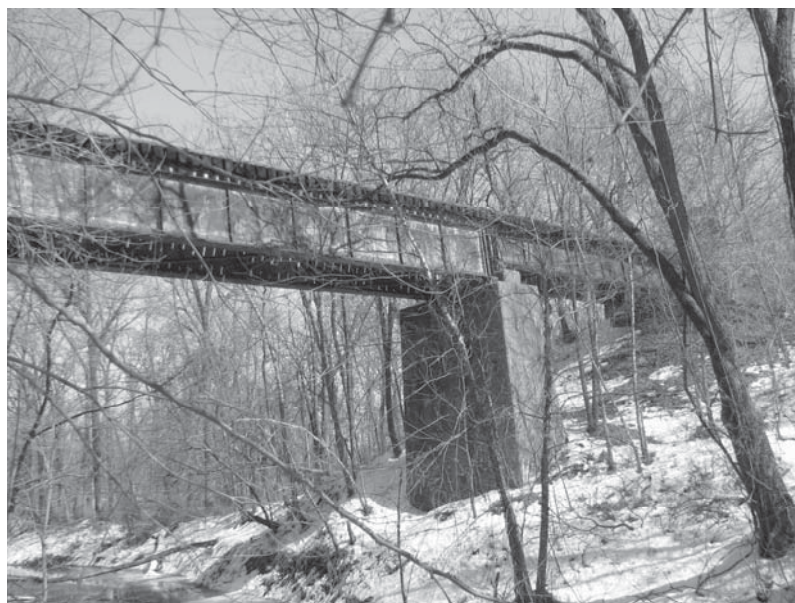
Looking along north face of bridge #960.
