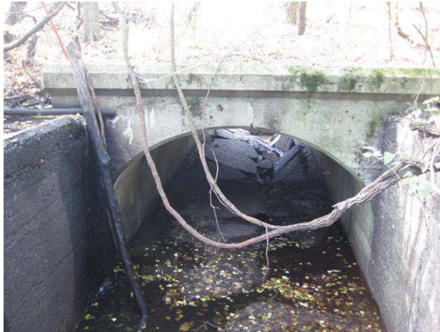
Looking south through culvert #2104 across intake chamber.
