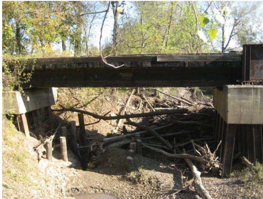
Looking north at west end span of four-span bridge #3031.
