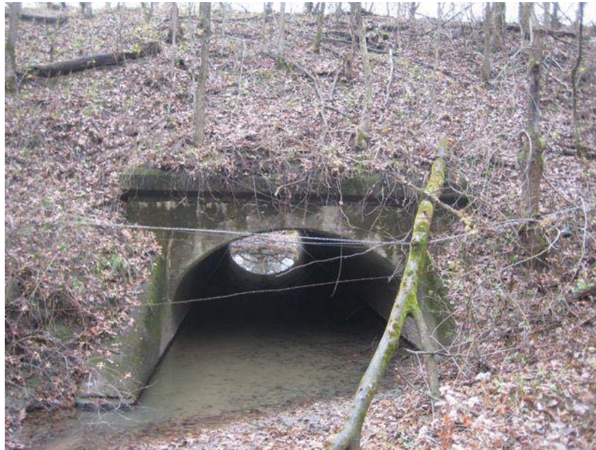
Looking downstream (south) at north end of culvert #1028.
