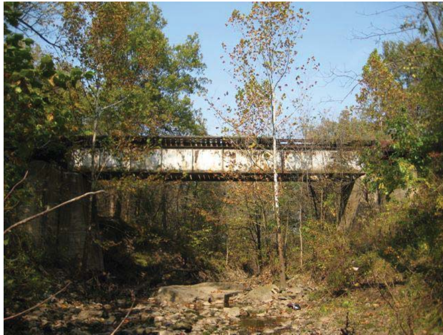
Looking upstream (north) at tall bridge #2152.
