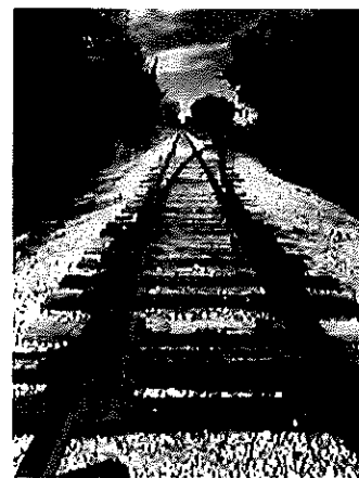
South Wye Turnout
