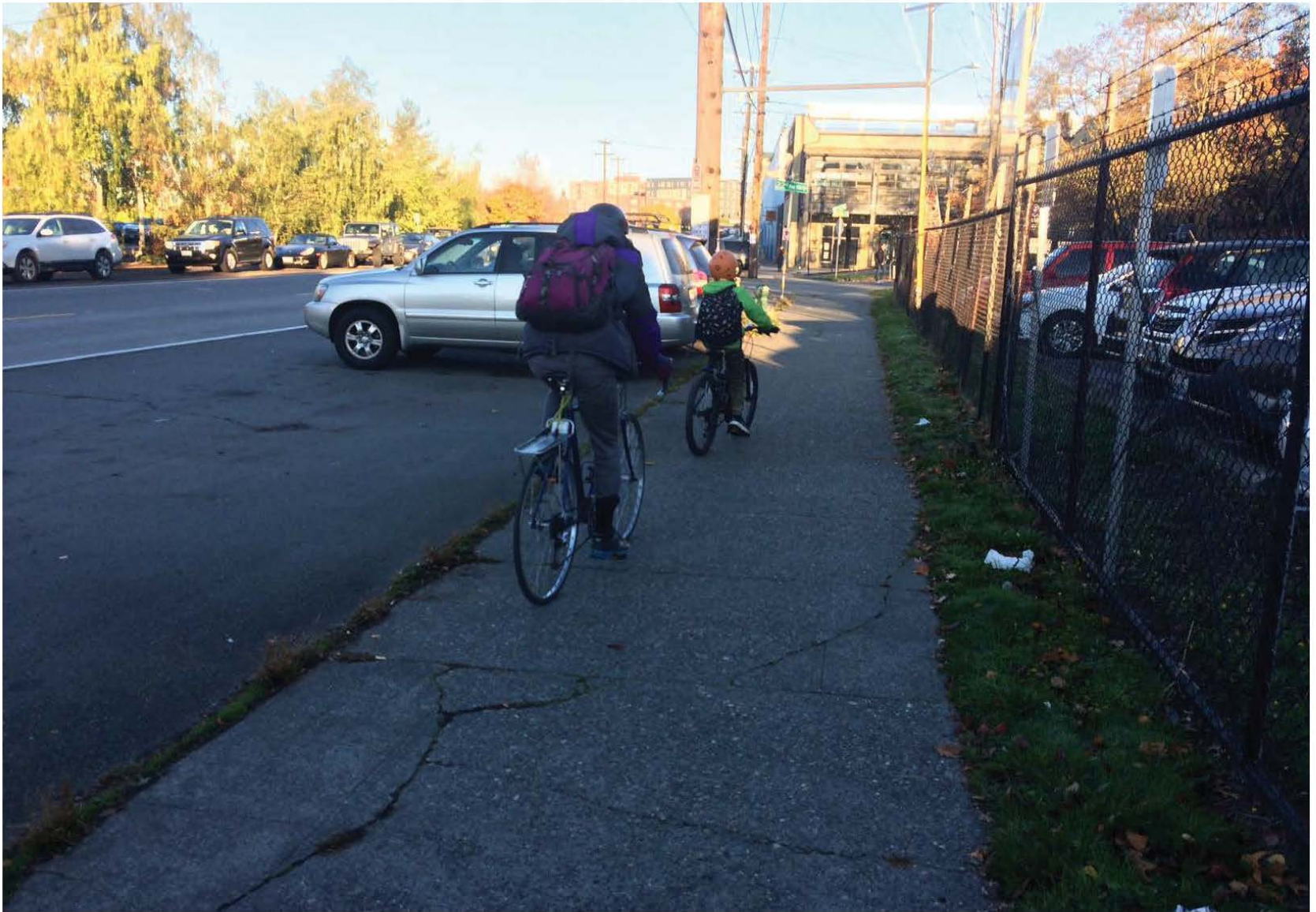
Location: NW 22 nd Ave & Shilshole Ave NW. Date: 10/27/17
