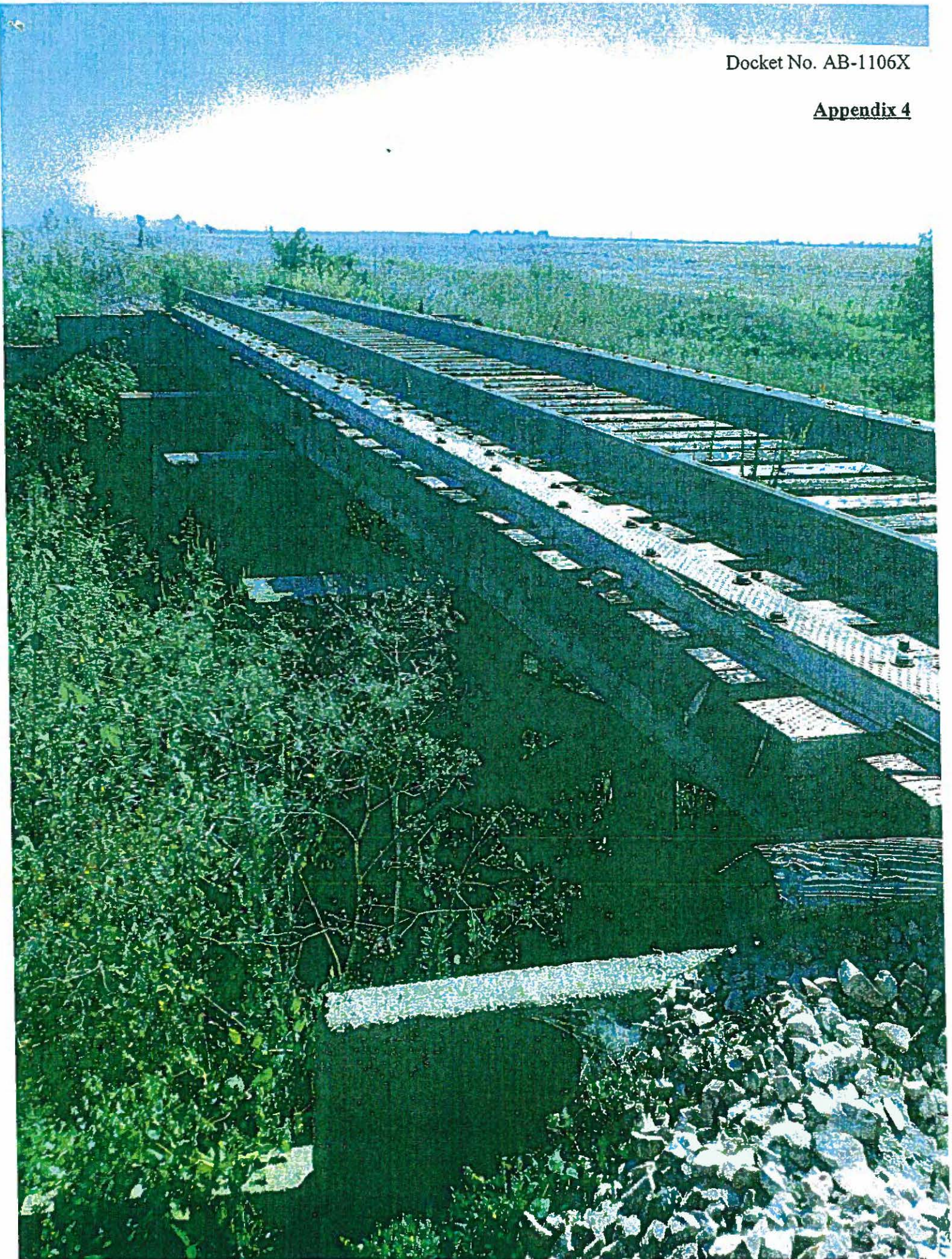
Bridge over Indian Creek in south half of rail line looking SSW
