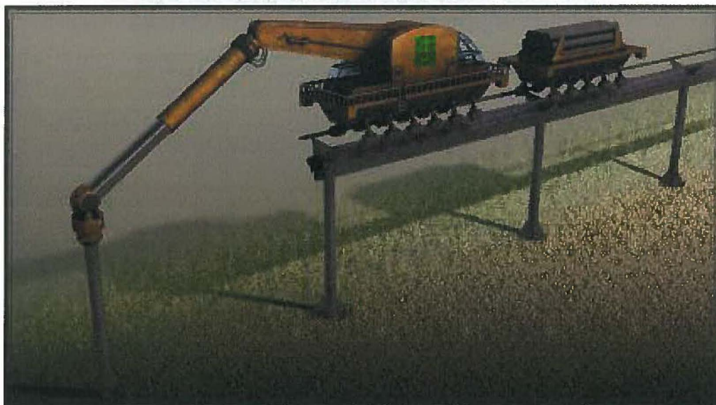
Figure 5 - Interstate Traveler - Integrated Installation Crane
