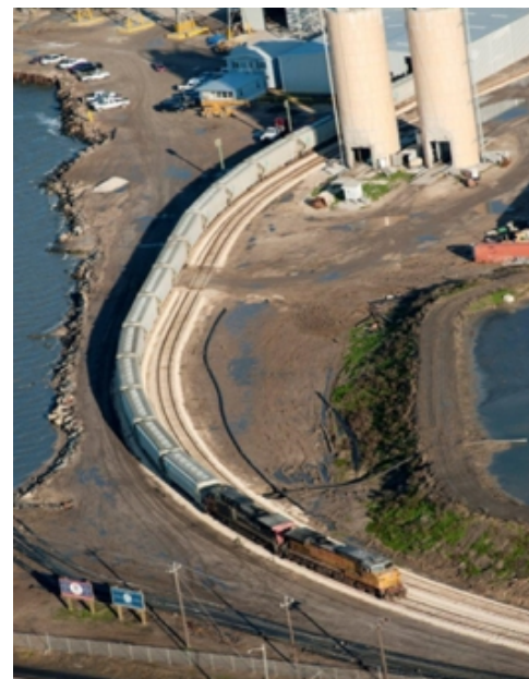
Soda Ash Export Terminal in Galveston, TX
