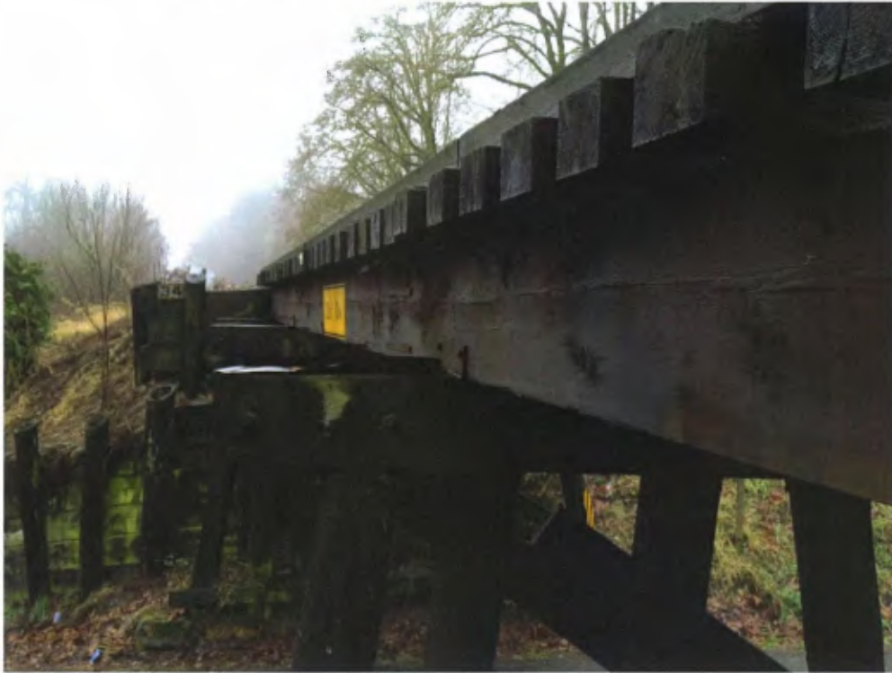
East Stringer Looking South from North Abutment
