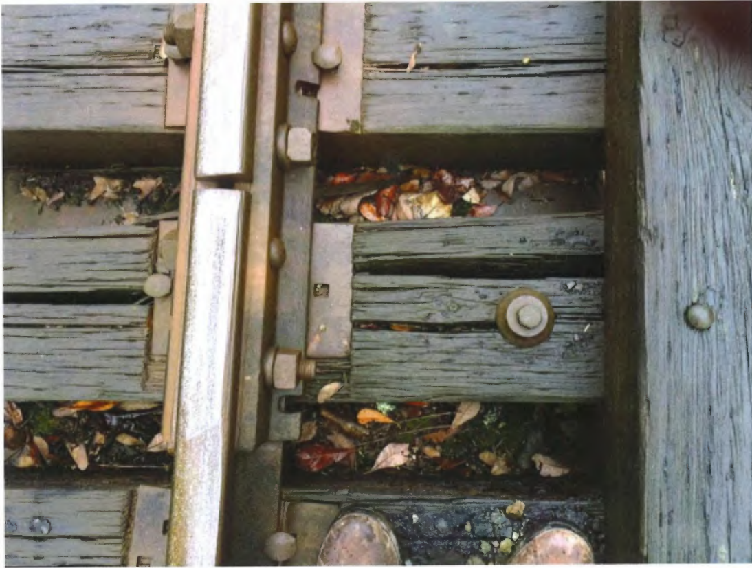
Multiple Deteriorated Ties at North Abutment Looking Southeast
