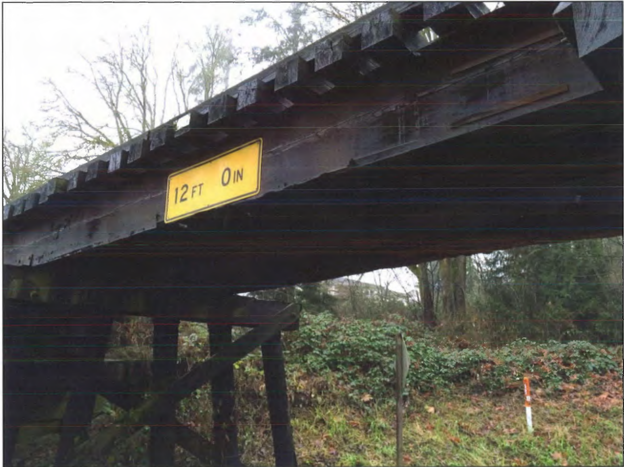
Span 2 Looking Southwest
