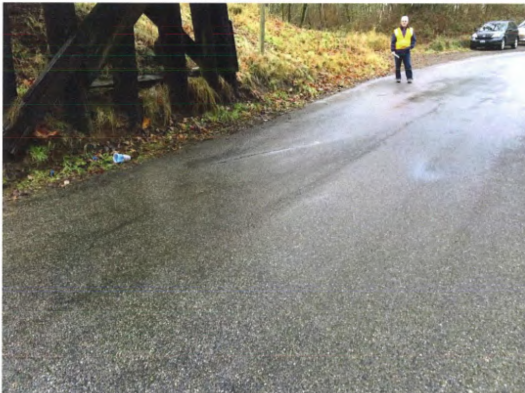
Utility Trench Settlement under Span 2 Looking West
