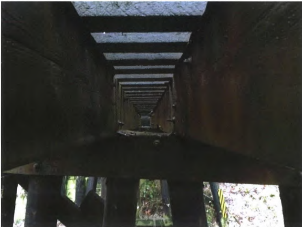
Looking South between East and West Stringers
