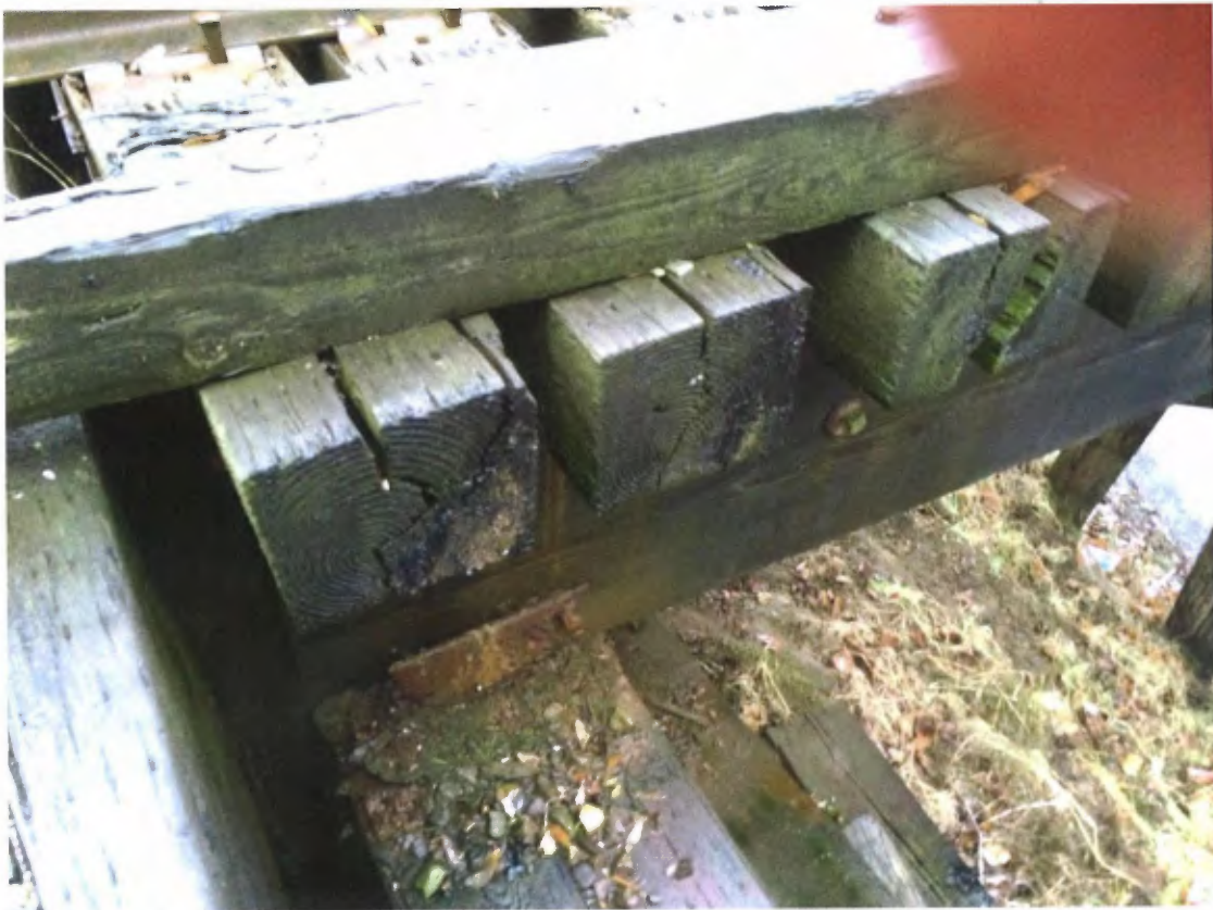
Multiple Deteriorated Ties at North Abutment Looking Southeast
