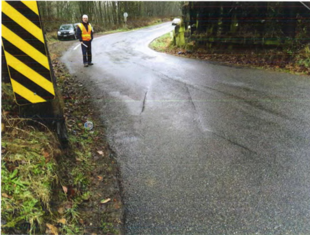
Utility Trench Settlement under Span 2 Looking West
