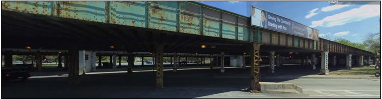
Existing Bridge at DC 27.45 42
