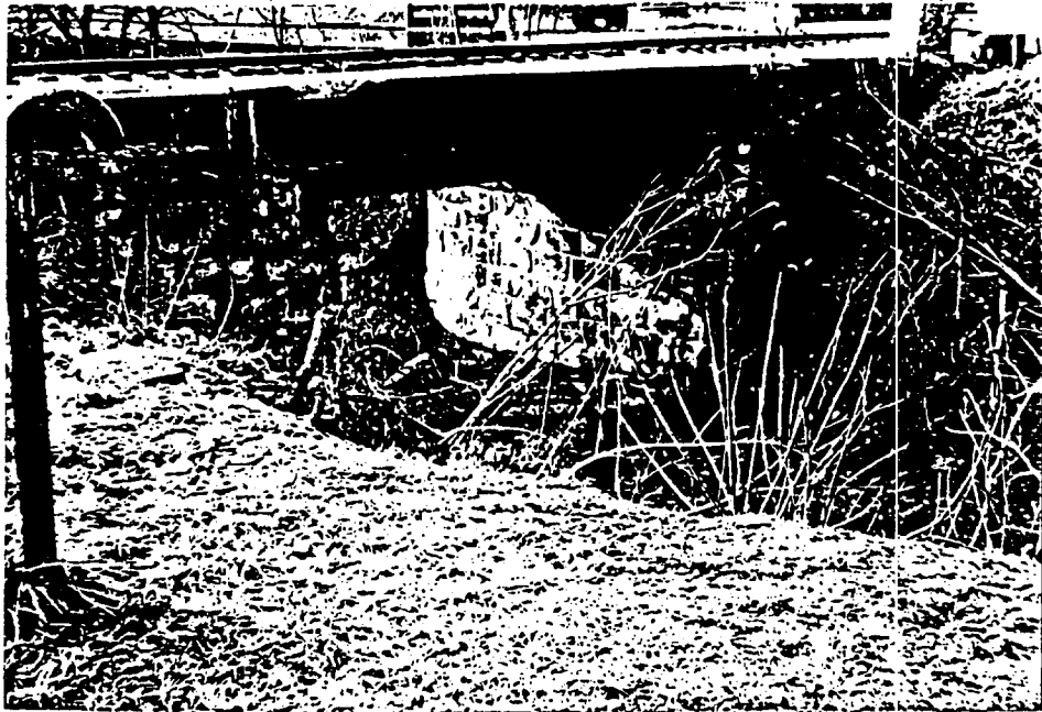
Bridge #115 Finck's Run Milepost 307.35 Barrackville, WV
