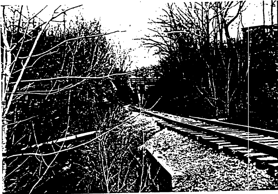
Bridge #118-3/4 Mahan Run Milepost 317.38 Rachel, WV
