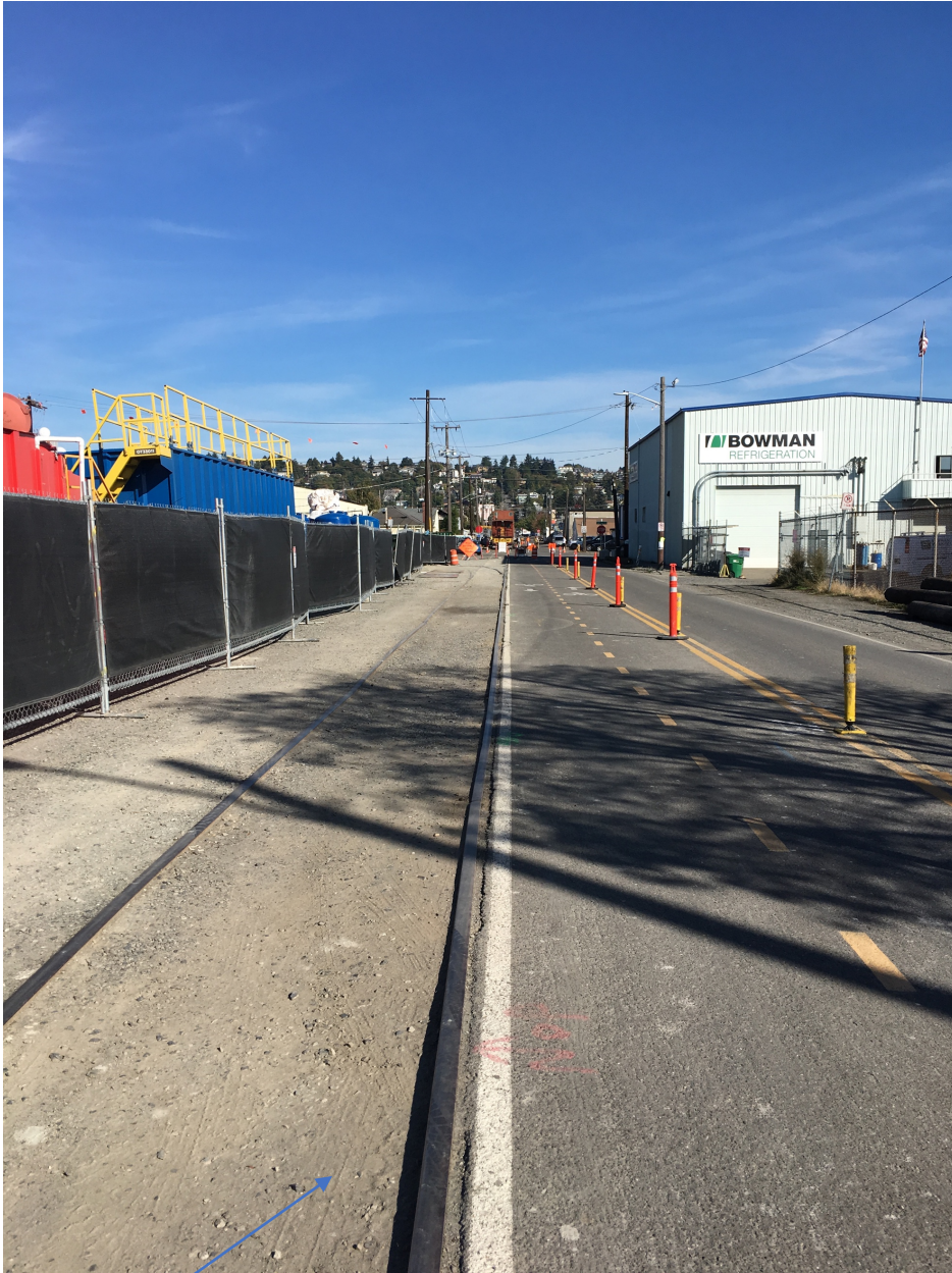
Looking east, BTRC mainline track as currently configured on NW 45 th Street in Seattle. 73
