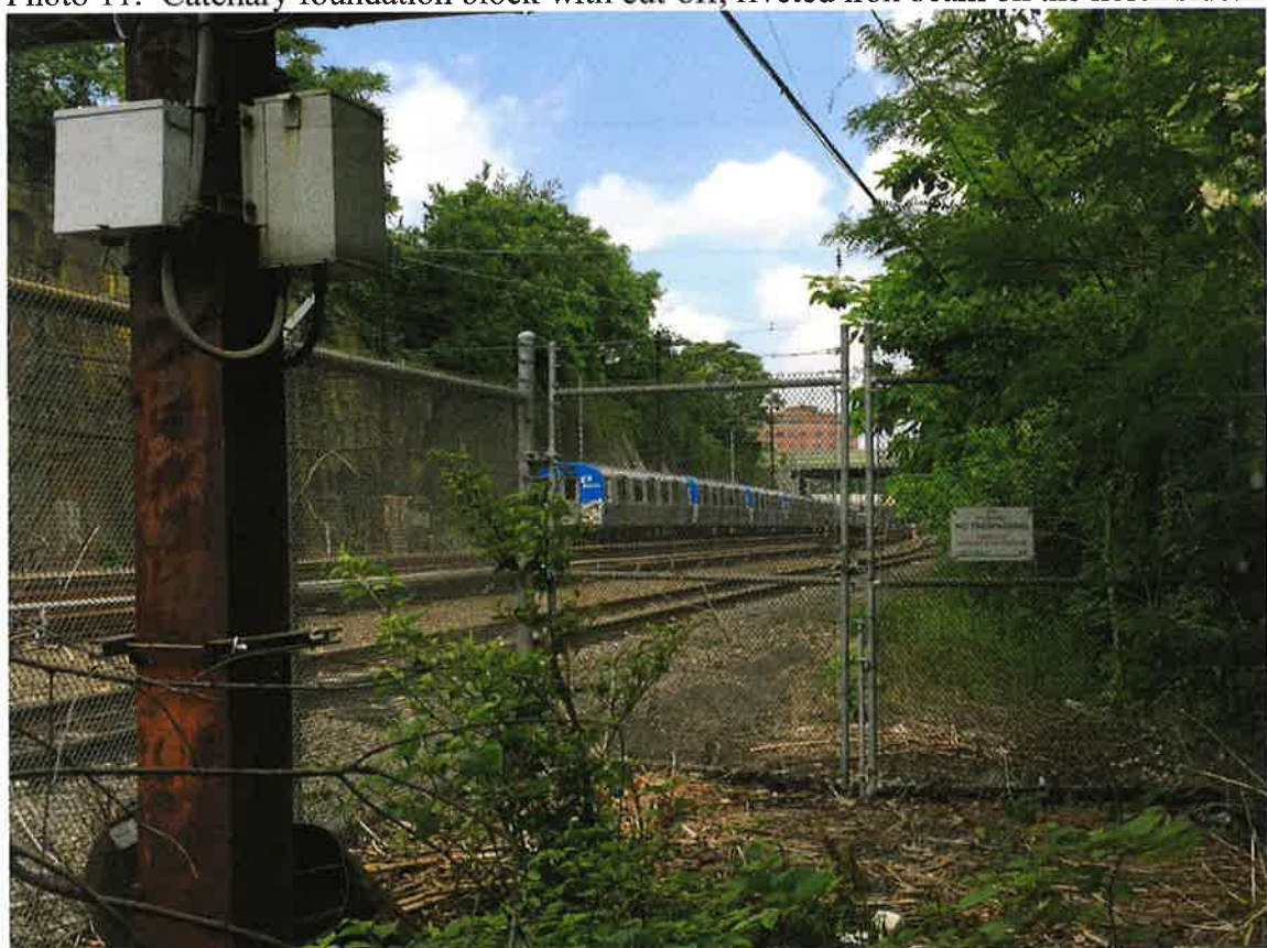
Photo 12. North side catenary pole with gate beyond showing junction of the Harsimus Branch with the main line.
