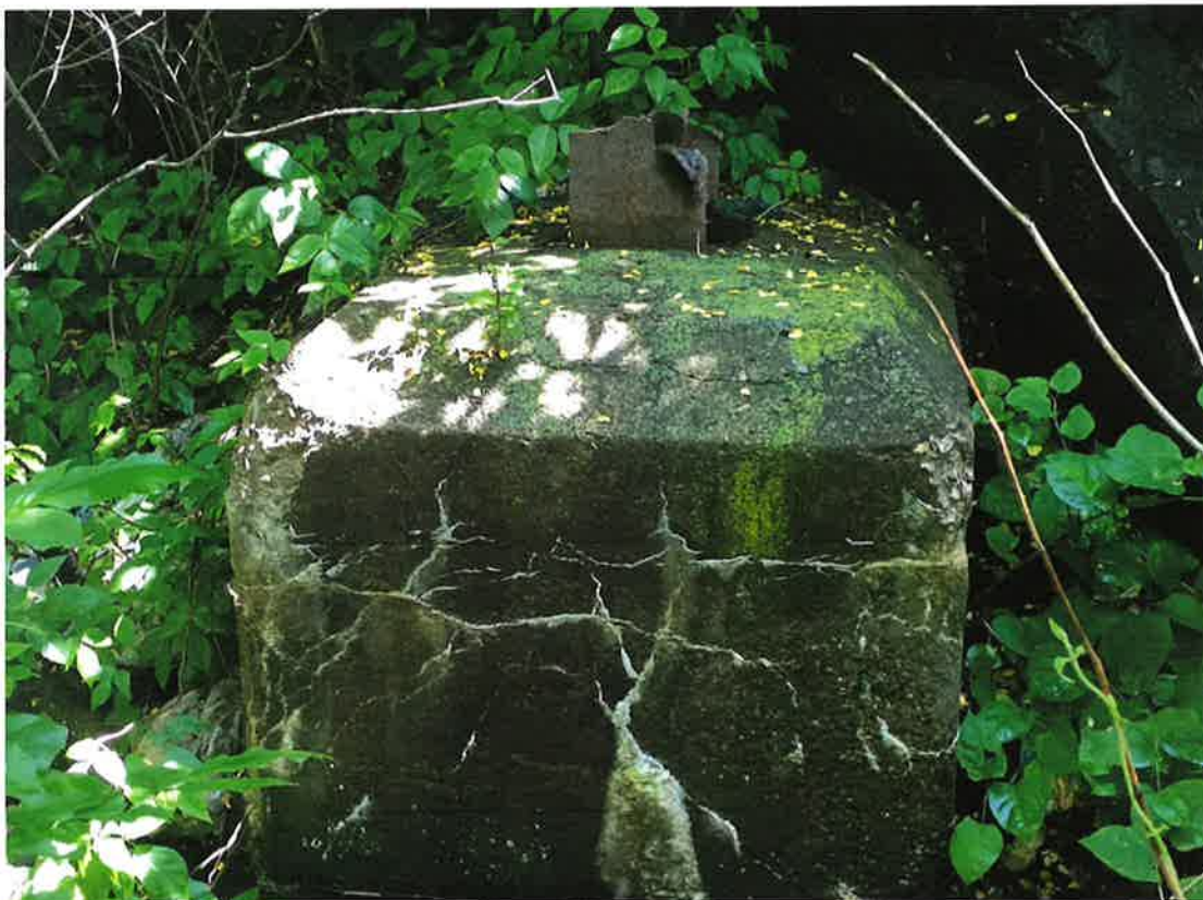
Photo 7. The fourth set of catenary foundation blocks, on the north side of the culvert.
