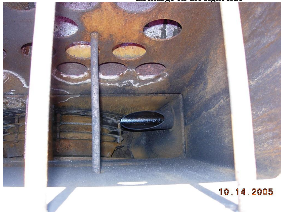
Figure 3: Inside of exhaust stack on Metrolink No. 804, showing the crankcase vent discharge on the right side
