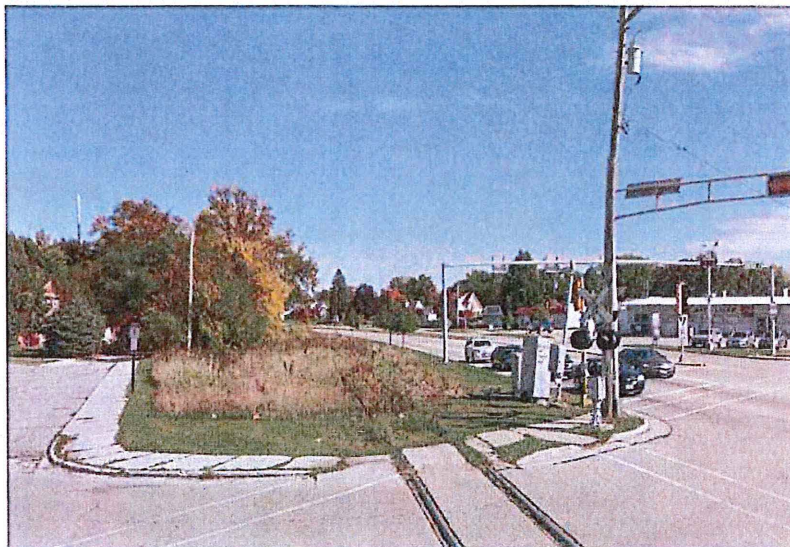
Photo 4. Rail Line at Union Avenue, Looking Northeast
