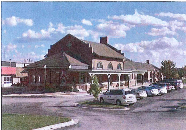
Photo 5. Chicago and North Western Depot (AHI No. 82541), Looking Southeast
