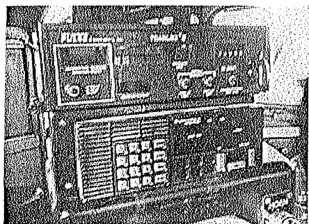
This picture depicts an electronic component referred to as the Head End Telemetry Device and is located on the console of the controlling locomotive of a train.
