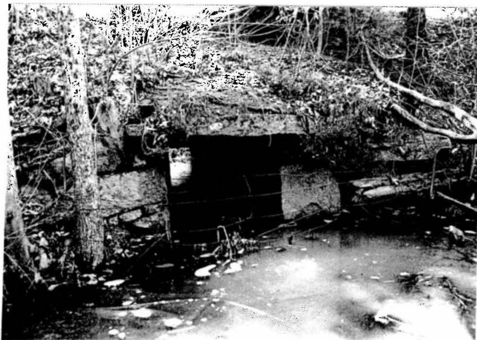
Photo # 49 description: Stone box culvert, Portsmouth (54.07) Roll #: 3 Frame #: 19 Direction:
