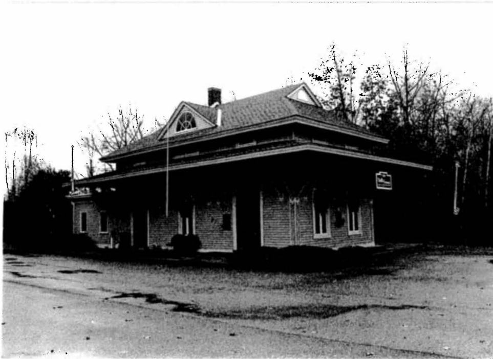
Photo # 19 description: North Hampton depot (east elevation)
