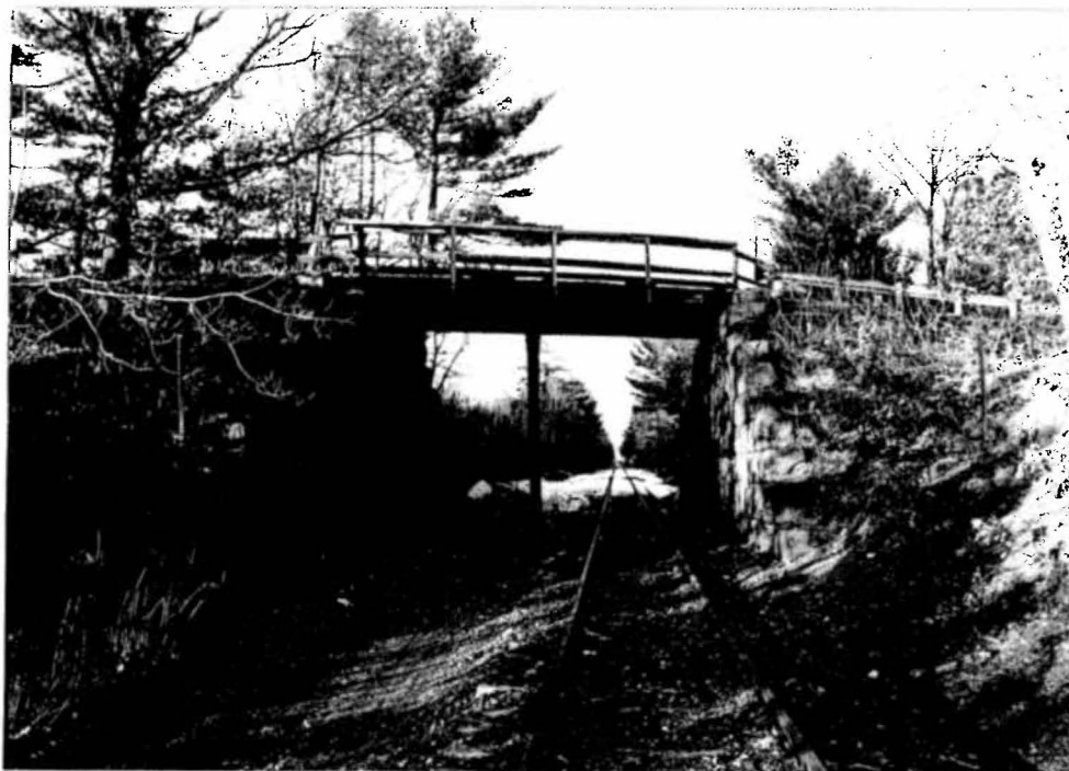
Photo # 43 description: Wood stringer bridge carrying Lobbs Hole Road over RR, North Hampton (48.18) Roll #: 5 Frame #: 11 Direction: north
