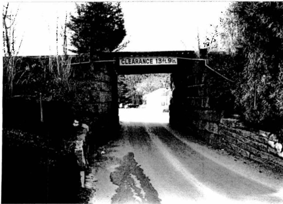
Photo # 33 description: Iron stringer bridge, Hampton (46.40) Roll #: 7 Frame #: 19 Direction: west
