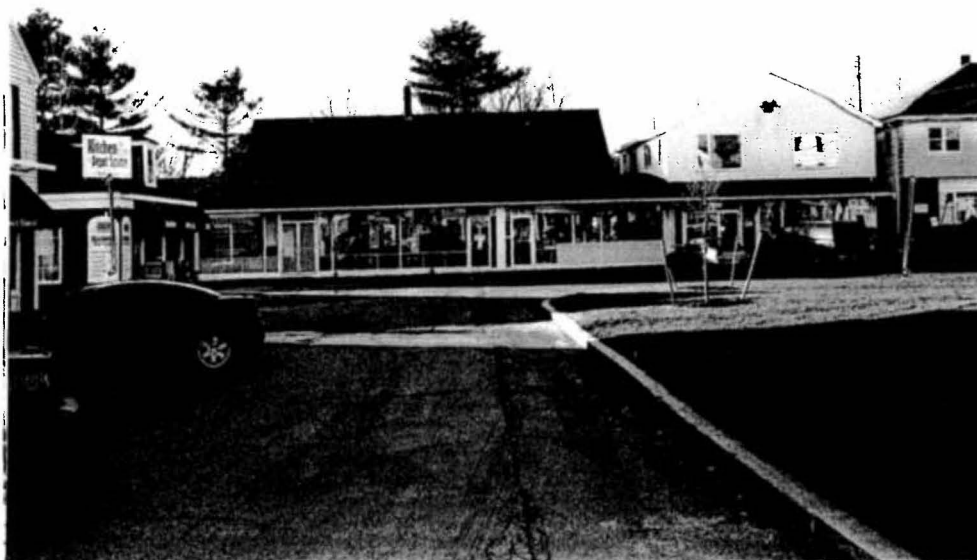
Photo #21 description: Hampton depot (East elevation)
