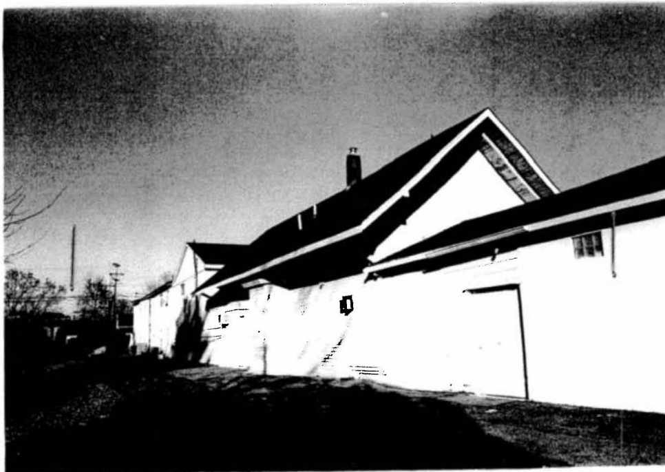
Photo #20 description: Hampton depot (west, trackside elevation)
