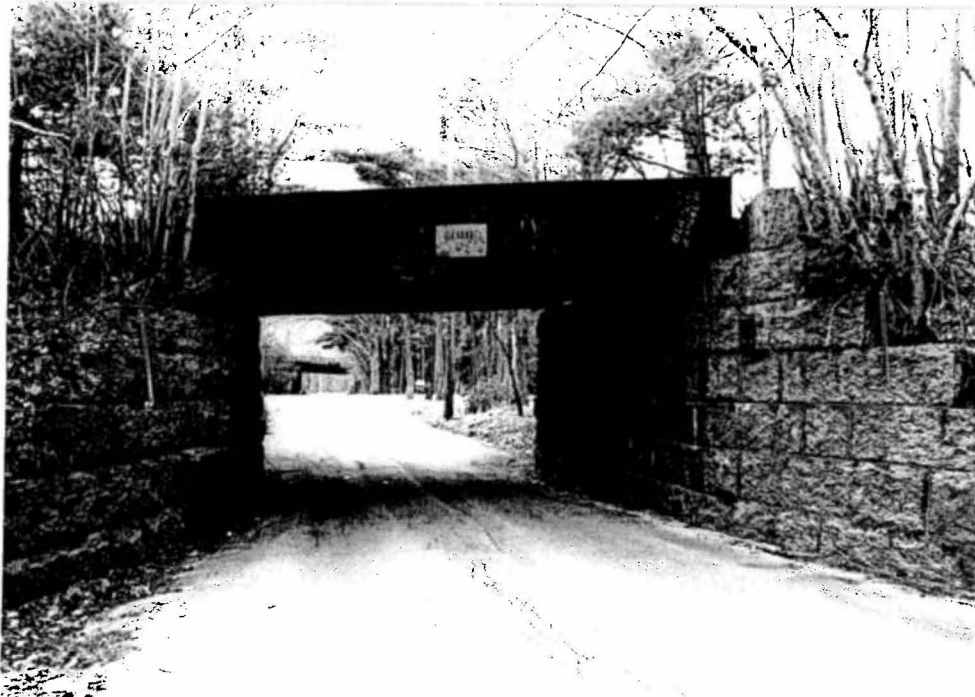
Photo #37 description: Half Thru Plate Girder Bridge over Drakeside Road, Hampton (46.02) Roll #: 8 Frame #: 2 Direction: west
