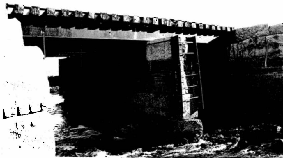
Photo # 28 description: Steel stringer bridge over Hampton Falls River (44.24)
