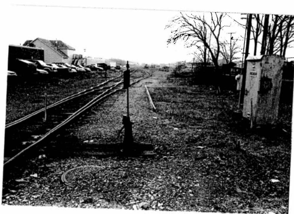
Photo # 58 description: switch and sign at Portsmouth
