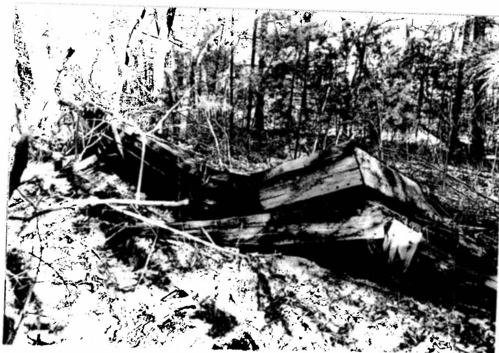
Photo # 16 description: Former Atlantic station shelter?, Seabrook
