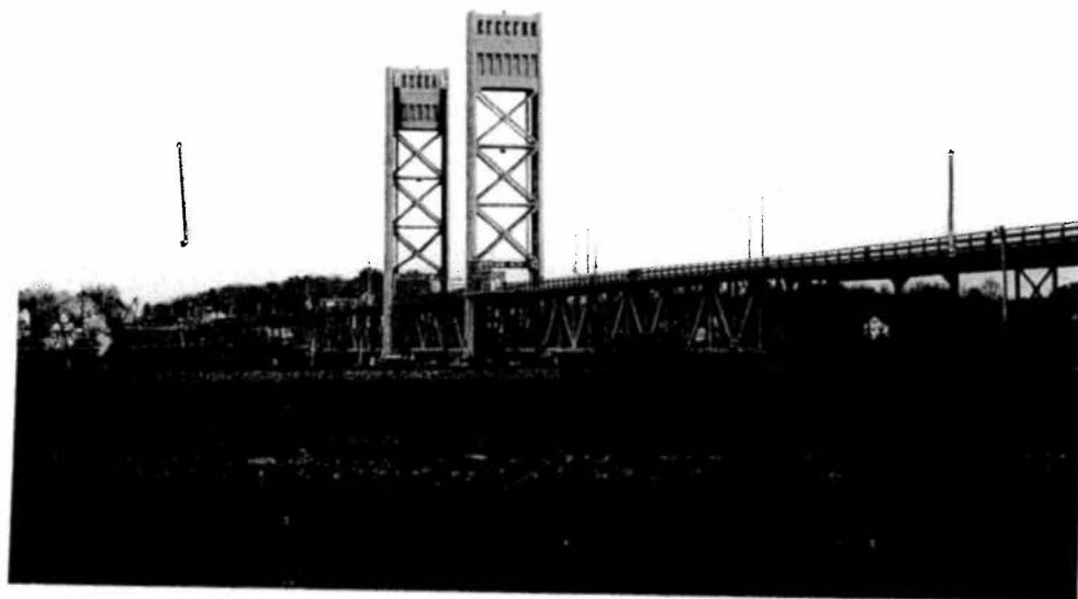
Photo # 40 description: Interstate (Long) Bridge, Portsmouth (57.23)
