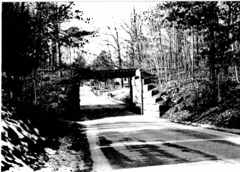
Photo #27 description: Steel stringer bridge over Walton Road, Seabrook (41.92)
