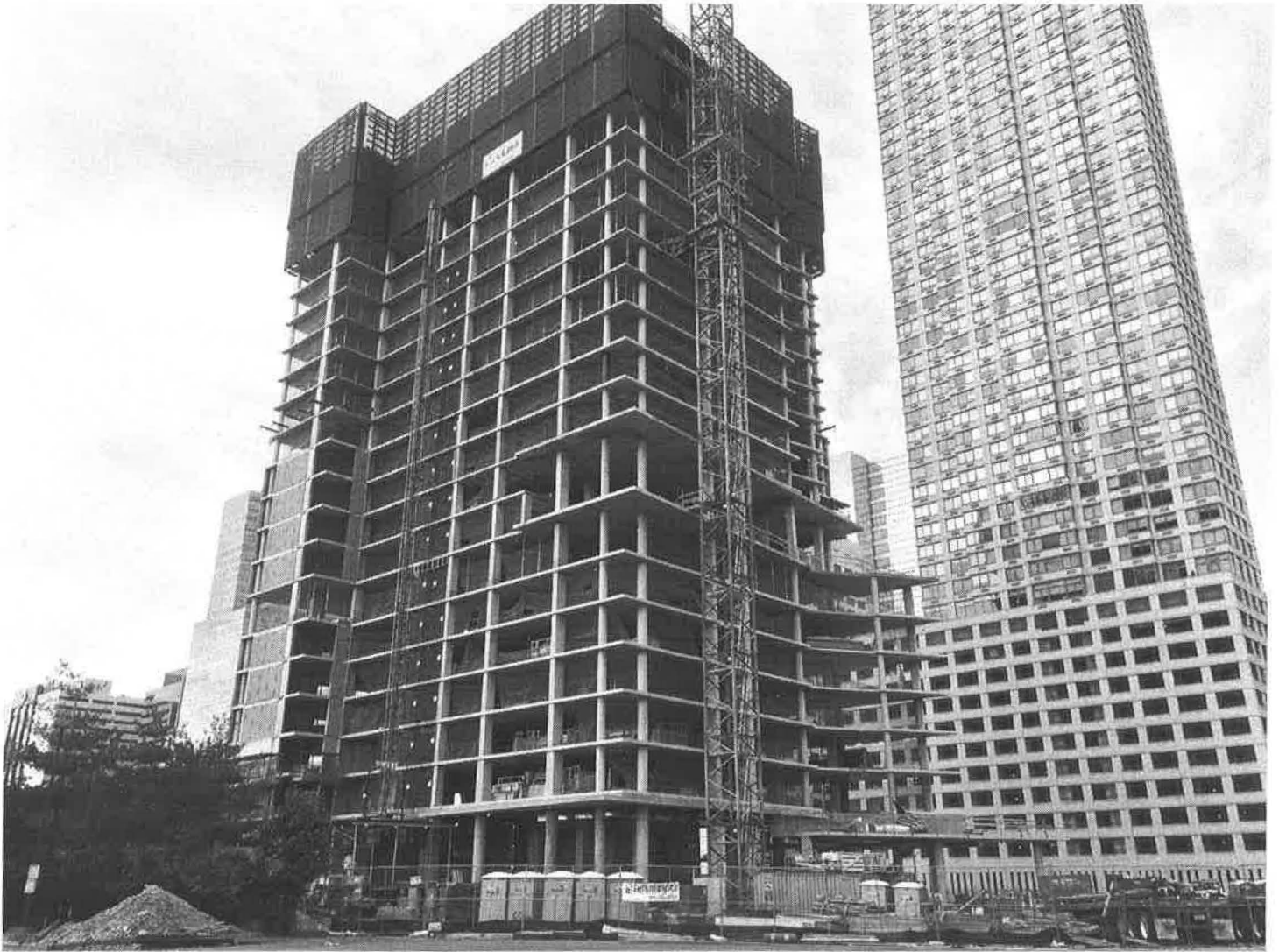
The first tower under construction at Hudson Exchange West
