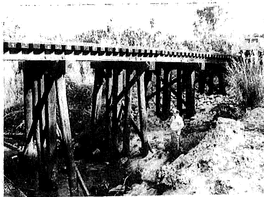
WEST SIDE LOOKING SOUTH
