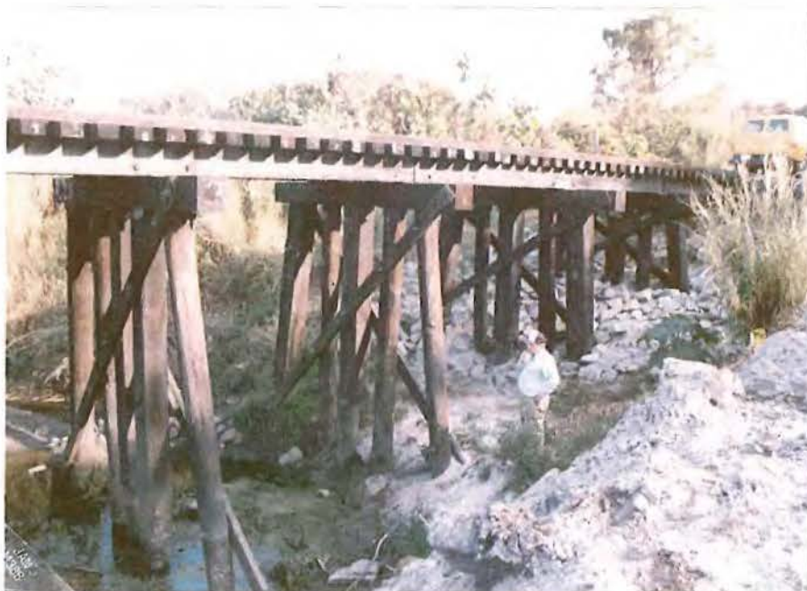
WEST SIDE LOOKING SOUTH
