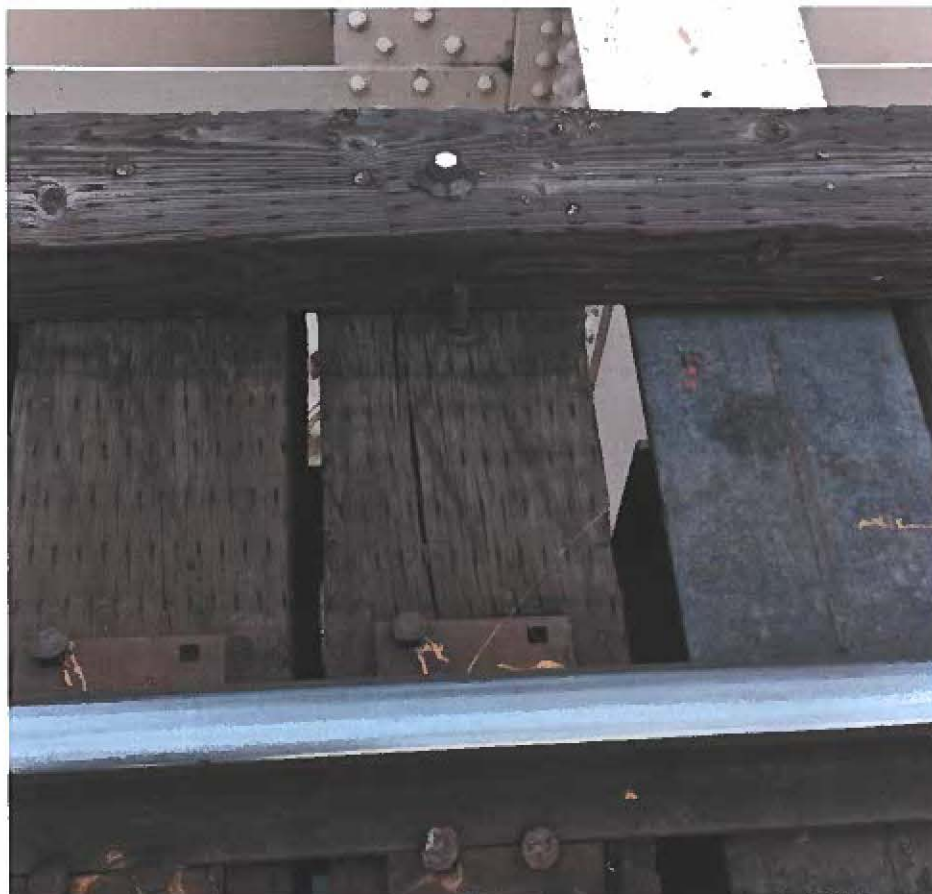
Picture 1 showing an old tie with a new crosstie spacer bolt installed.
