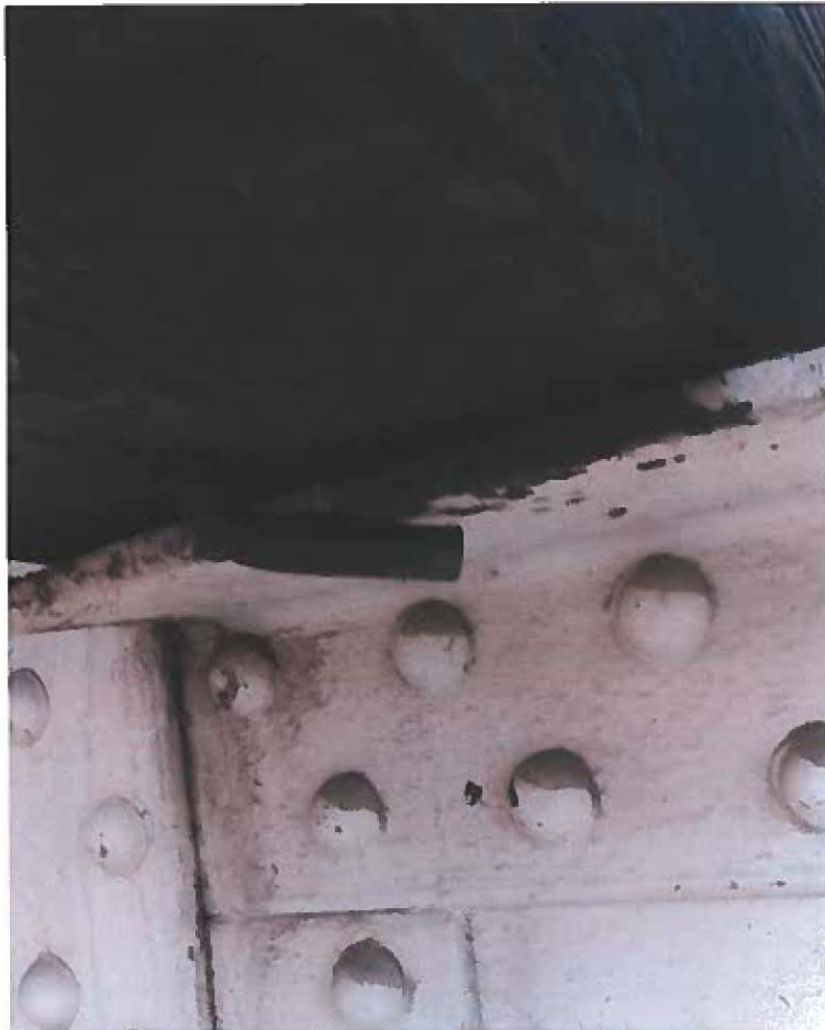
Picture 3 of a J bolt beginning to rotate out of position.
