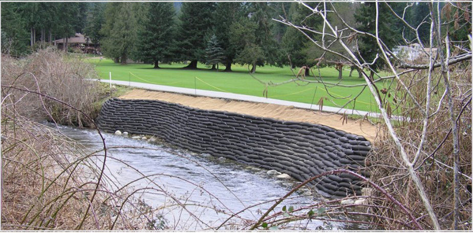
An example of river bank stabilization adjacent to a trail
