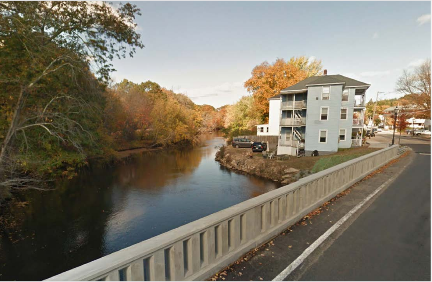
View of flood-prone property at the Providence Street / Rte. 122 bridge in the Rockdale section of Northbridge, looking northwest (Key #68)
