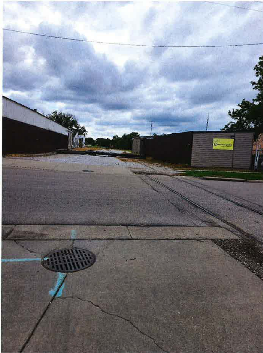
2. Tracks looking west from North 23 rd Street.
