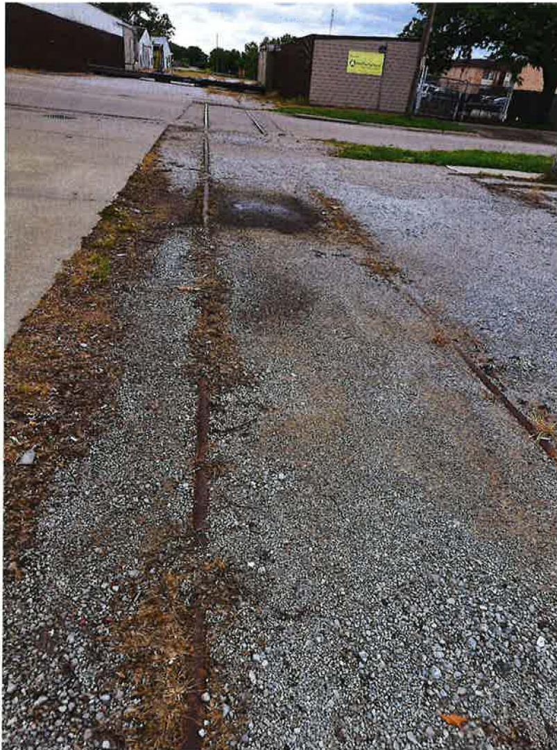
1. Tracks looking west from North 23 rd Street
