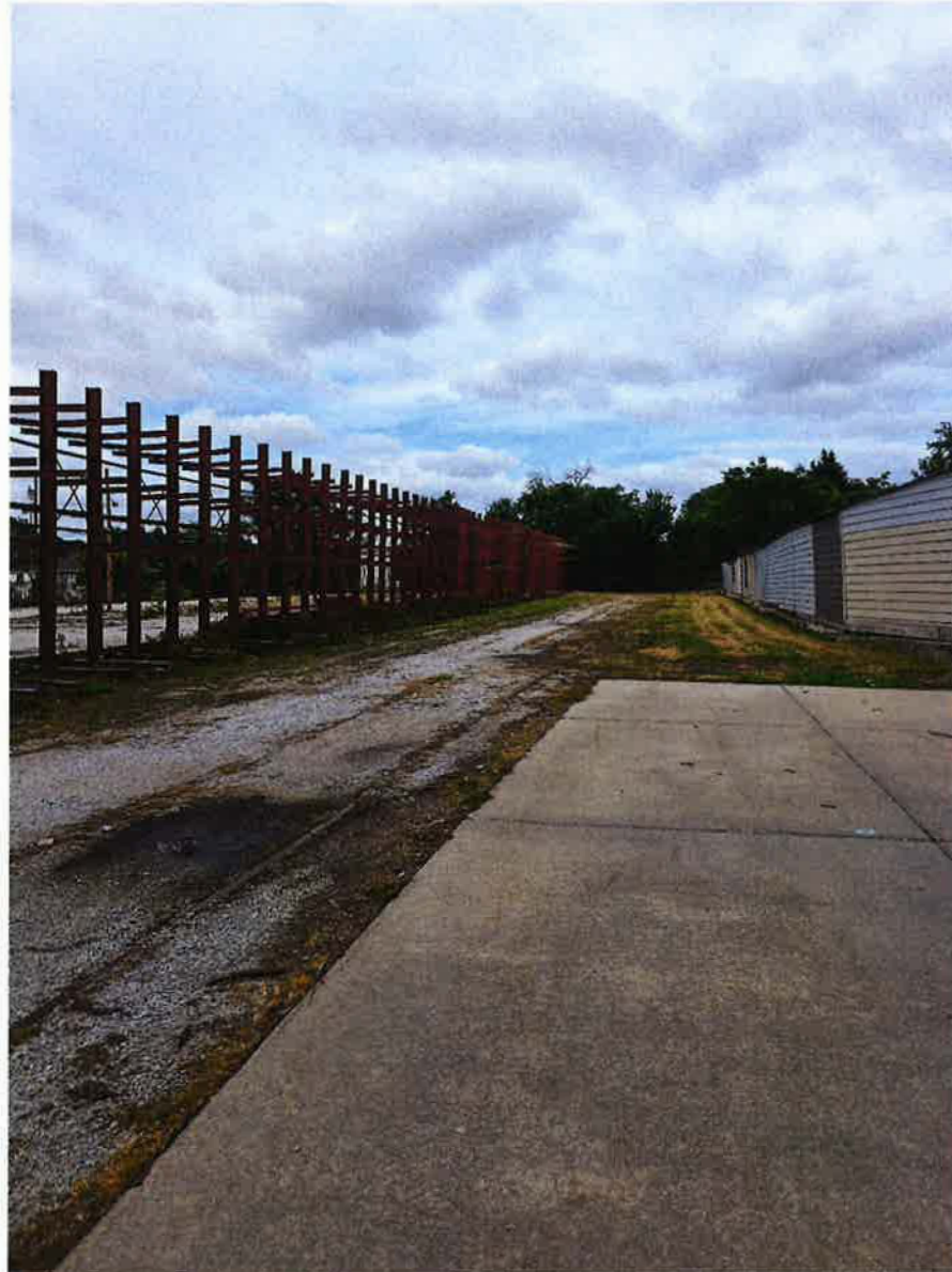
4. Tracks looking northeast from North 23 rd Street.
