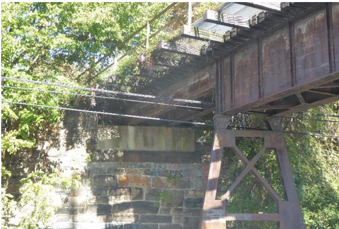
Photo 13. Wilkens Ave Bridge (10/23/24 [20241])
