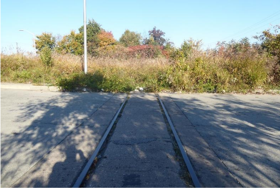
Photo 17. RR Corridor at Wilmarco St (10/23/24 [20205])
