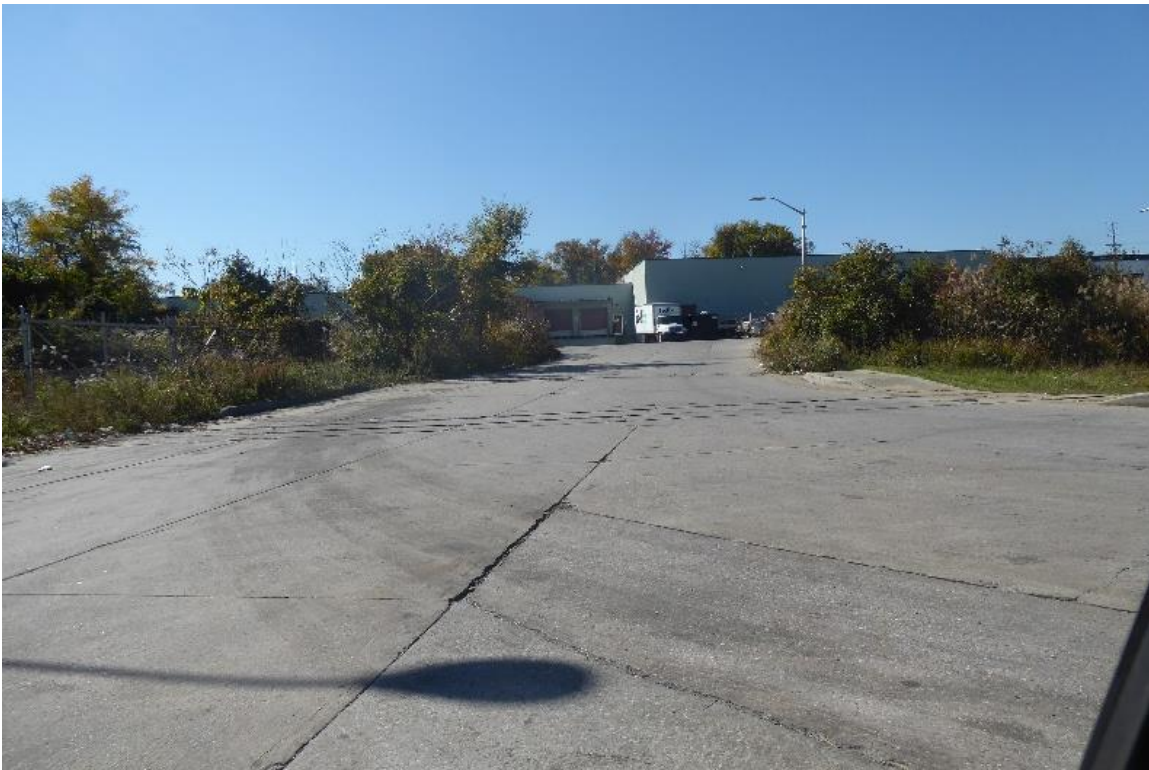
Photo 18. RR Corridor at Wilmarco St (10/23/24 [20304])
