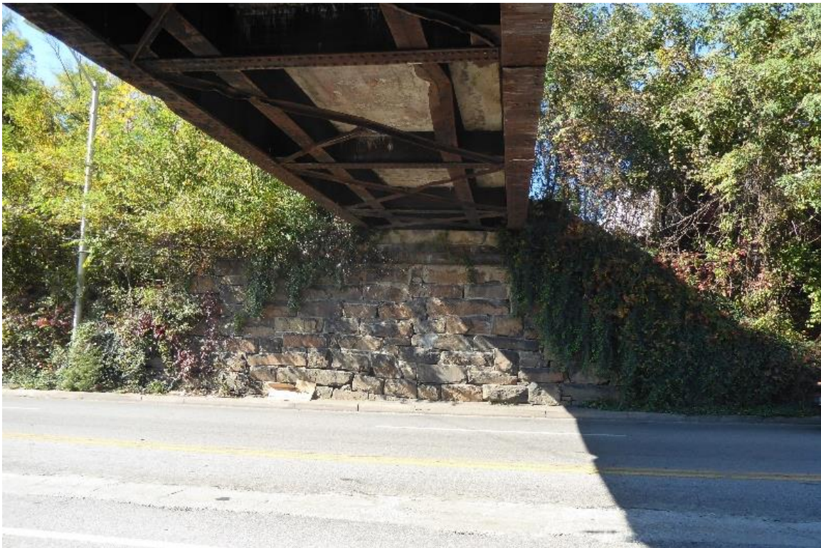
Photo 5. Caton Avenue Bridge (10/23/24 [20263])
