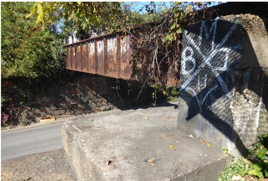
Photo 6. Caton Avenue Bridge (10/23/24 [20267])
