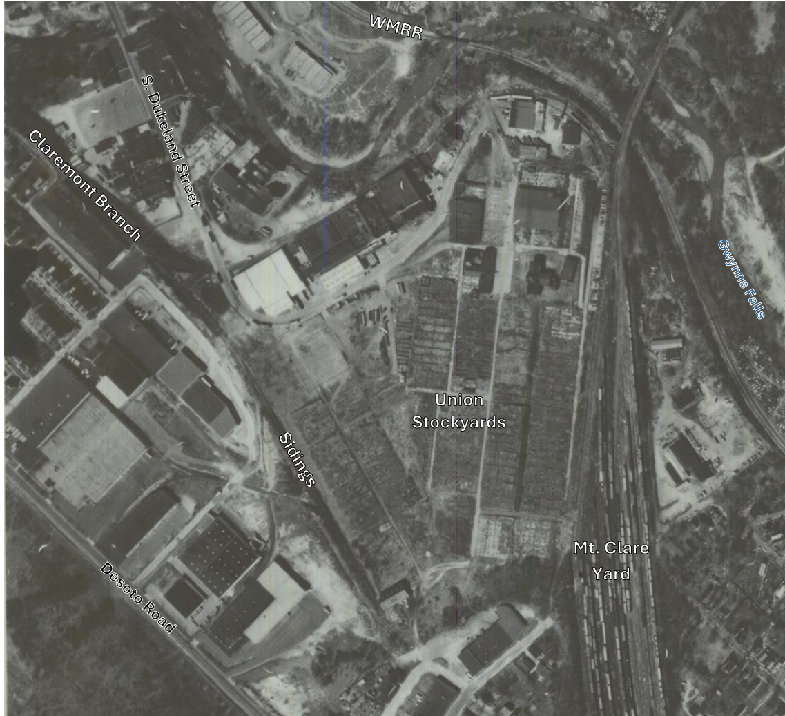
Exhibit 7. Portion of 1972 aerial photograph showing the Claremont Branch. By this time the Union Stockyards had ceased operations. Train cars are visible on the Claremont Branch at its northern most bend as it approaches the north end of the Mt. Clare Yard.
