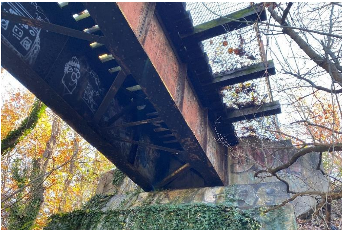
Photo 15. Wilkens Ave Bridge (11/21/24 (0945))
