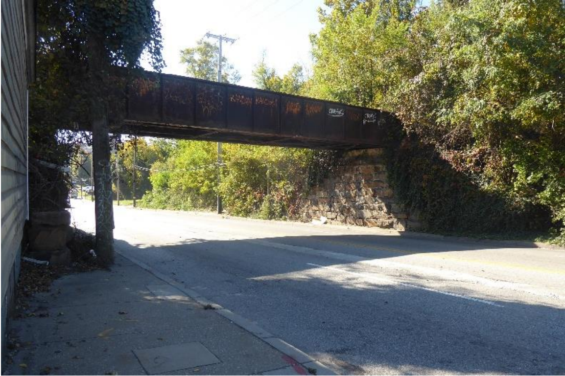
Photo 4. Caton Avenue Bridge (10/23/24 [20261])
