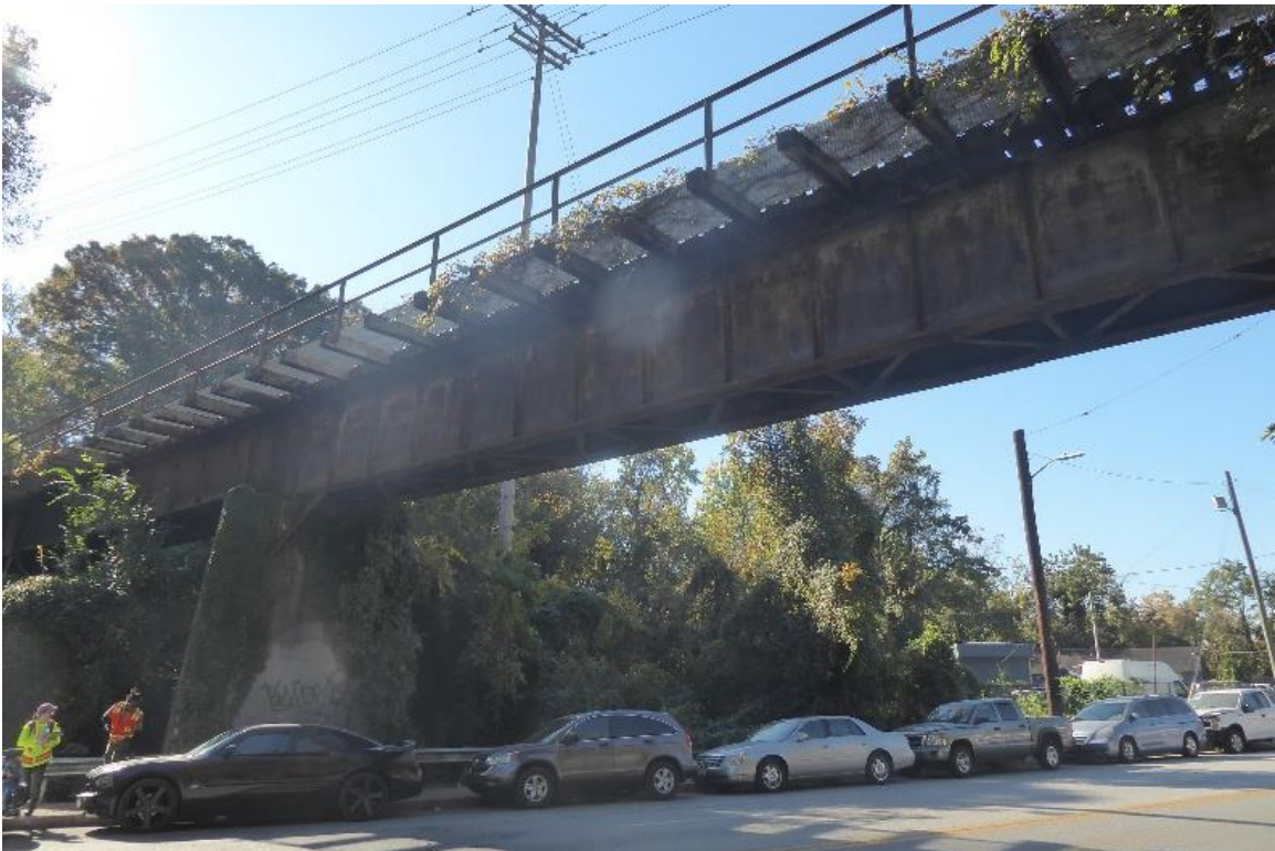
Photo 11. Wilkins Ave Bridge (10/23/24 [20239])
