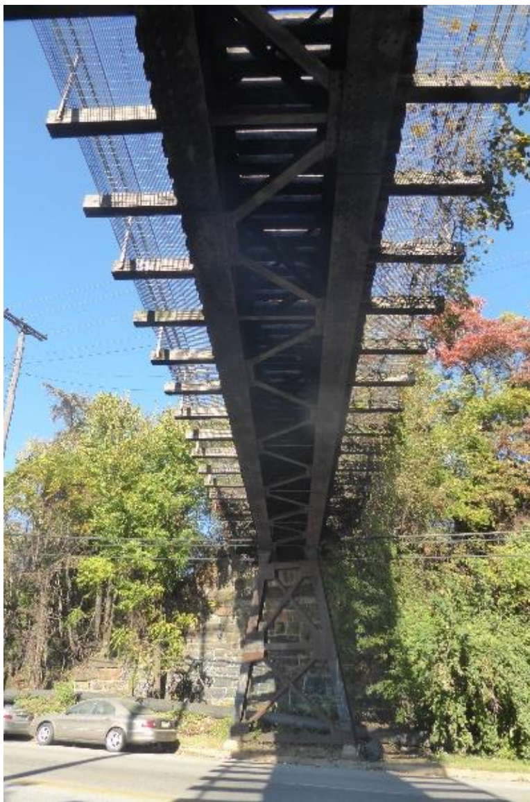
Photo 12. Wilkens Ave Bridge (10/23/24 [20239])
