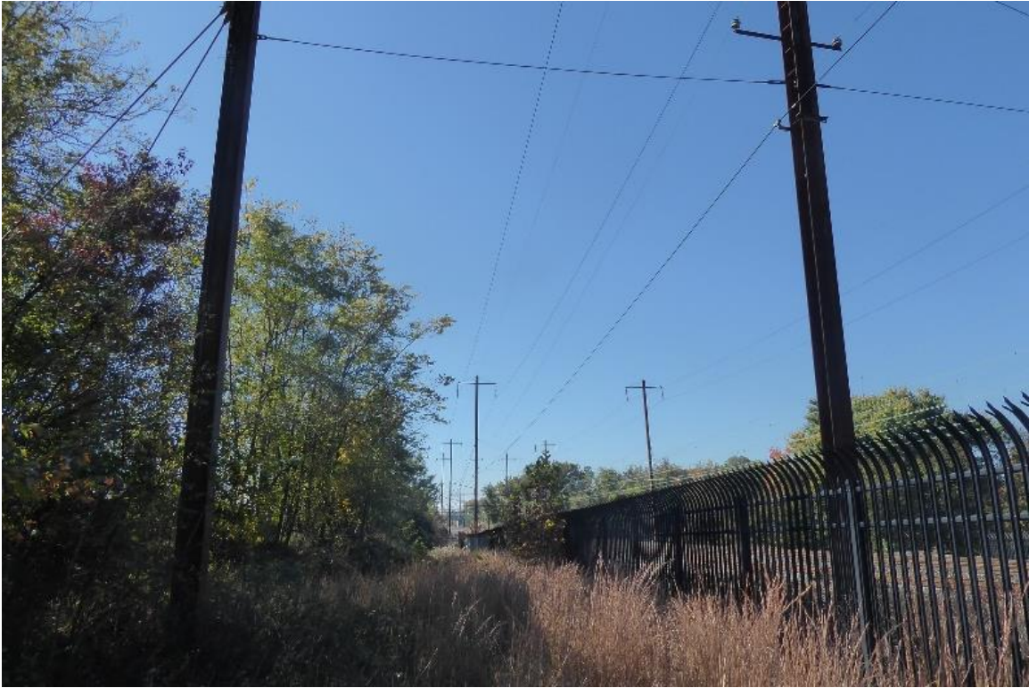
Photo 1. Remnant Wye Junction at NEC (10/23/24 [20249])
