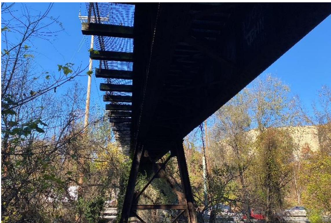
Photo 14. Wilkens Ave Bridge (11/21/24 [0952])
