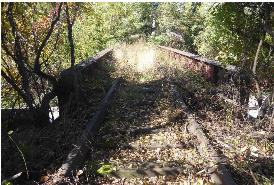
Photo 7. Caton Avenue Bridge (10/23/24 [20268])
