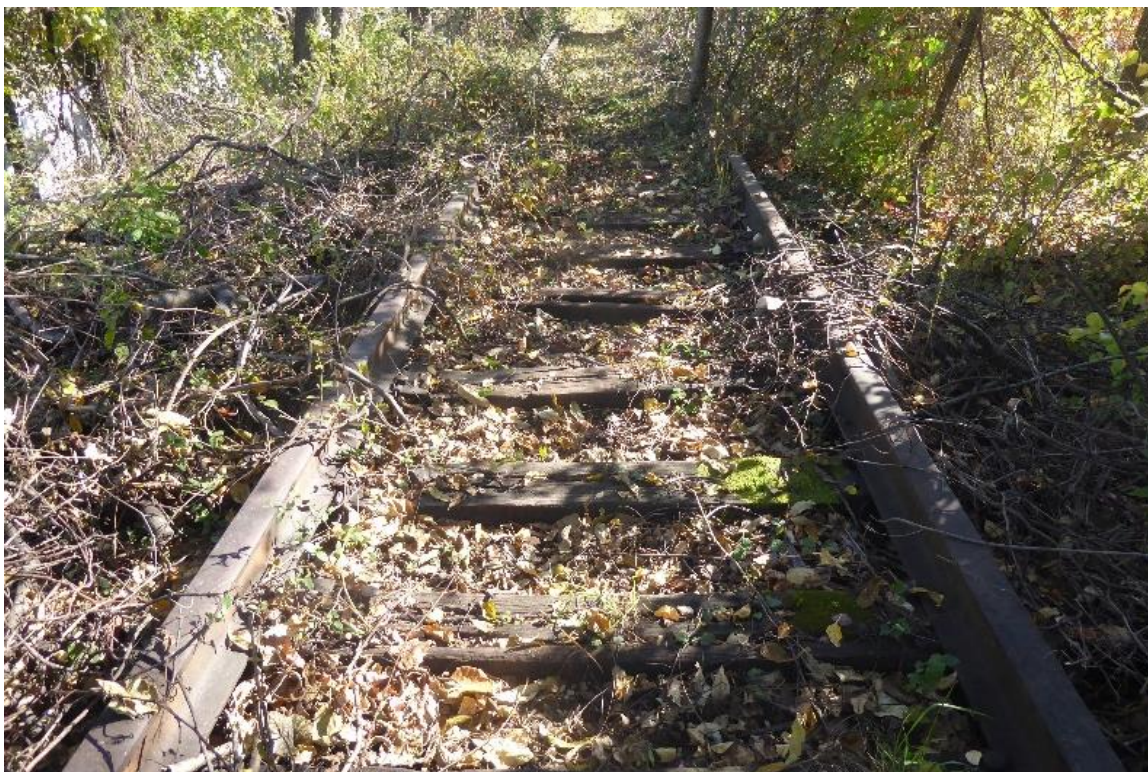
Photo 8. RR Corridor S. of Caton Ave (10/23/24 [20271])
