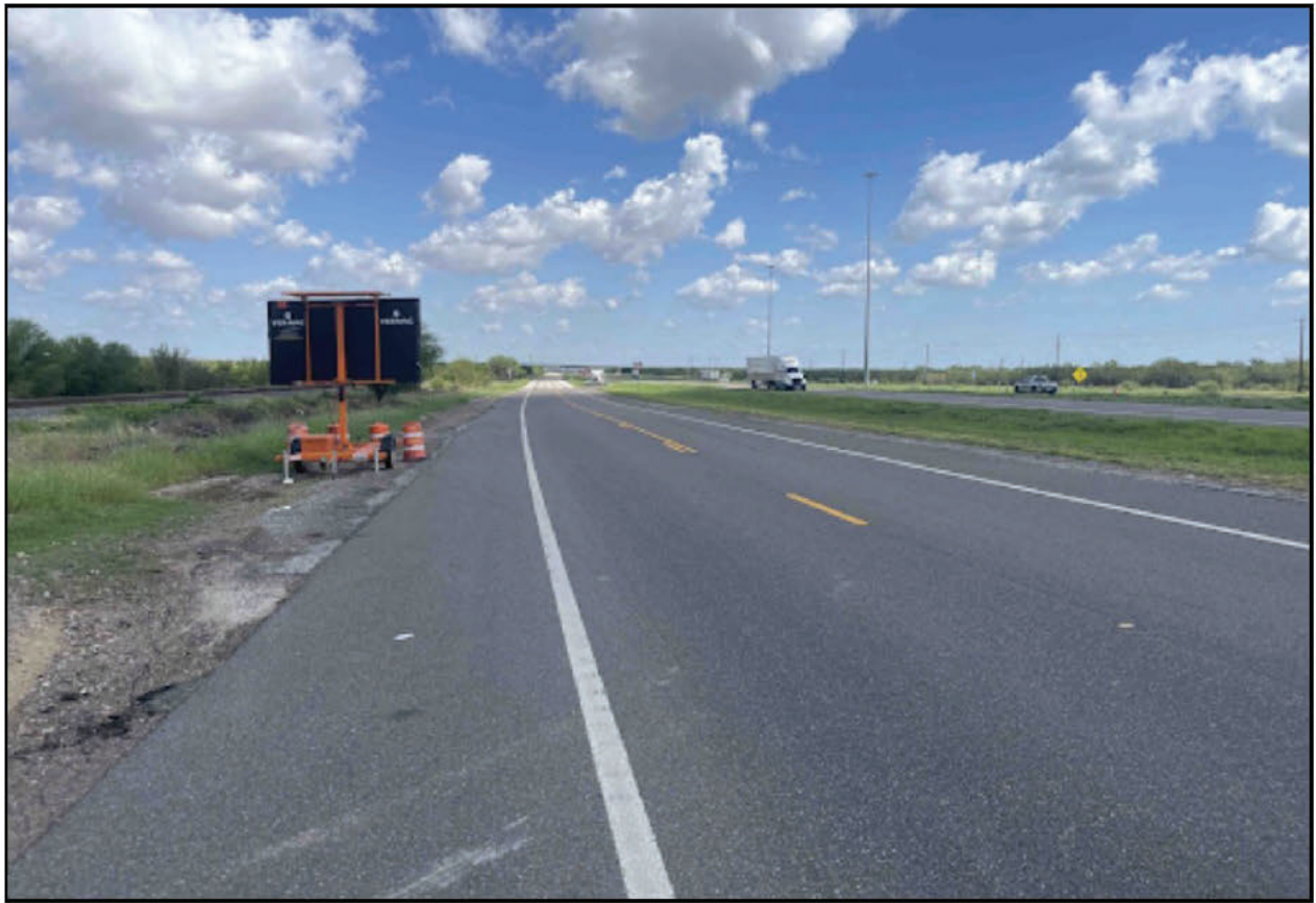
Figure 19. View of W-01, Facing Northeast Along the Frontage Road, with Views of the North and Southbound Lanes of I-35 to the East.
