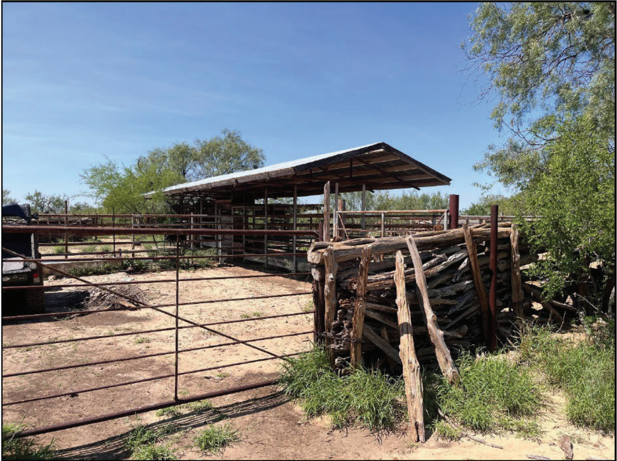
Figure 21. View of W-03, Facing West towards open sided shed.
