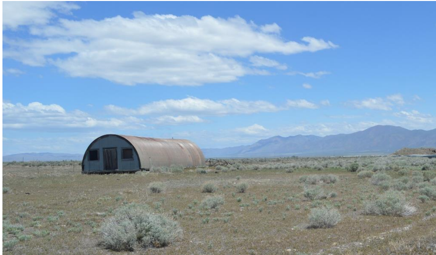
Figure 5. Quonset hut on abandoned farmland in Crescent Valley.
