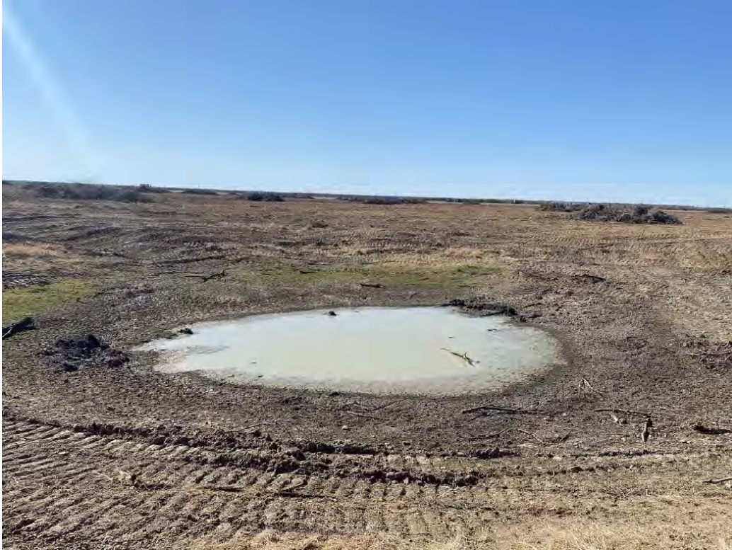
Photo 9. View of P-2, an excavated pond recently cleared of vegetation, facing west
