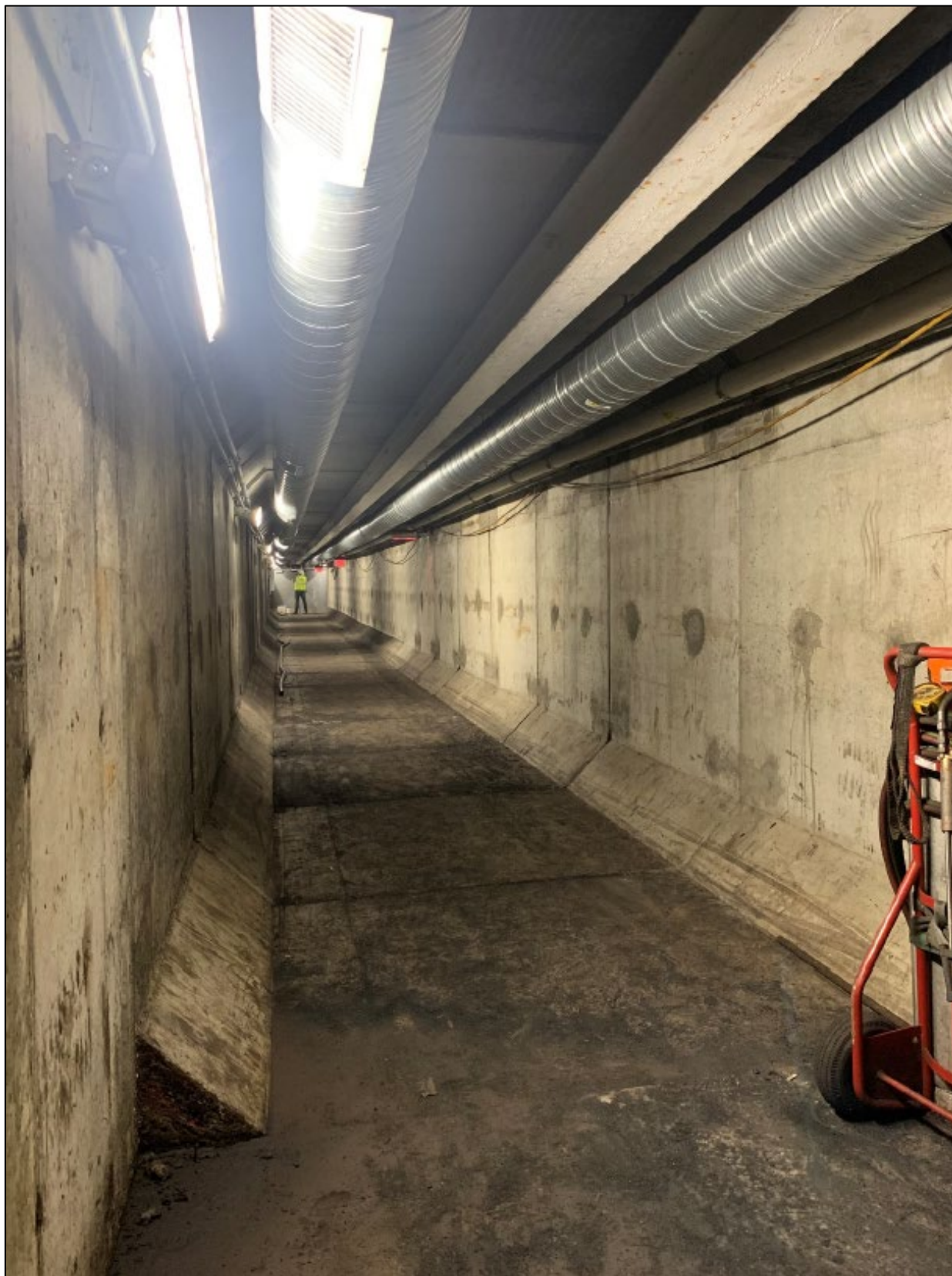
Figure 2.2.1. North Escape Tunnel as seen on July 9, 2020.
