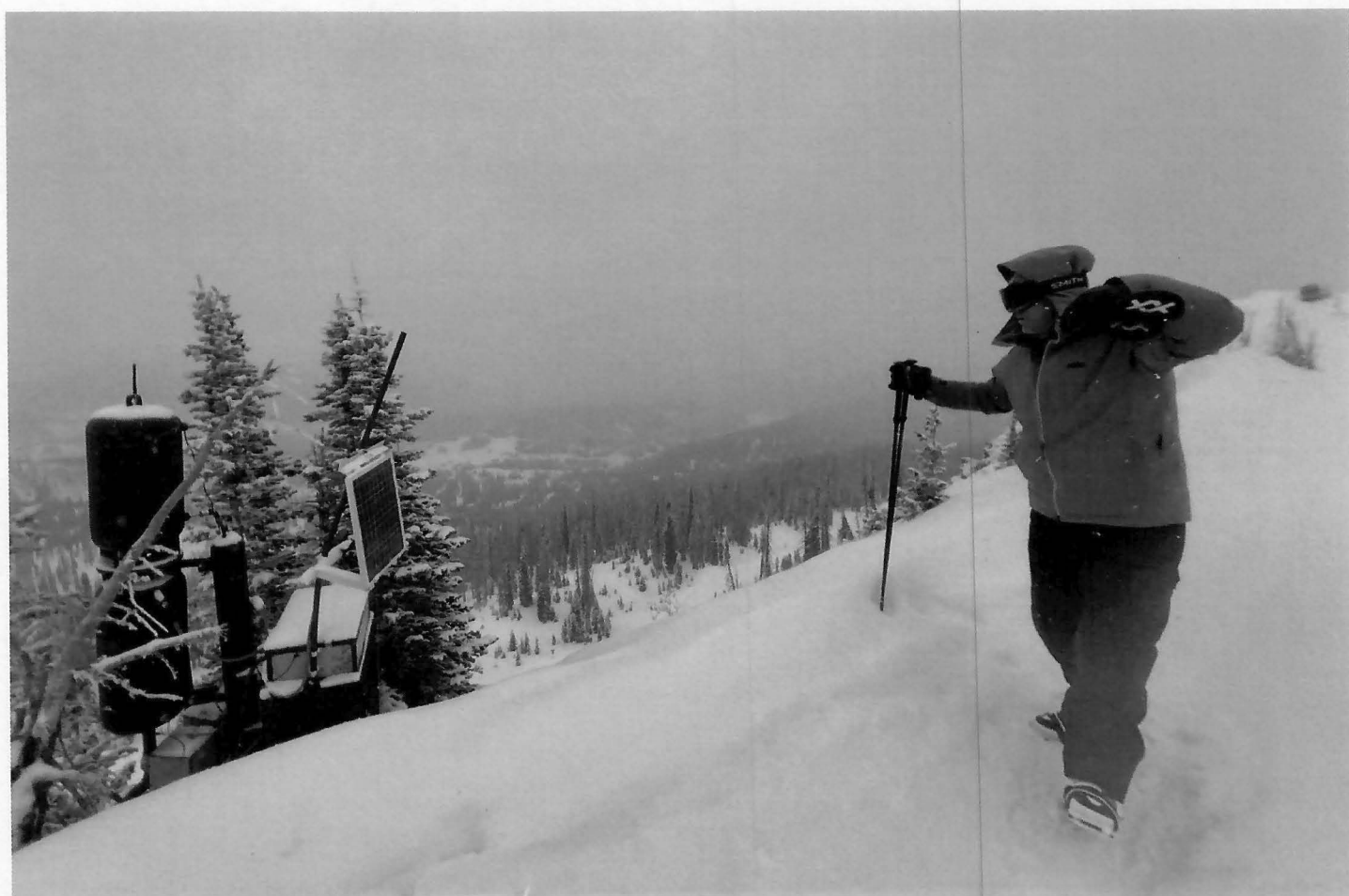
Davey Pitcher hikes on a ridge above the avalanche mitigation devices he built to help keep the high-elevation resort safer
