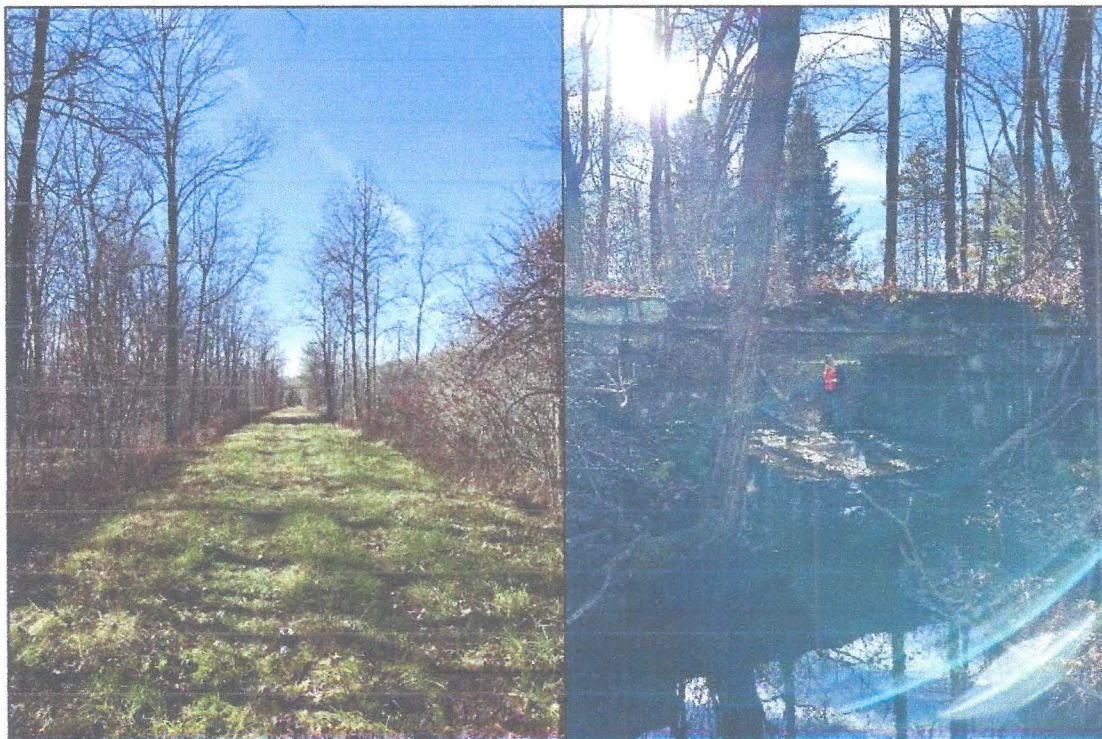
Figure 2 - Existing Railroad Grade and Bridge Structure
