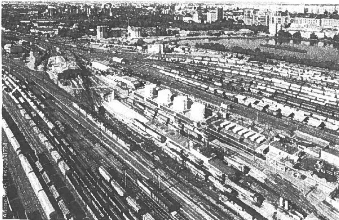
A typical rail yard
