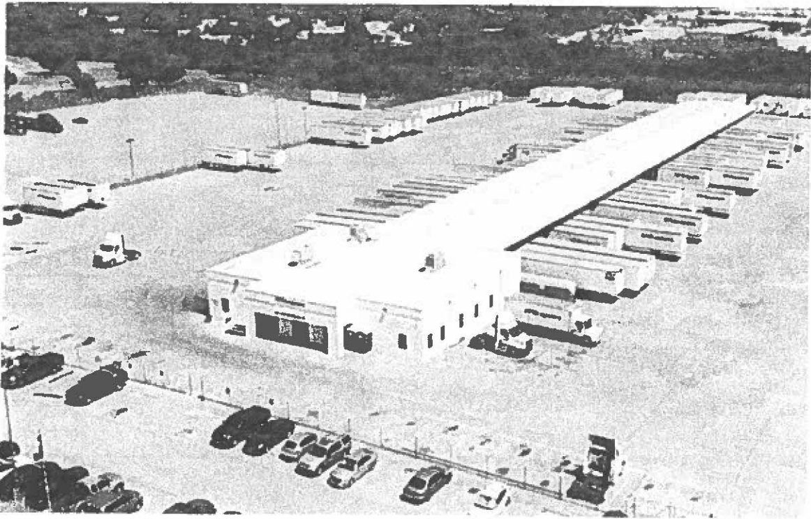
A typical truck terminal
