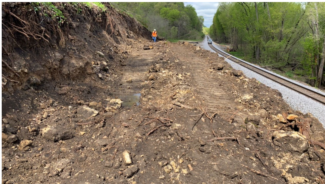
Figure 3. Initial topsoil clearing and berm construction with undisturbed portions of ROW visible in background; facing Northwest. (M. Richison 04/29/24)
