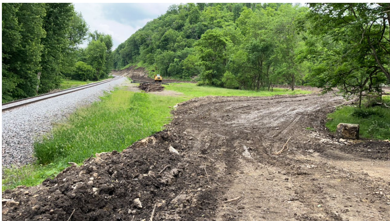
Figure 7. Topsoil removal in staging area, near three-pipe box culvert; facing Southeast. (M. Richison 06/04/24)
