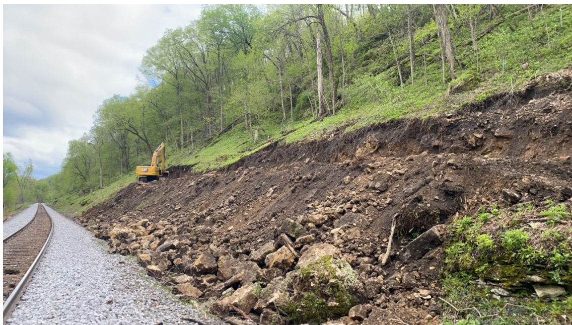
Figure 2. Initial topsoil clearing near MP 69.48; facing Southeast. (M. Richison 04/29/24)
