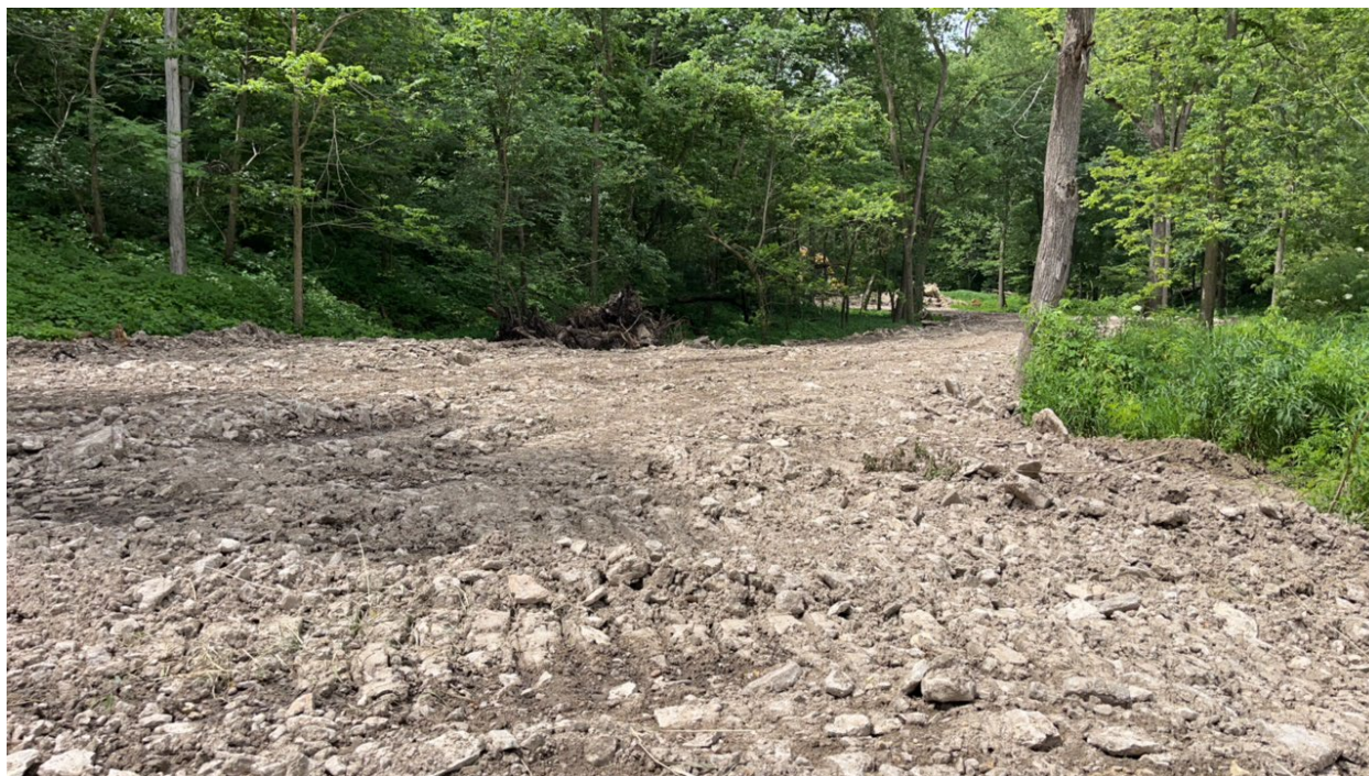
Figure 10. Topsoil removal and access road construction, western portion of project area; facing South. (M. Richison 07/01/24)
