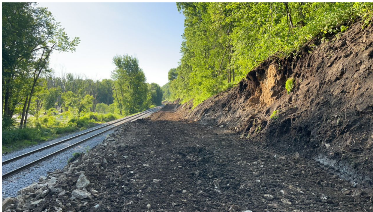
Figure 6. Topsoil and overburden removal; facing East. (M. Richison 05/30/24)
