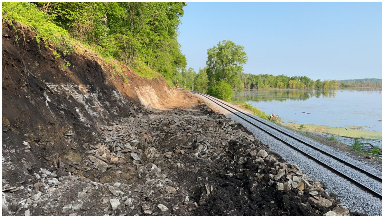
Figure 5. Topsoil and overburden removal; facing Northwest. (M. Richison 05/15/24)
