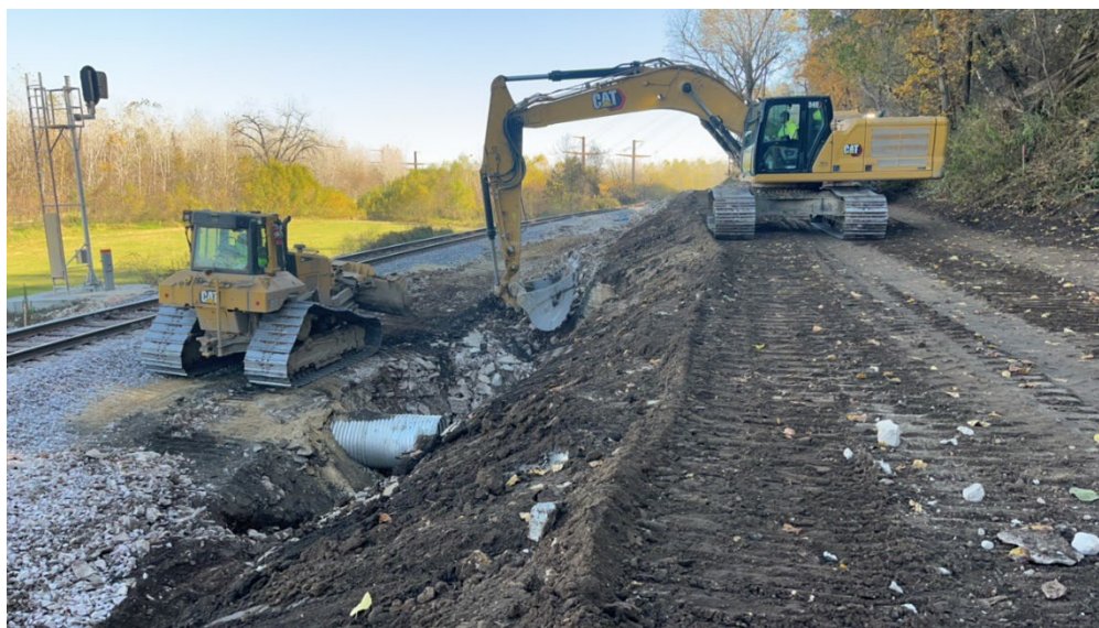
Figure 20. Culvert area cleanup after installation, near westernmost extreme of project area standing on 360 th St; facing east. (M. Richison 10/24/24)
