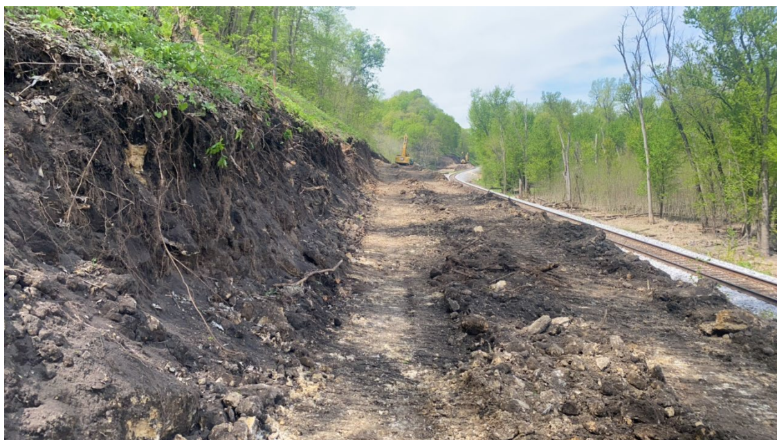
Figure 4. Initial topsoil clearing near private farm access road, eastern portion of project; facing Northwest. (M. Richison 05/01/24)
