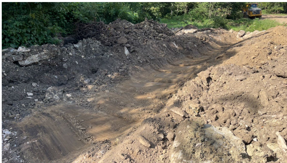
Figure 13. Example of excavated trench for erosion and water control; facing Southeast. (M. Richison 08/09/24)
