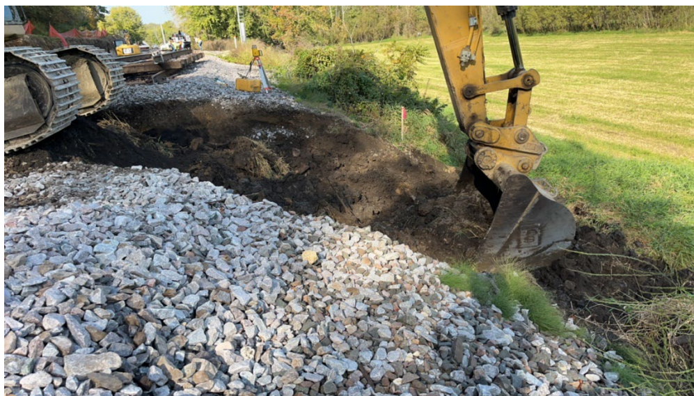
Figure 19. Culvert installation under existing railroad, near western extreme of project area and railroad crossing; facing Northwest. (M. Richison 10/09/24)
