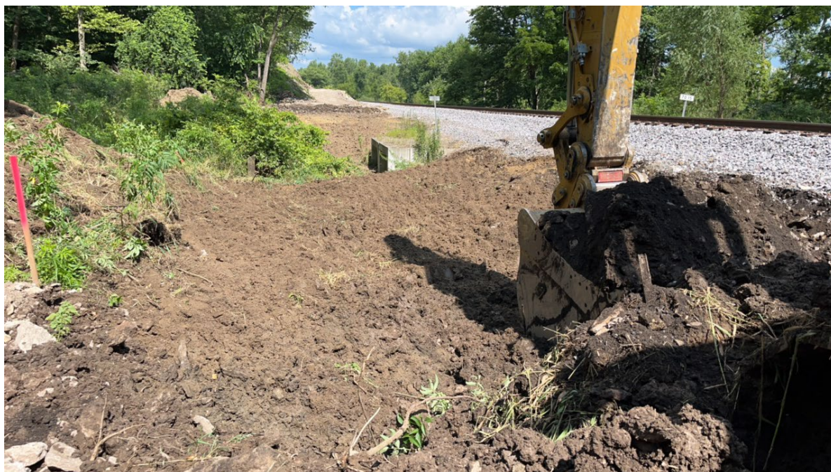
Figure 11. Topsoil removal and bridge construction staging area, at MP 70.15; Facing west. (M. Richison 07/11/24)
