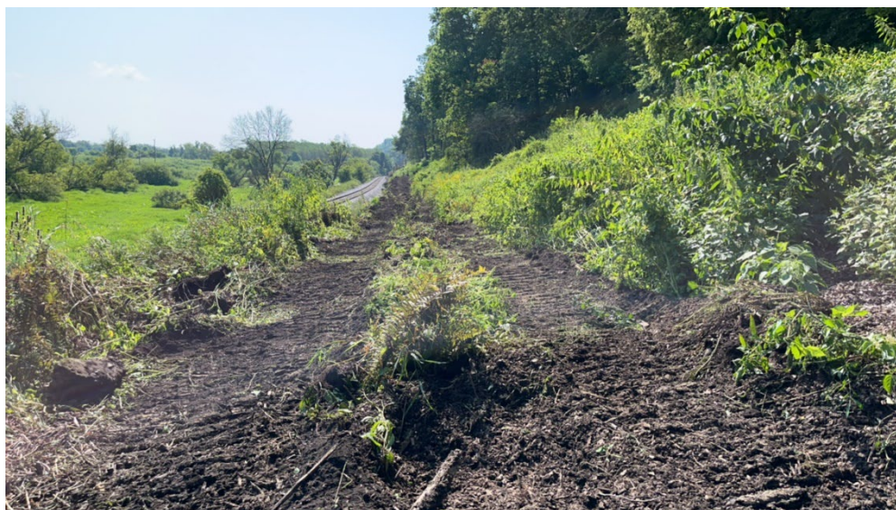
Figure 14. South Singer Switch Cabin project location, new disturbance complete; facing Northeast. (M. Richison 05/06/24)
