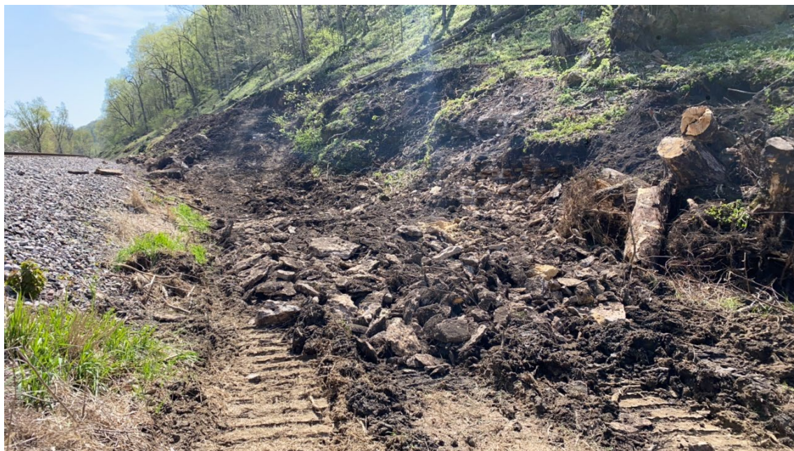
Figure 1. Initial topsoil clearing for railroad siding construction; facing East. (M. Richison 04/25/24)
