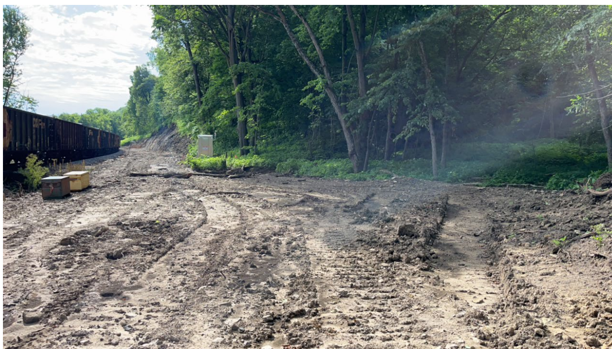
Figure 9. Access to southern bridge and staging area topsoil removal, easternmost extent of project area; facing Southeast. (M. Richison 06/26/24)
