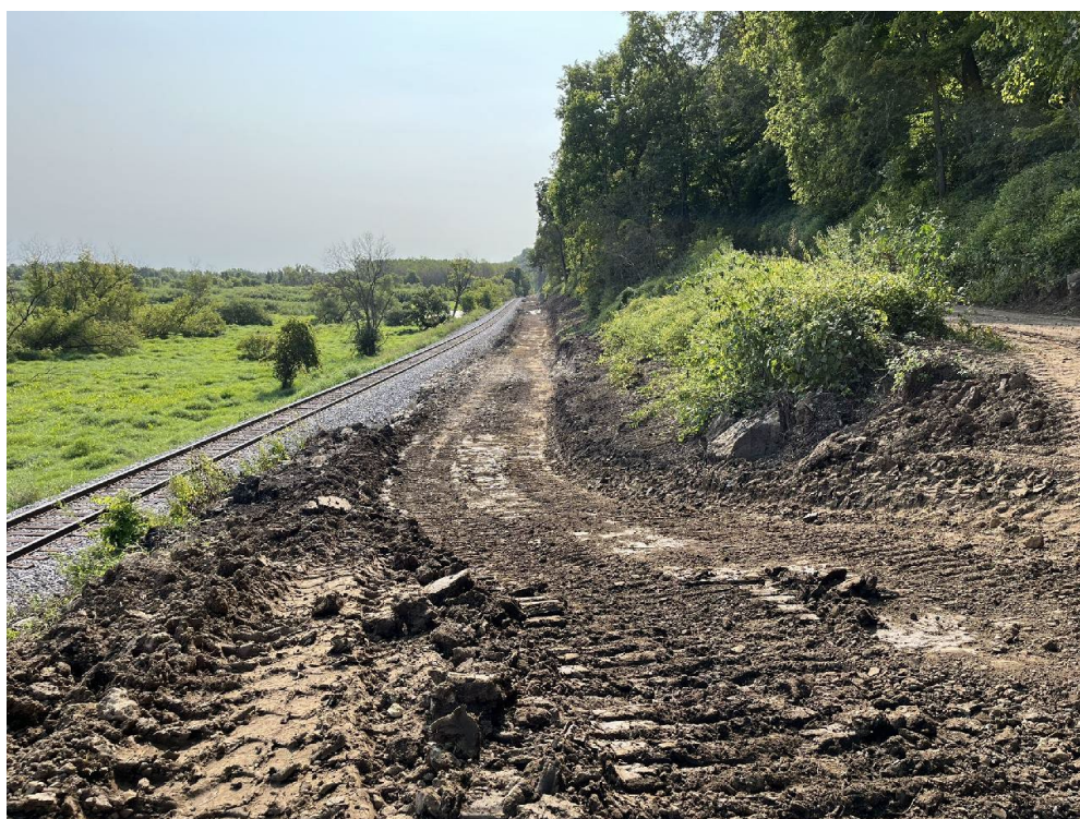
Figure 16. Access from 360 th St to ROW with topsoil and overburden removed, turn around point for haul truck traffic; facing East. (M. Richison 09/09/24)
