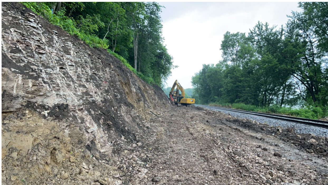
Figure 8. An example of overburden removal and extent of bedrock in ROW area, western section of project area; facing West/Northwest. (M. Richison 06/20/24)
