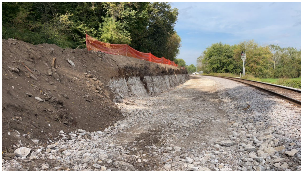
Figure 17. 360 th St entrance to ROW topsoil and overburden removal complete, westernmost area of project area near railroad crossing; facing Northwest. (M. Richison 09/18/24)
