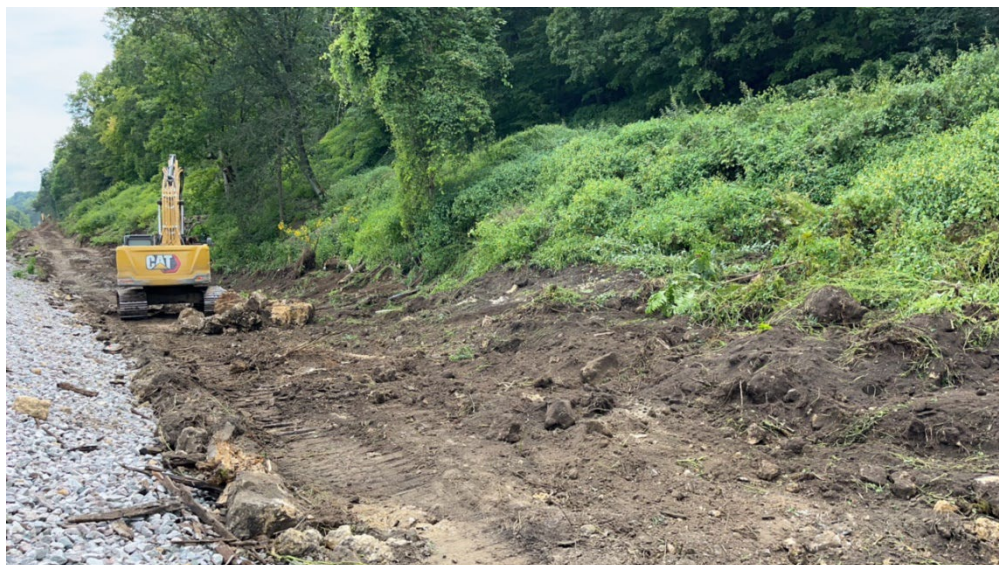
Figure 15. Topsoil removal on western portion of ROW; facing Southeast. (M. Richison 08/20/24)
