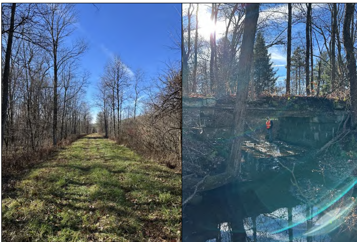
Figure 2 - Existing Railroad Grade and Bridge Structure
