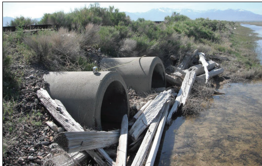
Figure 9. Feature 1. Two concrete culverts along 42TO505, facing southeast along railroad alignment.
