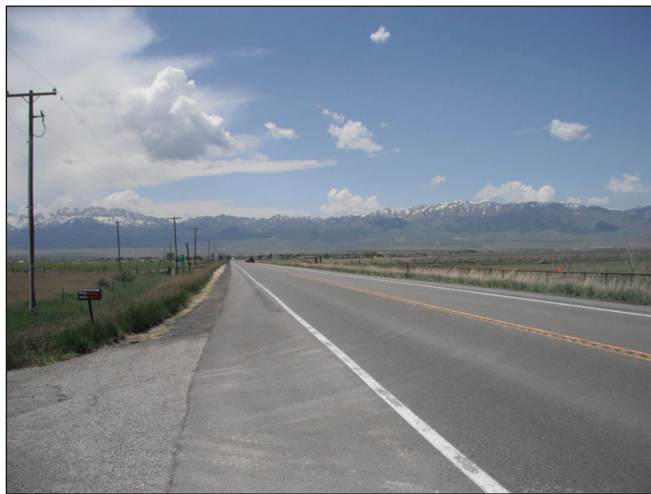
Figure 11. View west of State Highway 138 which is the alignment of the Lincoln Highway, 42TO1077 in the APE.
