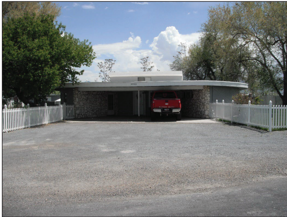
Figure 7. View south of structure at 3932 Marshall Road, Grantsville, Utah
