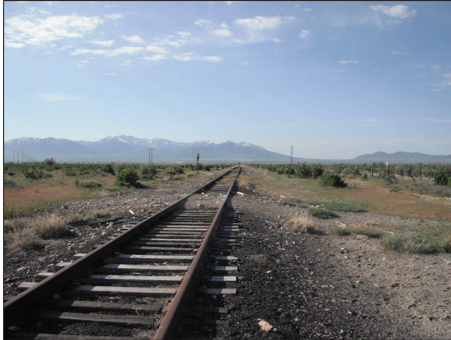
Figure 6. Overview of APE and existing railway, looking south from the northern end.
