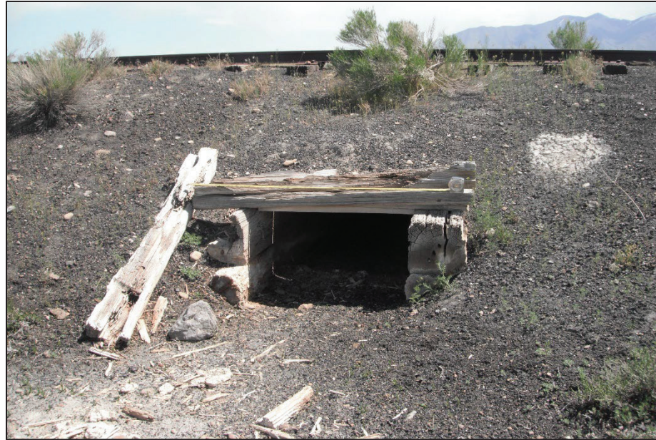
Figure 10. Example of a box culvert (Features 2-6) at 42TO505, facing northeast.
