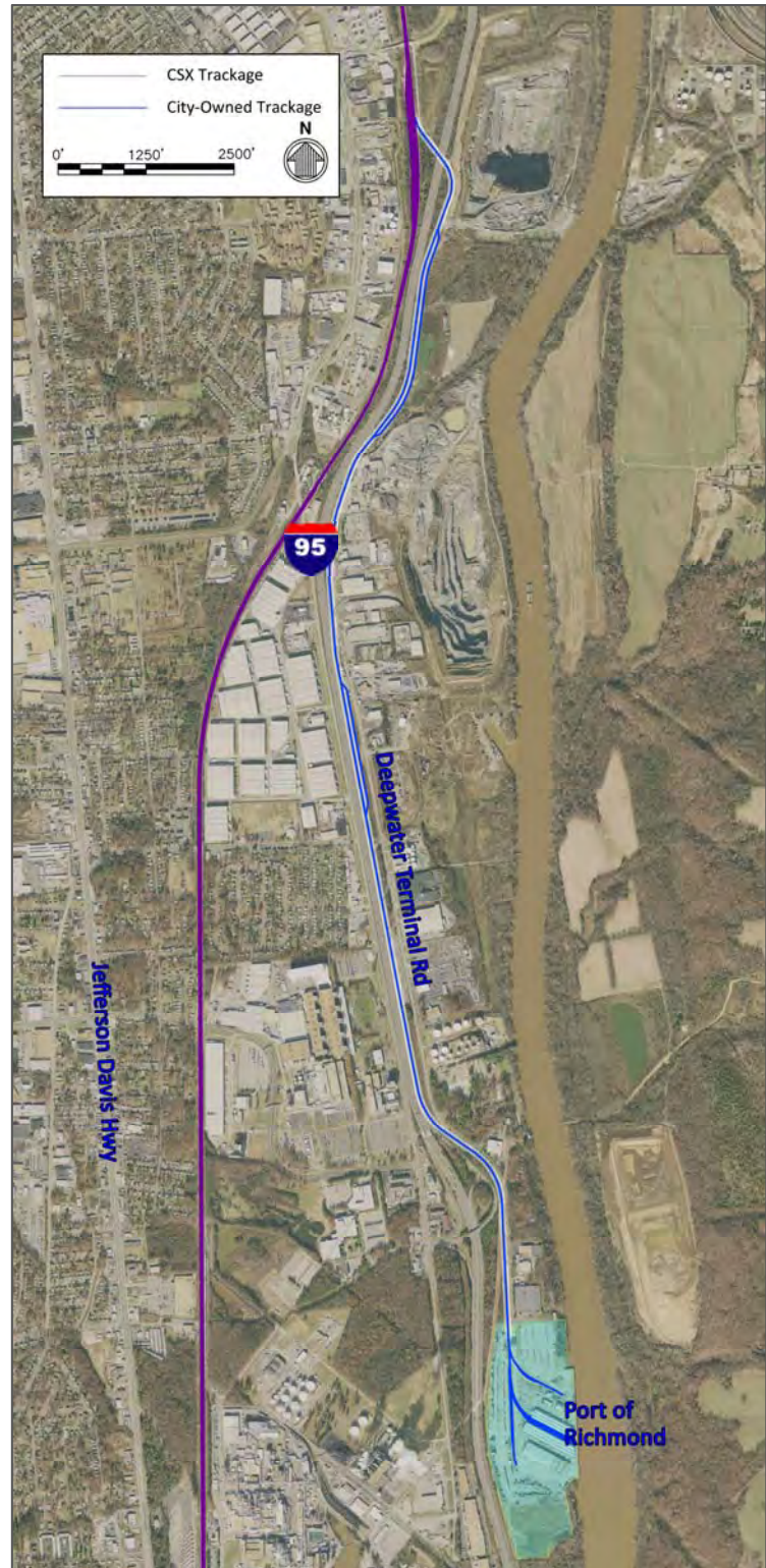
Figure 28 – Port of Richmond Overall Rail System
