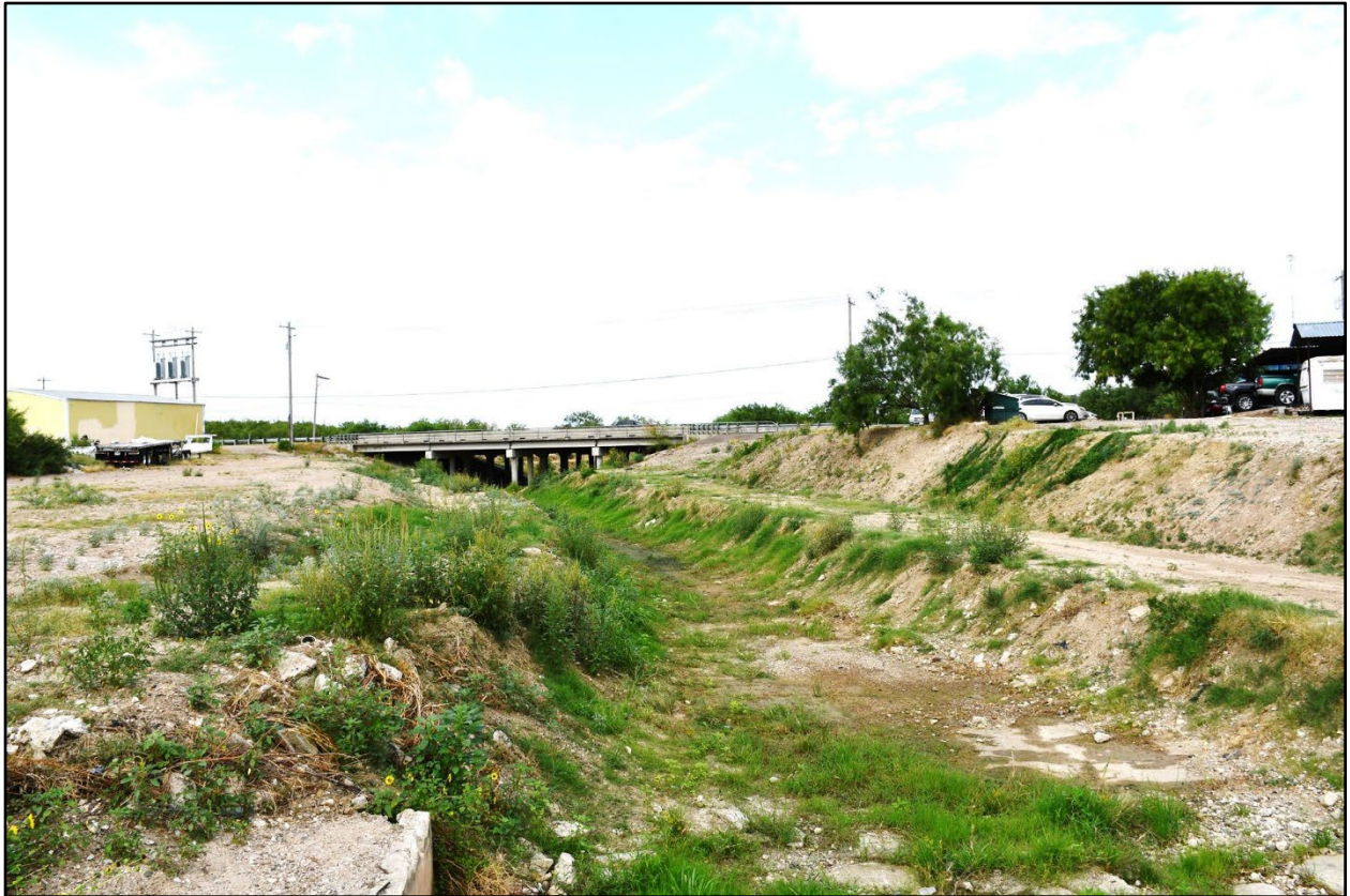
Figure 11. View of SM-09, Facing west toward US 277 from the Barrera Street culvert.
