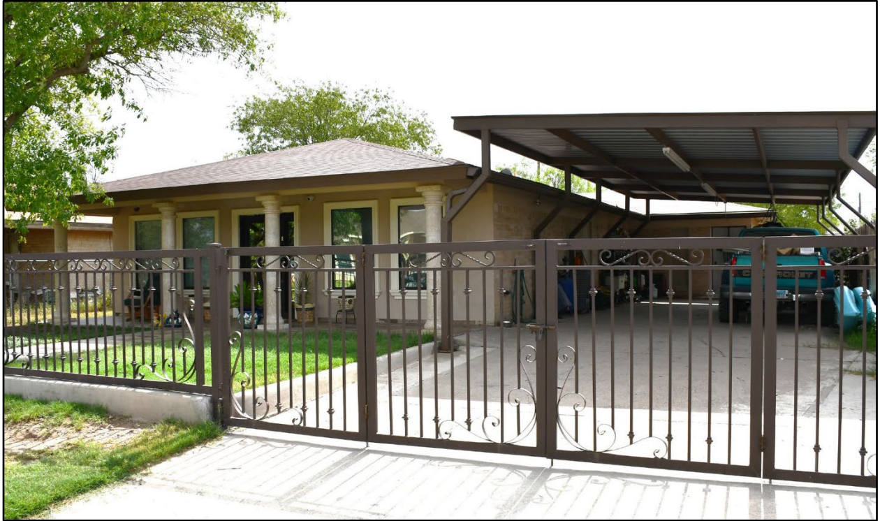
Figure 14. Oblique view of SM-12, Facing northeast towards west (front) elevation and south (side) elevations from Commissary Avenue.
