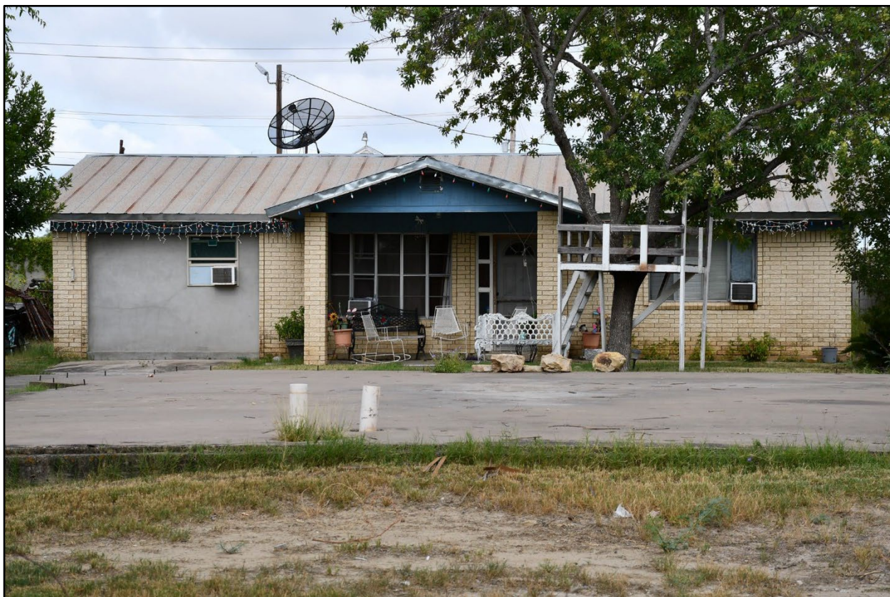
Figure 7. View of SM-05, Facing west towards east (front) elevation from Barrera Street.
