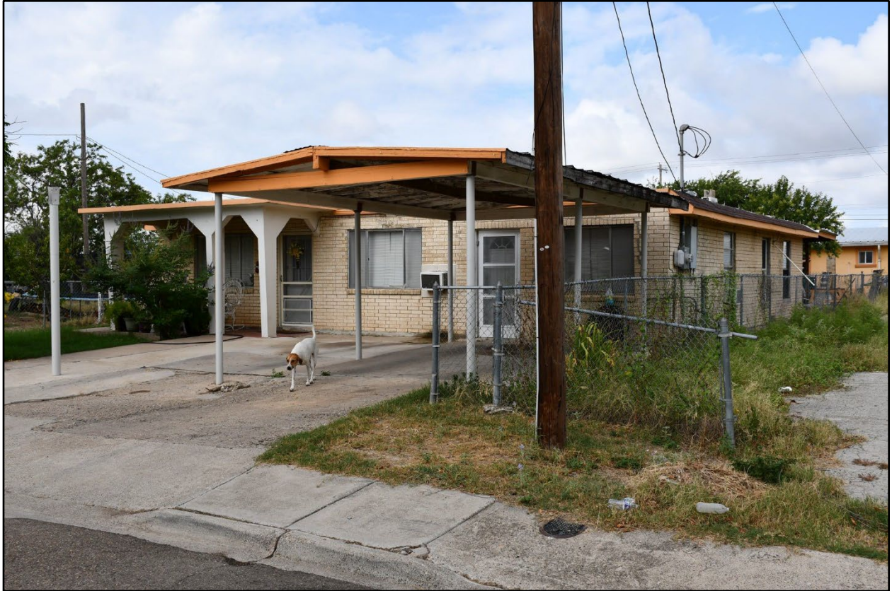
Figure 6. Oblique view of SM-04, Facing southwest towards east (front) and north (side) elevations from Barrera Street.
