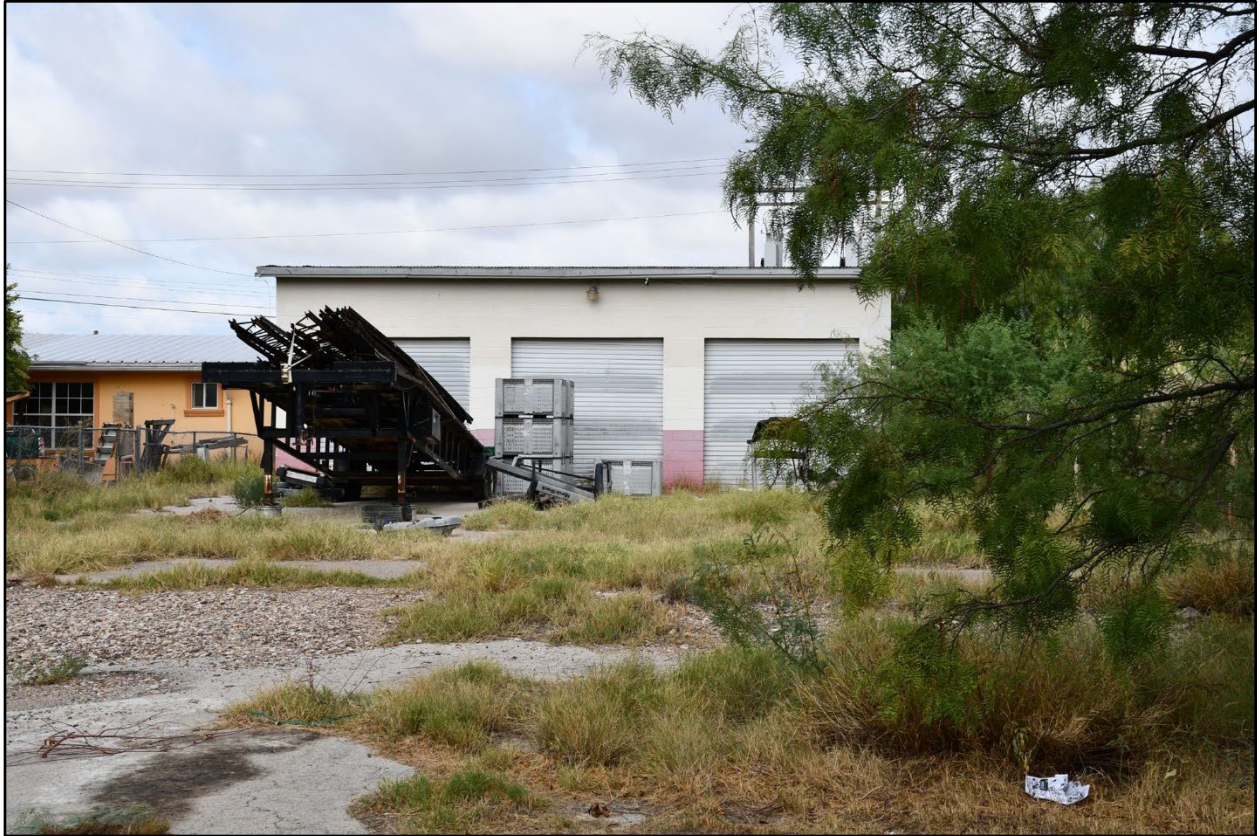
Figure 5. View of SM-03, Facing west towards east (front) elevation from Barrera Street.
