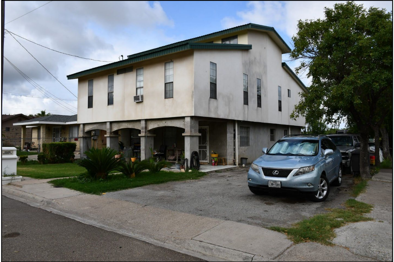
Figure 8. Oblique view of SM-06, Facing southwest towards east (front) and north (side) elevations from Barrera Street.
