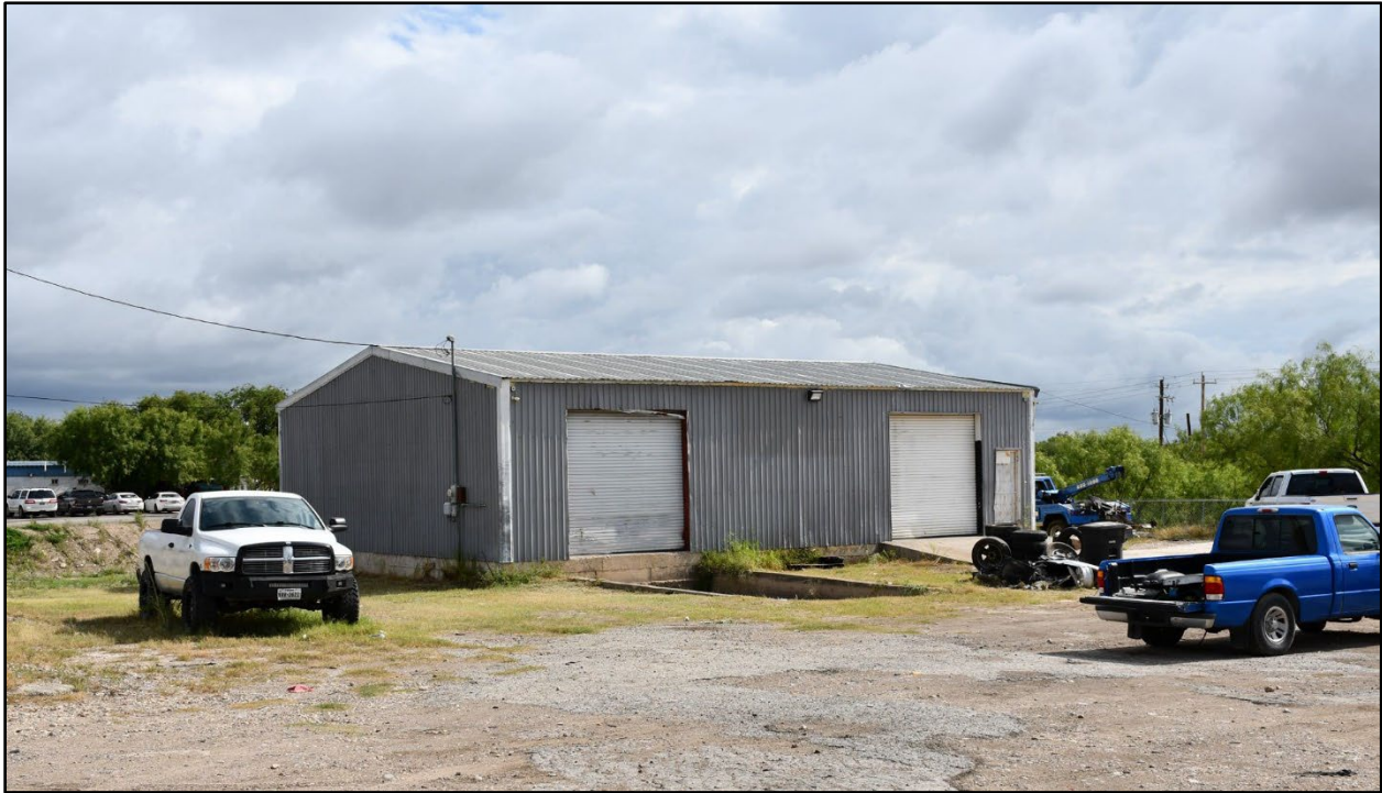
Figure 10. View of SM-08, Facing northeast towards west (side) and south (front) elevations from US 277.
