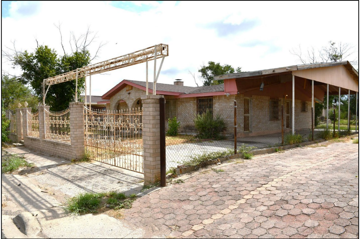
Figure 16. Oblique view of SM-14, Facing northeast towards west (front) elevation and south (side) elevations from Commissary Avenue.
