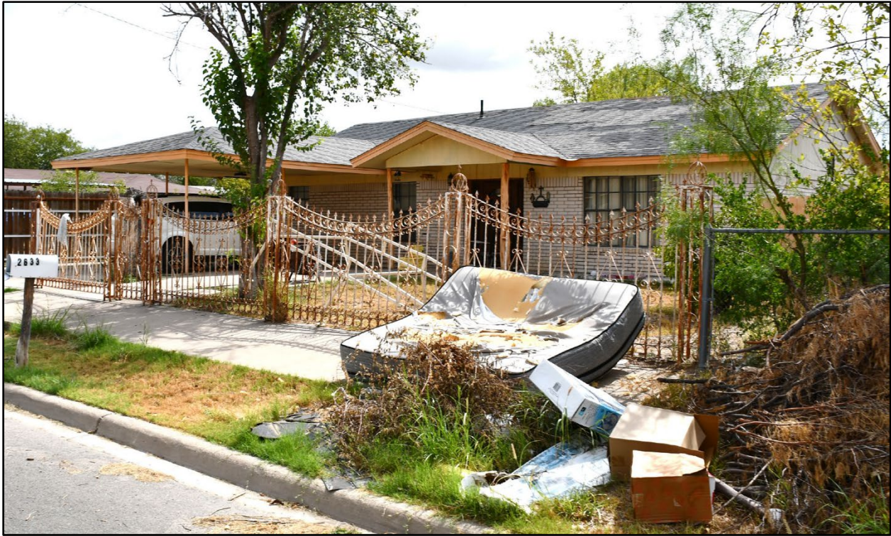
Figure 13. Oblique view of SM-11, Facing northeast towards west (front) elevation and south (side) elevations from Commissary Avenue.
