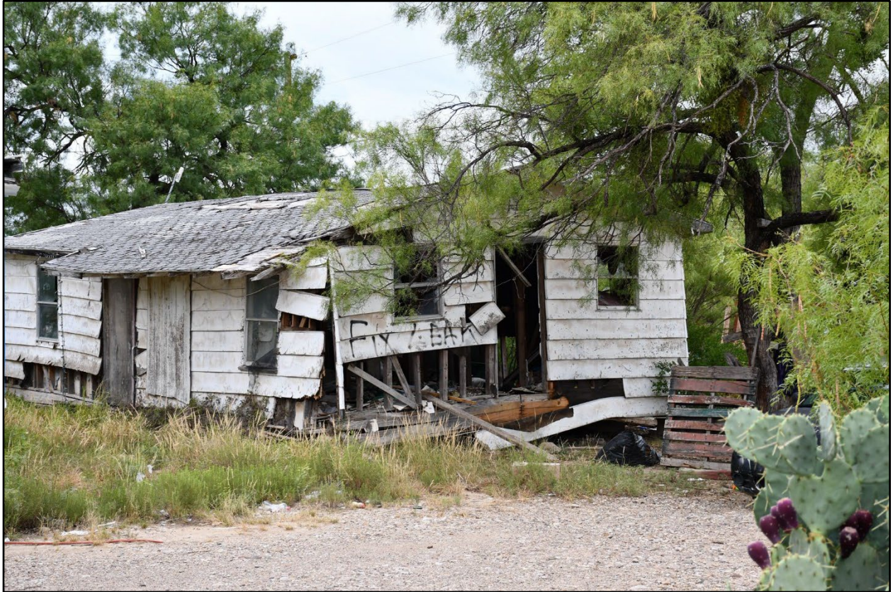
Figure 4. Oblique view of SM-02, Facing southeast towards west (side) and north (front) elevations from Dr. Gates Drive.
