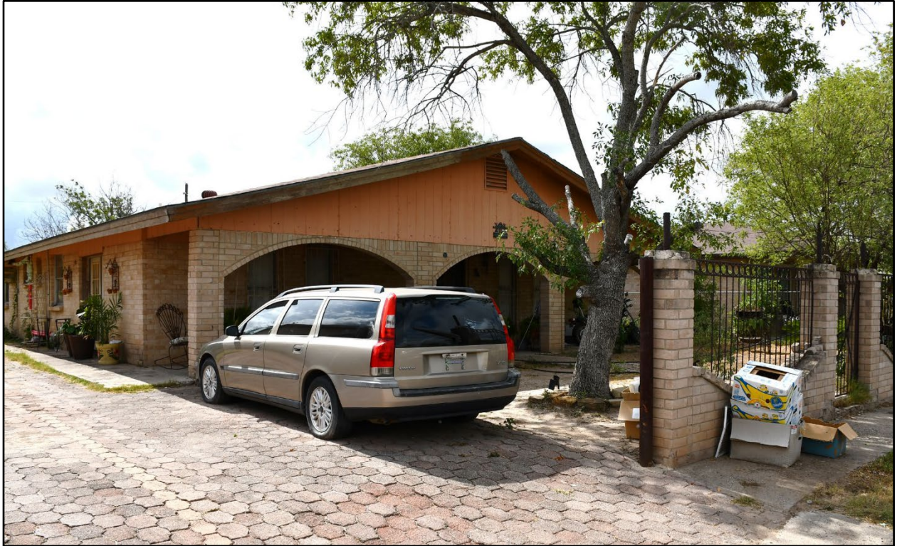
Figure 15. Oblique view of SM-13, Facing southeast towards west (front) elevation and north (side) elevations from Commissary Avenue.
