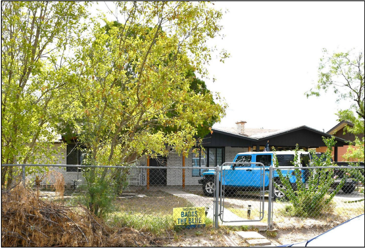
Figure 12. View of SM-10, facing east towards west (front) elevations from Commissary Avenue.
