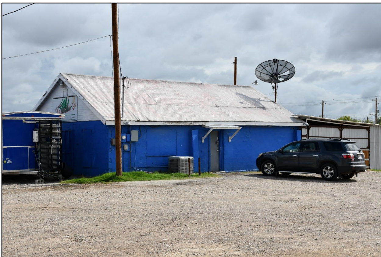
Figure 9. View of SM-07, Facing northeast towards west (front) and south (side) elevations from US 277.
